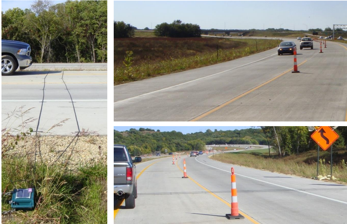
Figure 3.9. K-18 EB site setup photos
