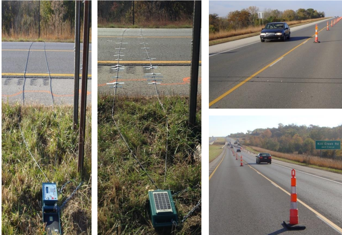
Figure 3.8. K-10 EB site setup photos
