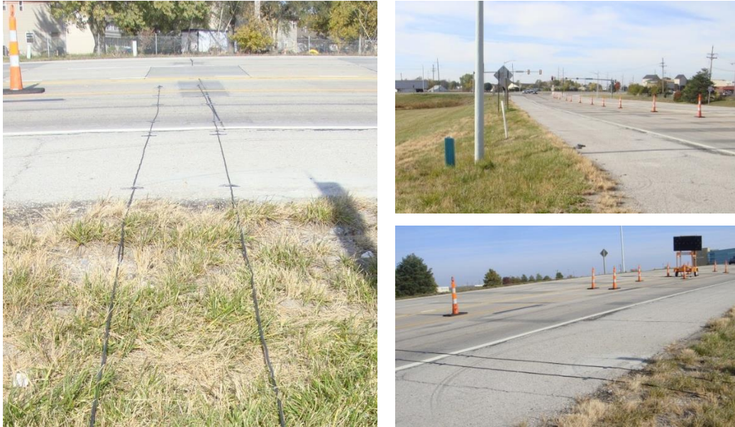
Figure 3.11. US-56 EB site setup photos
