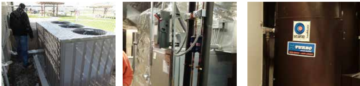
Air-cooled condensing unit
