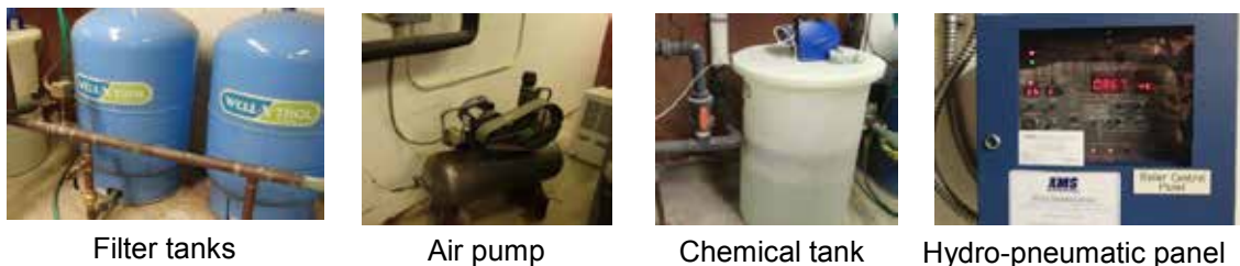
Figure 64. Water-treatment system components for Mackinaw Dells rest area.
