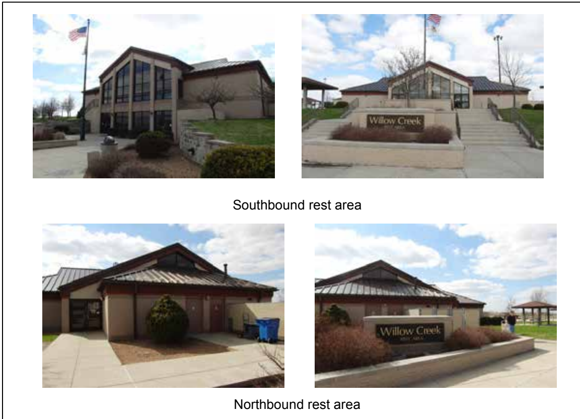
Figure 14. Willow Creek rest area.
