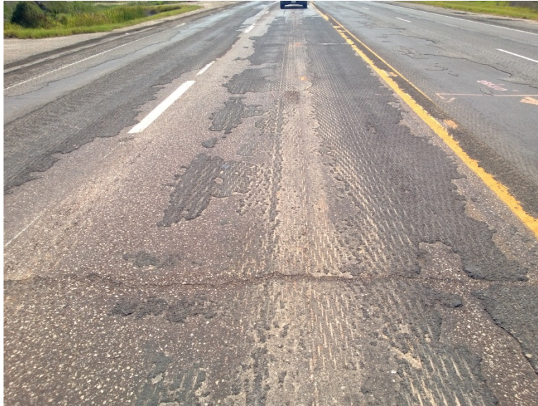
Figure 6.3. Prepared Surface.
