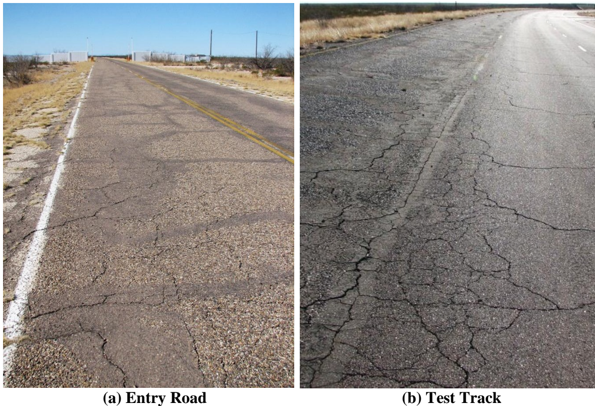
Figure 6.9. Surface Distress.
