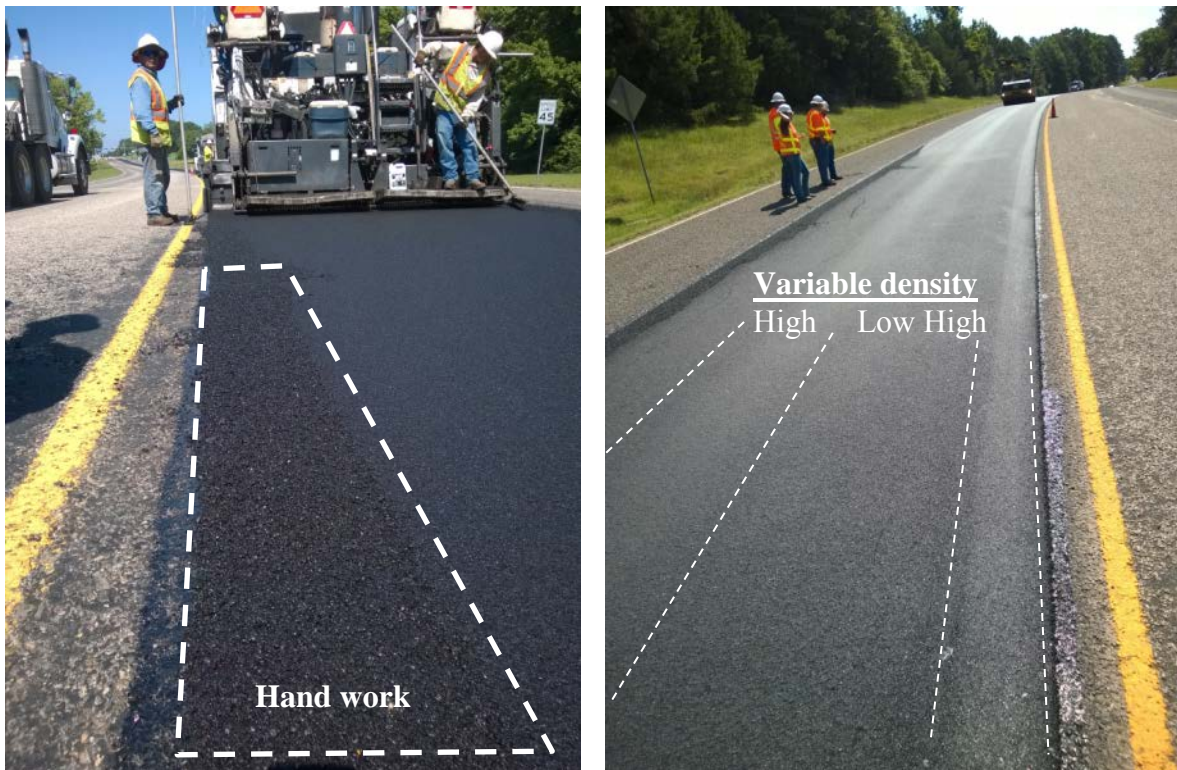
Figure G.11. Hand-Working Issue Causing Uneven Compaction.
