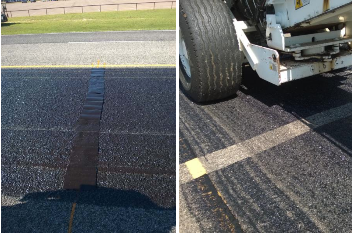
Figure G.10. Measuring Tack Application Rate.
