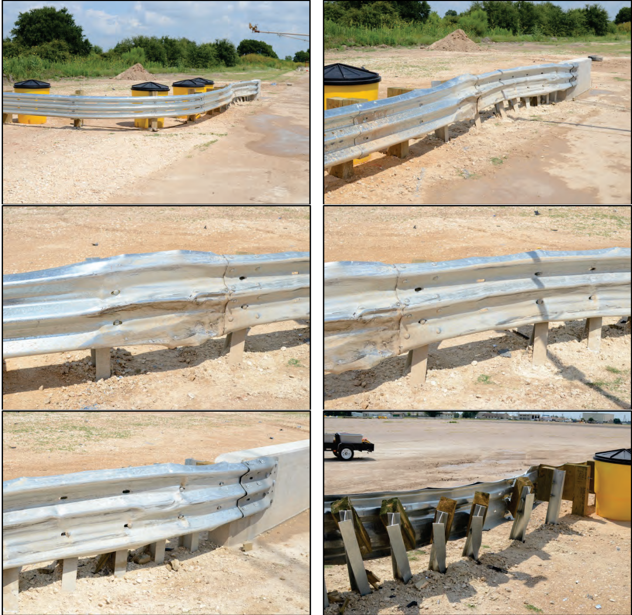
Figure 7.21. Installation after Test No. 467114-6.
