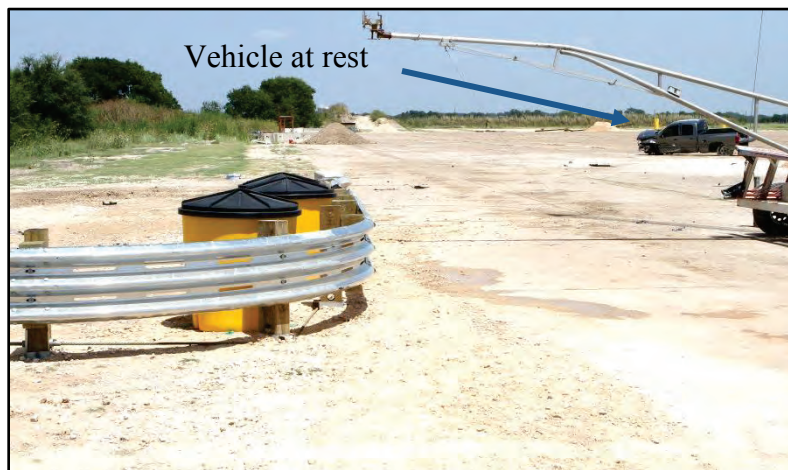
Figure 7.25. Vehicle/Installation after Test No. 467114-7.
