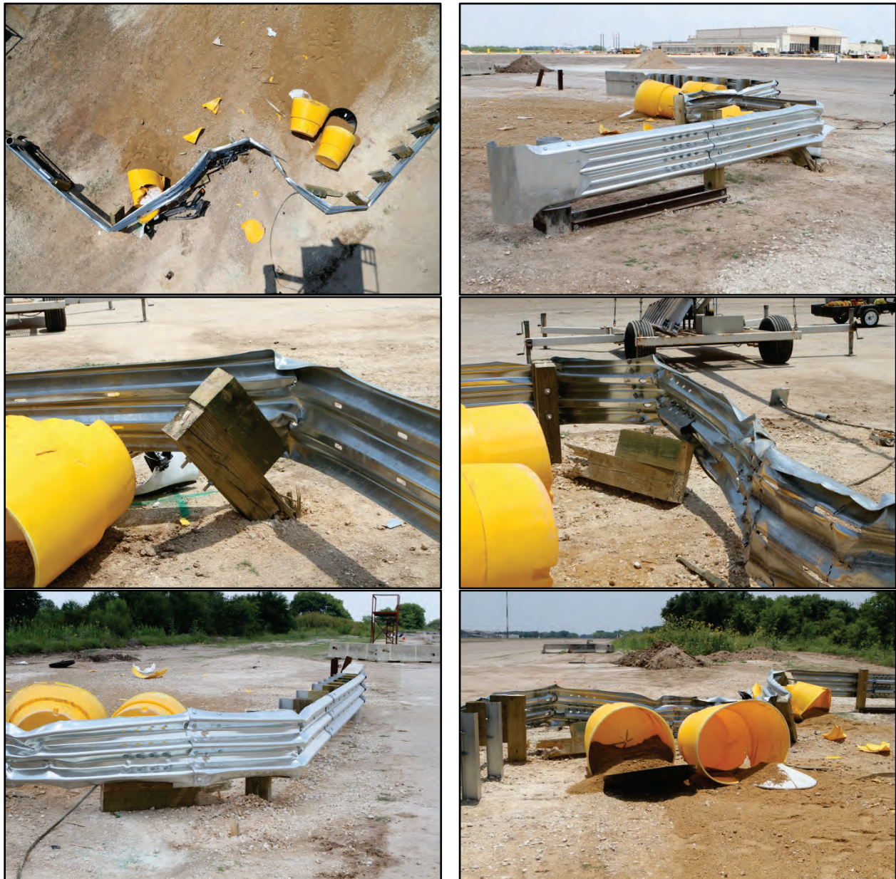
Figure 7.9. Installation after Test No. 467114-4.
