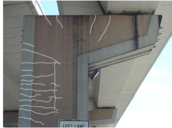
(b) Cantilever Bent
