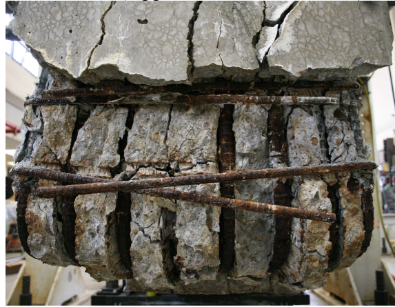
(d) Anchorage Debonding of U-Bars, and Lateral Displacement of Longitudinal Steel, in the External Beam-Column Joint
