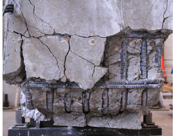
(b) Specimen 2 (Slight Damage)
