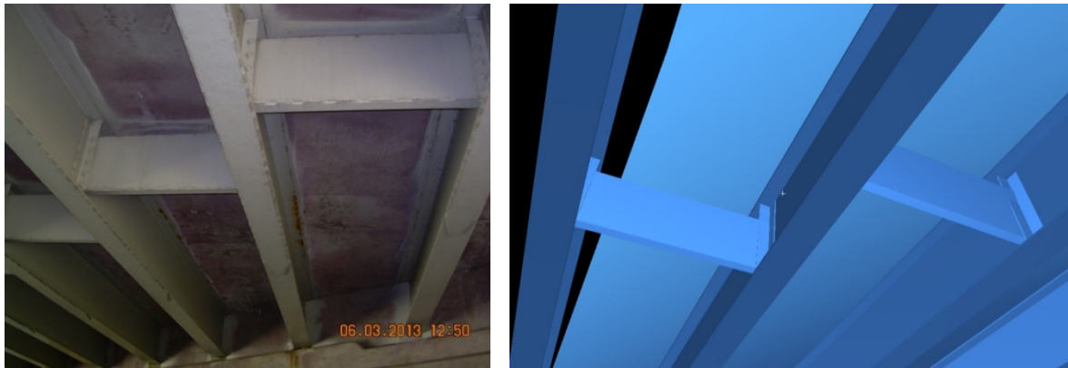
(a) Digital image (b) Modeled geometry Figure 3-6. Girders and intermediate diaphragms
