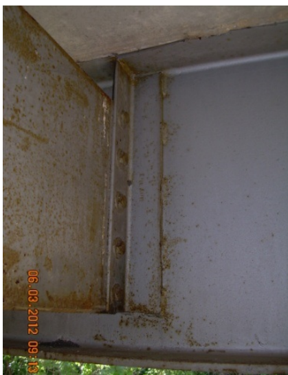
(a) Webgap at L_1 (Bridge)
