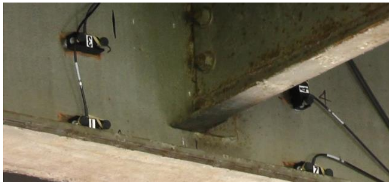
(a) AE sensors are mounted using magnet holders
