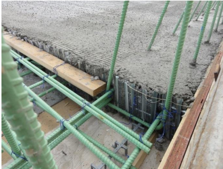
Figure 3-11 Metal shoring used in deck construction process.
