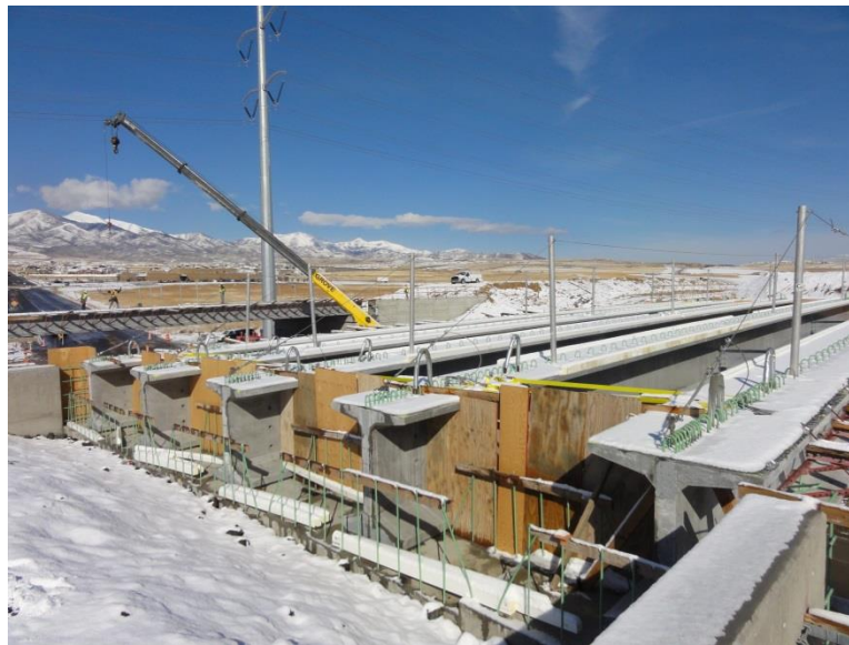
Figure 3-2 Pre-stressed, pre-cast, single-span concrete girders.
