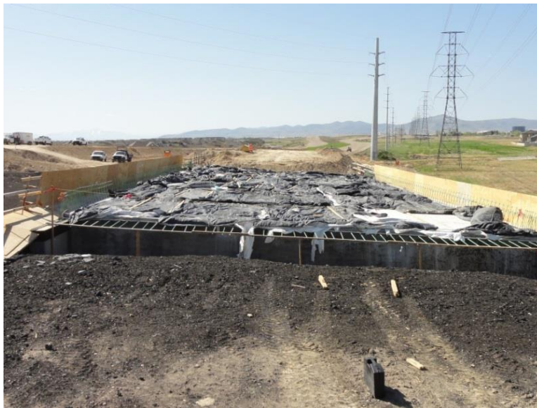
Figure 3-12 Covered bridge deck during curing.
