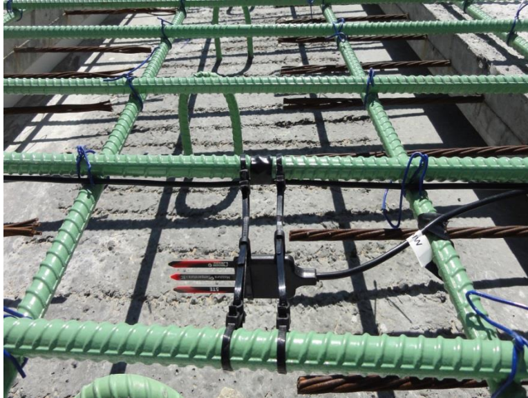
Figure 3-6 Sensor installed at level of top mat of reinforcement.
