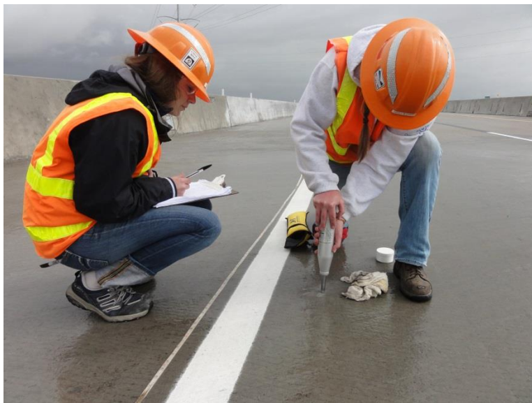
Figure 3-16 Schmidt rebound hammer testing.
