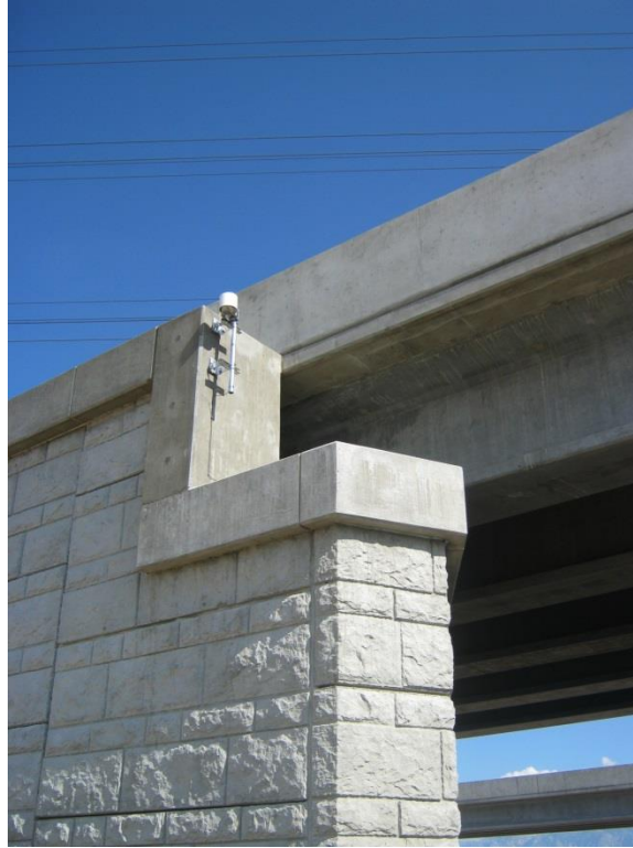
Figure 3-9 Precipitation gauge mounted on bridge.
