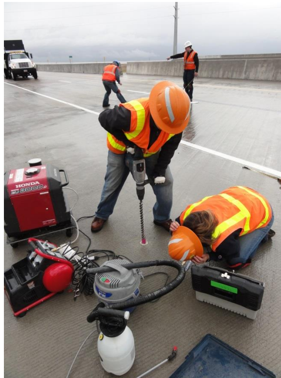
Figure 3-19 Concrete sampling for chloride concentration testing.
