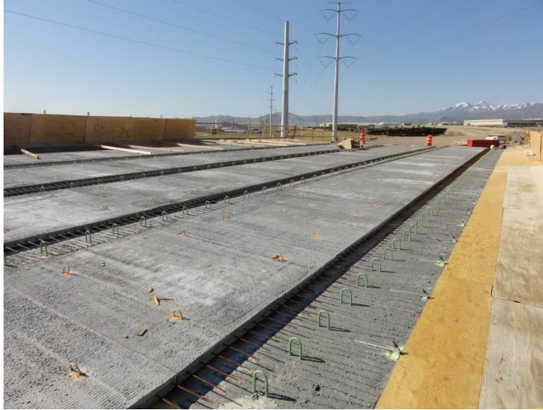
Figure 3-5 Half-deck concrete panels.
