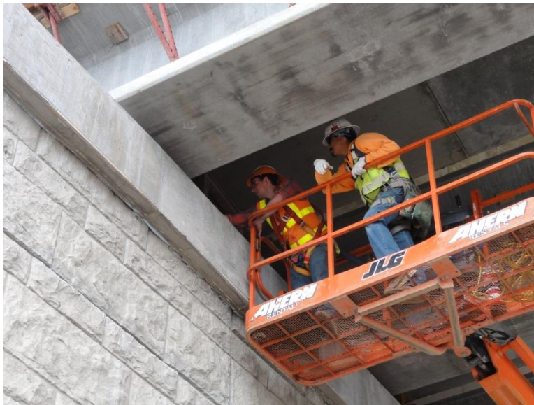
Figure 3-7 Mounting of data logger box on diaphragm wall.
