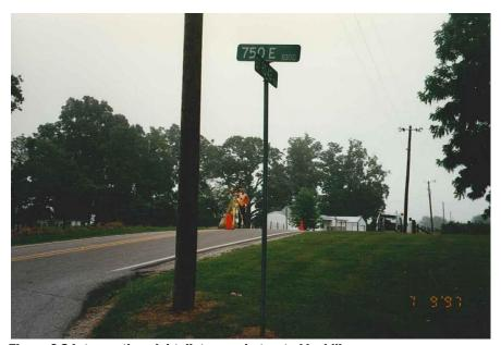
Figure 6.2 Intersection sight distance obstructed by hill.
