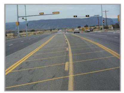
Figure 6.6 Overlapping sets of pavement markings.
