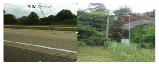
Figure 2.2 Mainline WIM detector and wireless control box
