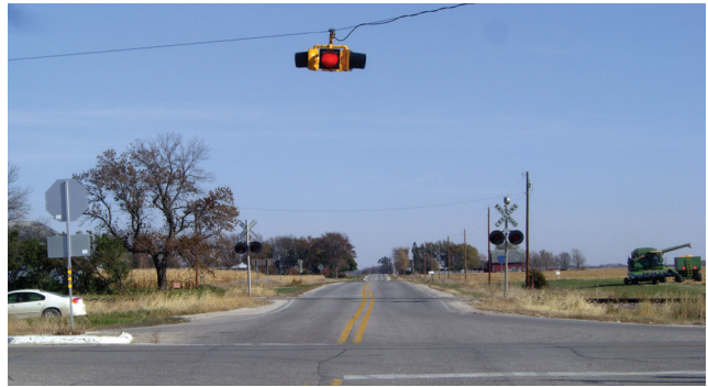
Figure 5. Overhead flashing beacon for all-way stop (Bob Sperry/Iowa Local Technical Assistance Program)
