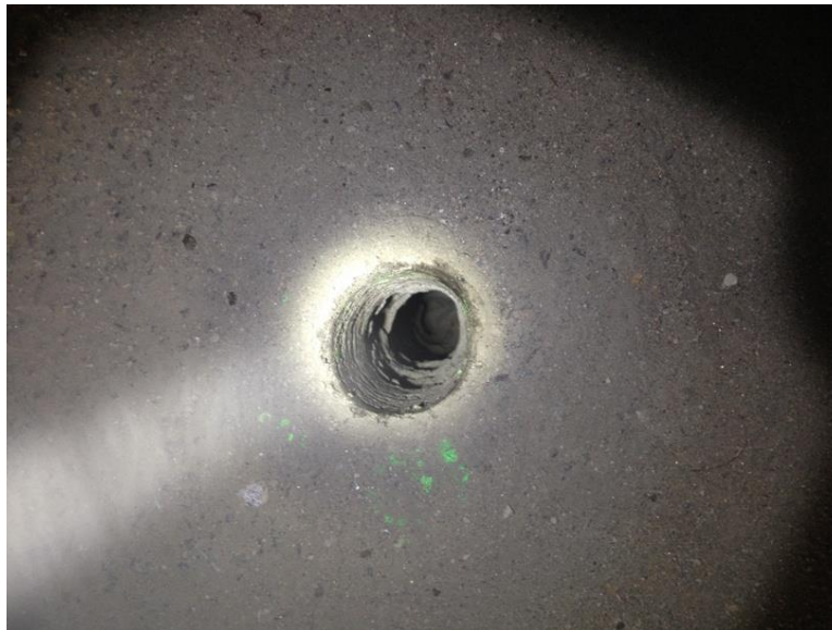
Figure 5: Drilled Injection Hole (2.5 inches x 20 feet)
