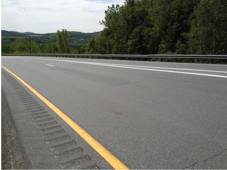
Figure 1: Deep Injection Site – Prior to Injection.
