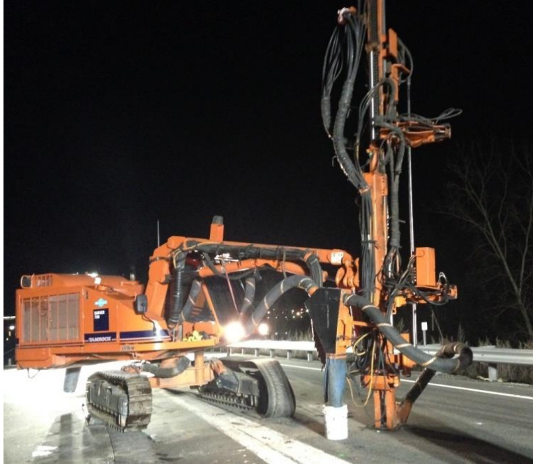
Figure 4: Tamrock 700 Drill Rig – Drilling 2.5-inch Injection Holes.
