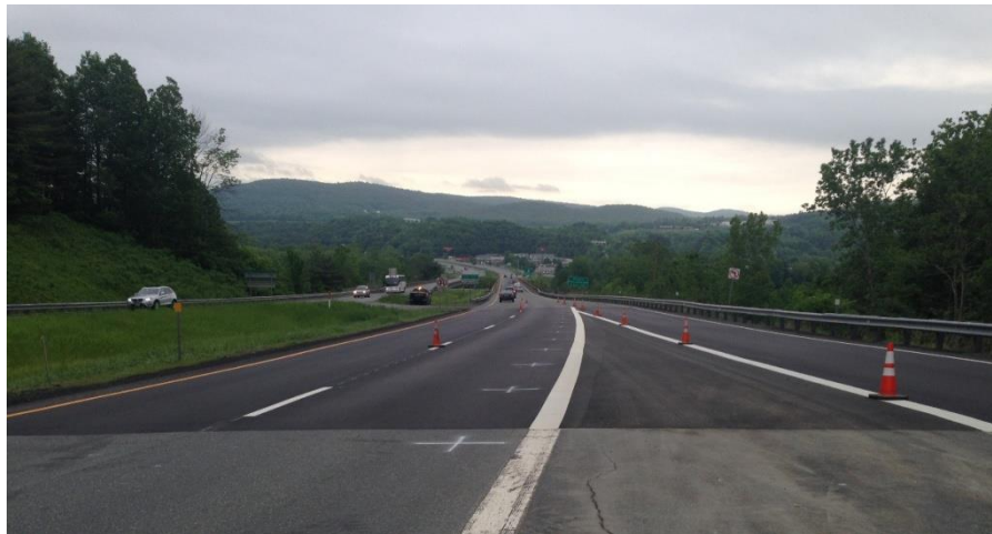
Figure 10: Deep Injection Site – Post Paving.
