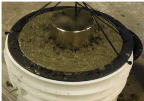
(a) Bottom Half of a Concrete Encasement
