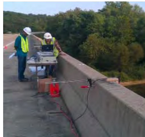
(b) Over Bridge Deck
