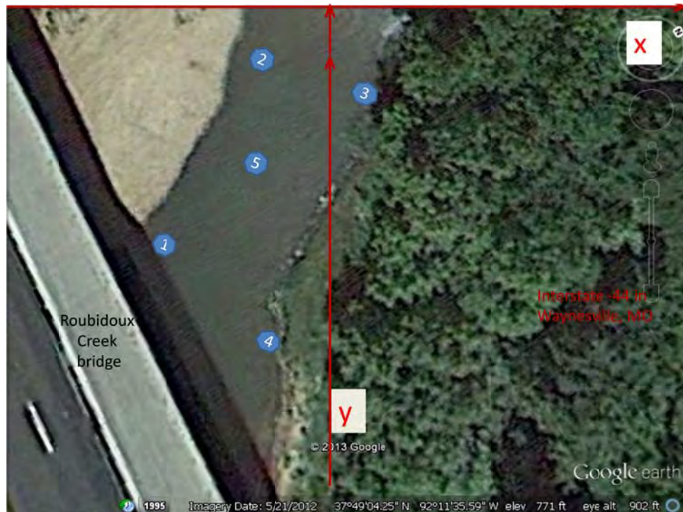
Figure 6.13 Experimental Site for Field Test 3 at I-44 Roubidoux Creek Bridge
