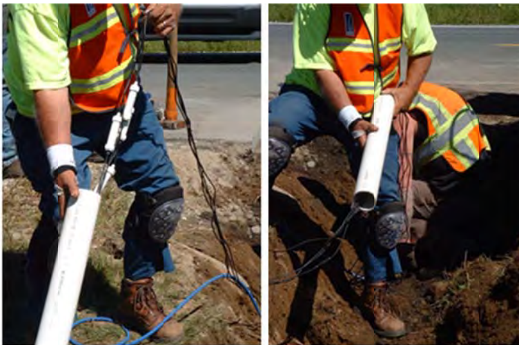
Figure 9. Backfilling trench in roadway at Warren Flats site
