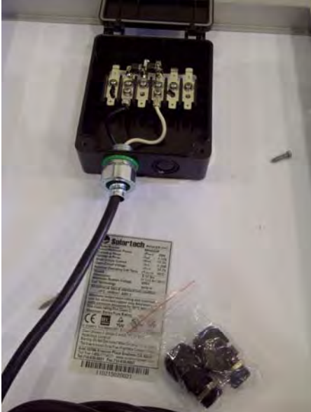
Solar Panel Junction Box with Liquid tight conduit Connection (seal top of connector with sealing puddy)
