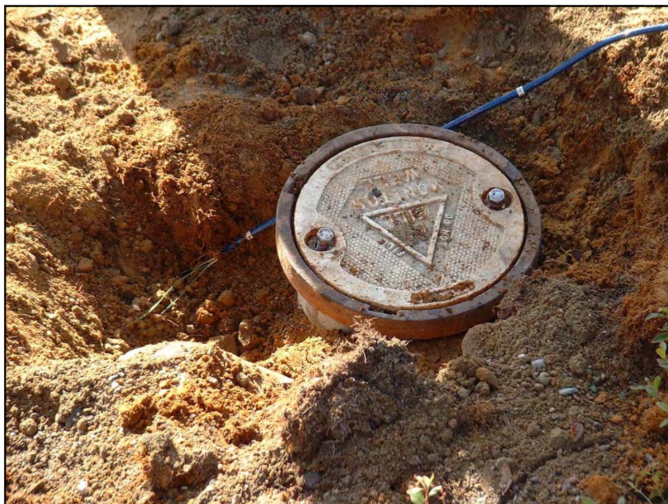
Fig E-6. Water Well Completed Installation at Ground Level
