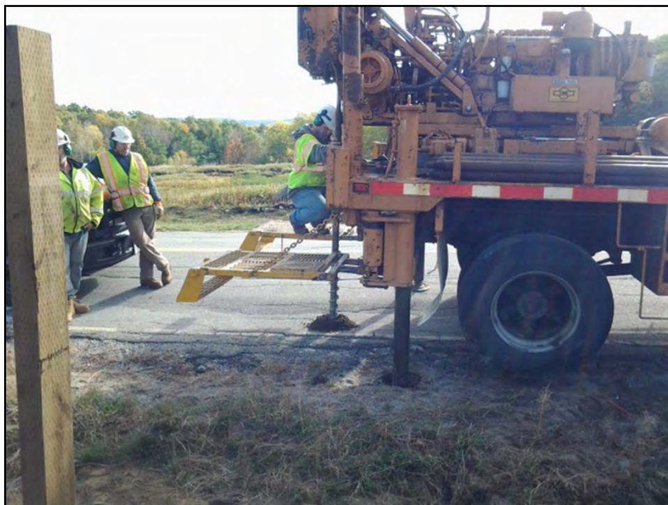
Fig E-14. Exploratory Boring for Ledge
