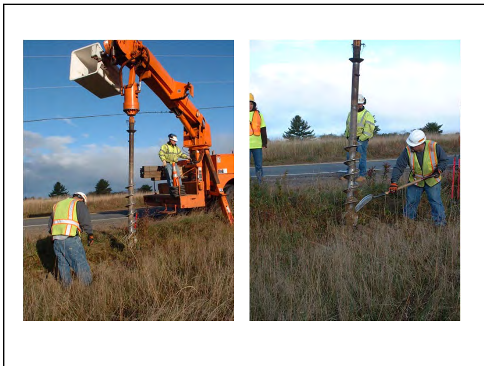
Fig F-1. Drilling Hole for Readout Box Post
