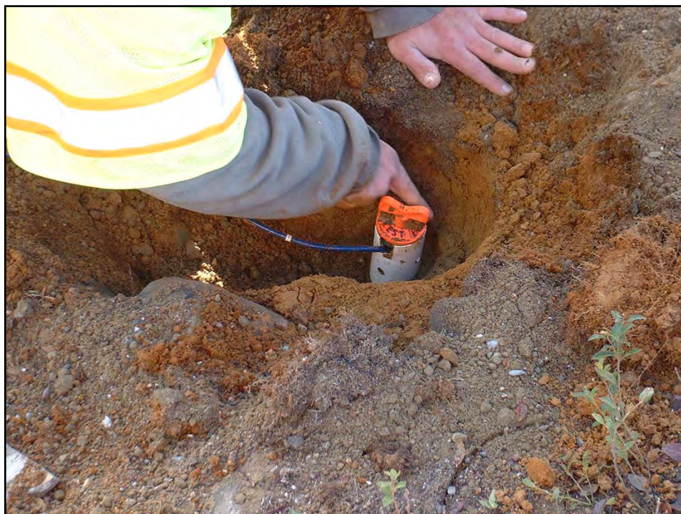
Fig E-4. Pressure Transducer Cable Coming Out of Top of Casing
