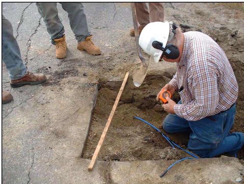
Fig E-23. Setting Top Surface Temperature Sensors
