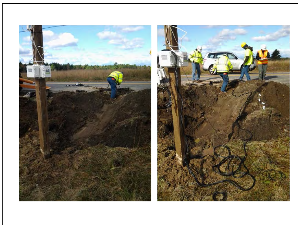
Fig F-12. Running Instrumentation Wires from Road to Readout Post
