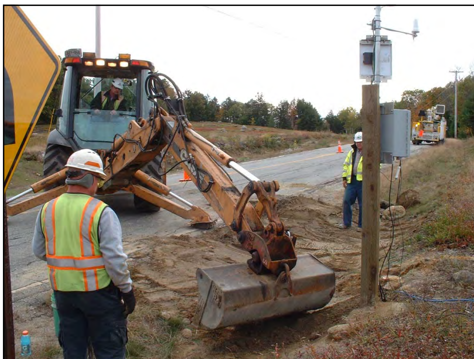
Fig E-28. Finishing Ditch Line
