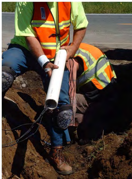
Fig D-21. Protective Casing for Modules
