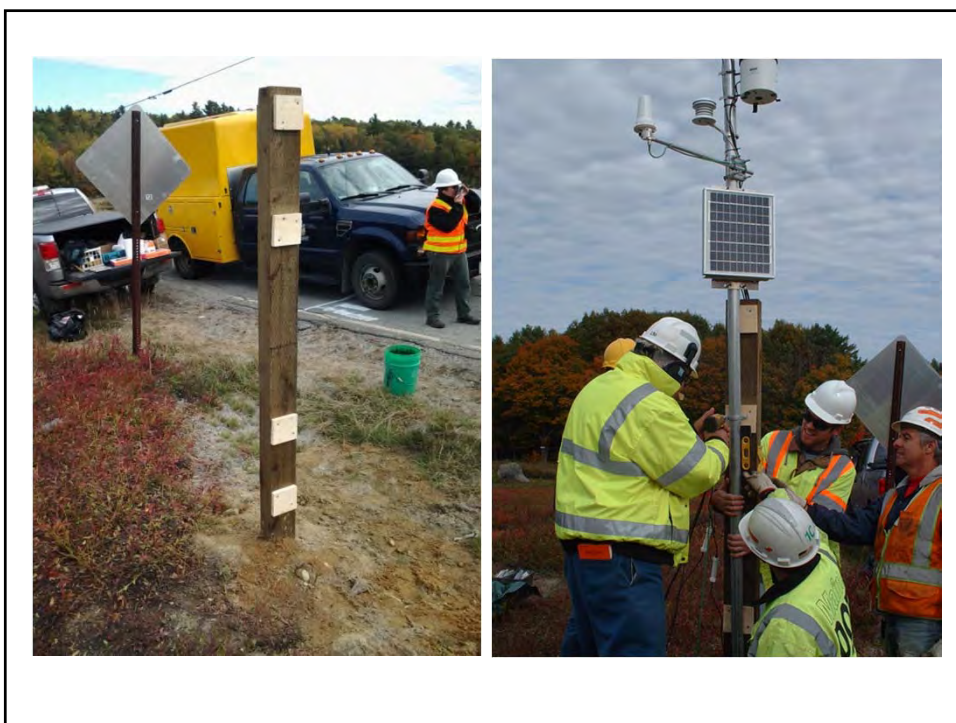
Fig E-12. Set off Blocks for Mounting
