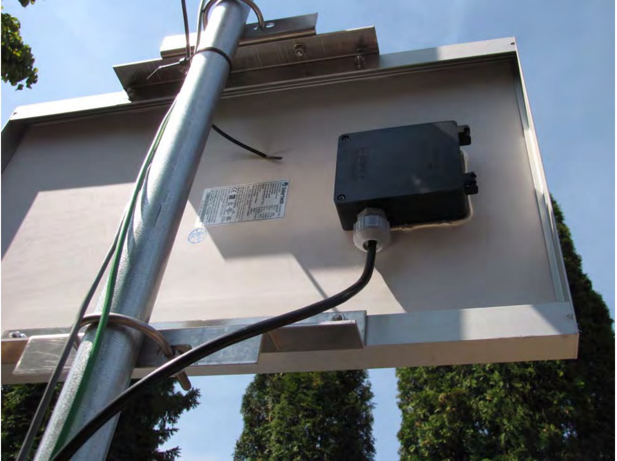
Solar Panel with Pole Mount / Cable Gland and Cable to Satellite Enclosure
