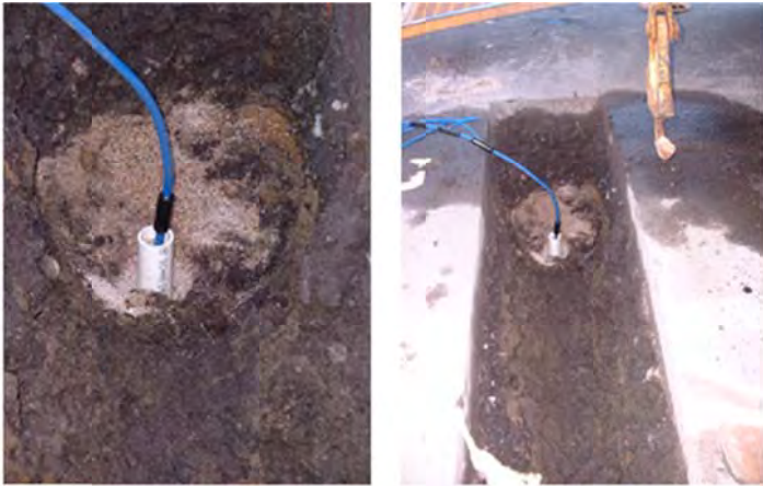
Figure 6. Installation of thermistor string at Warren Flats site
