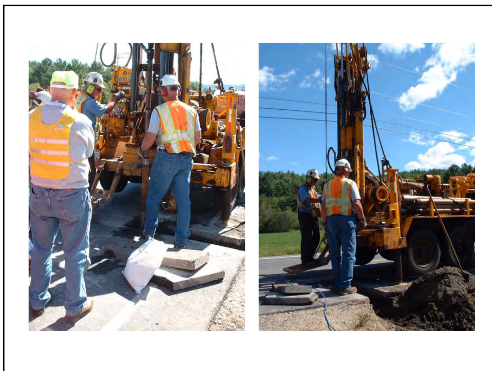
Fig D-10. Drilling Temperature Sensor Holes Fig D-11. Temperature Sensor Installation
