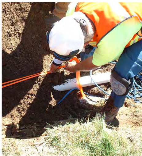
Flagging placed in trench prior to final backfilling
