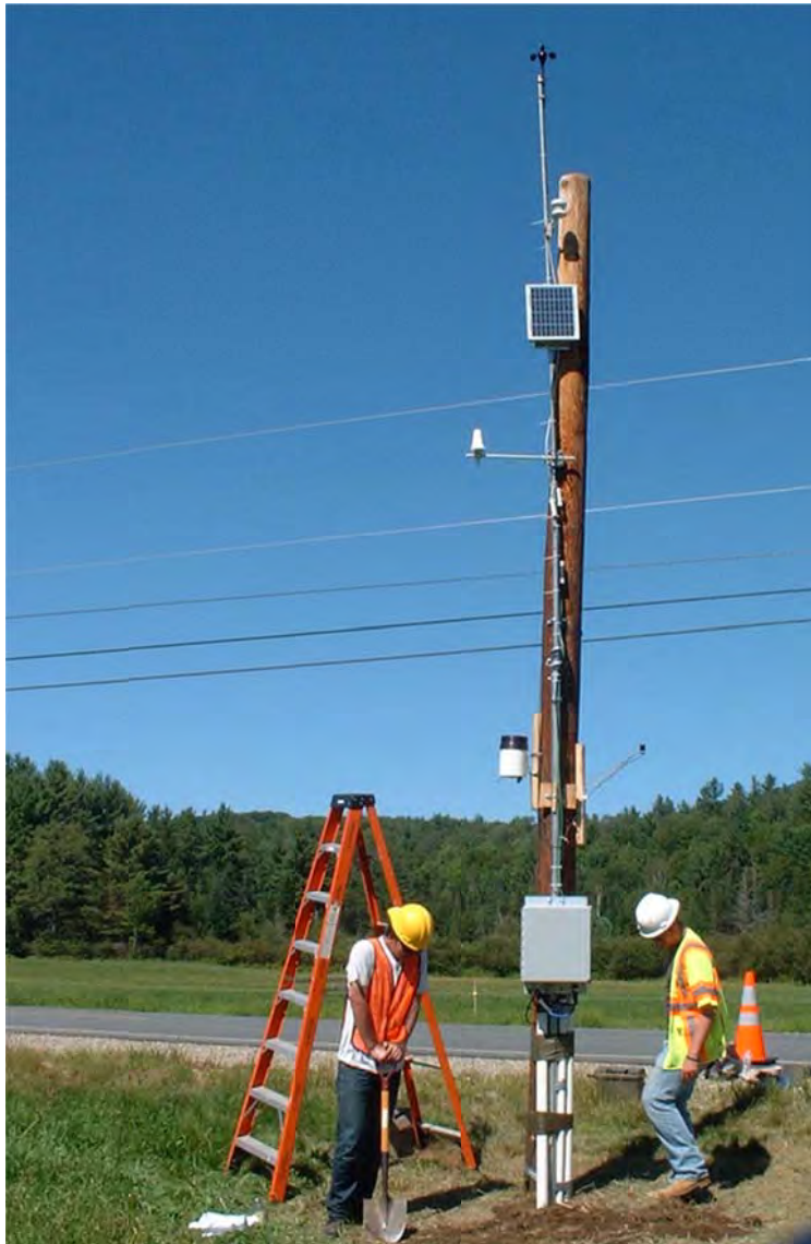
Figure 4. Warren Flats, NH Site
