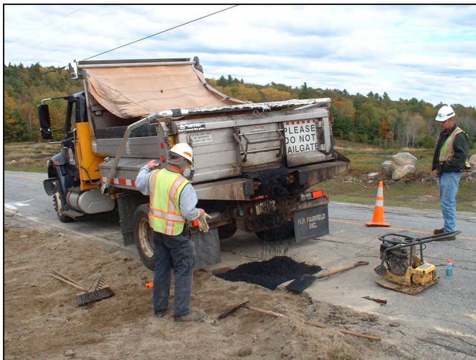
Fig E-28. Hot Asphalt Pavement Patching Trench
