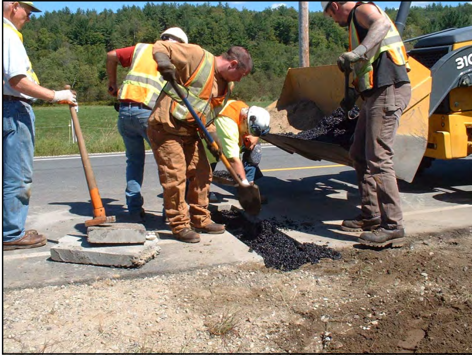
Fig D-24. Placing Temporary Cold Patch Pavement
