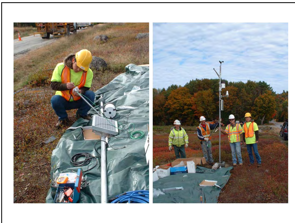
Fig E-10. Mounting Instrumentation to Pole Fig E-11. Checking Locations on Pole
