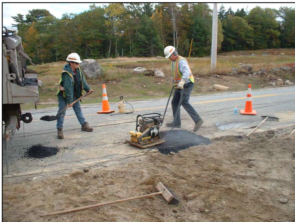
Fig E-29. Compacting Hotmix
