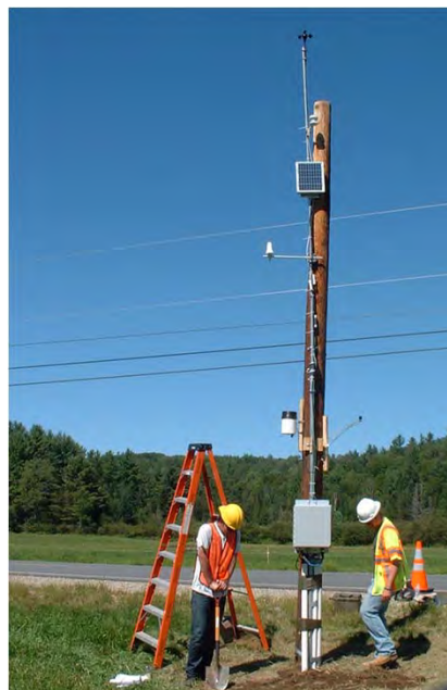
Fig D-8. Looking North
