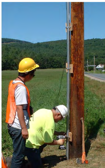
Fig D-5. Looking West
