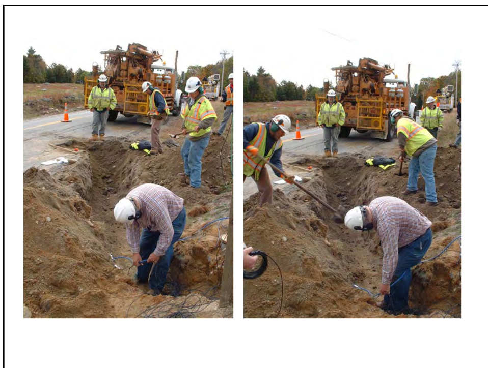
Fig E-25. Running Instrumentation Cables to Readout Box
