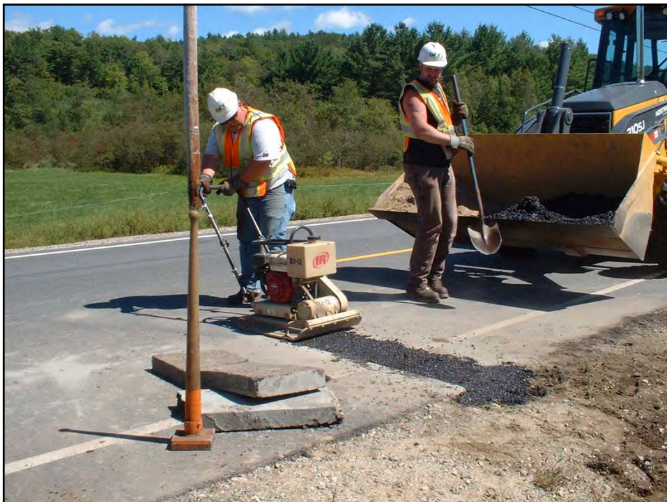
Fig D-25. Compacting Cold Patch
