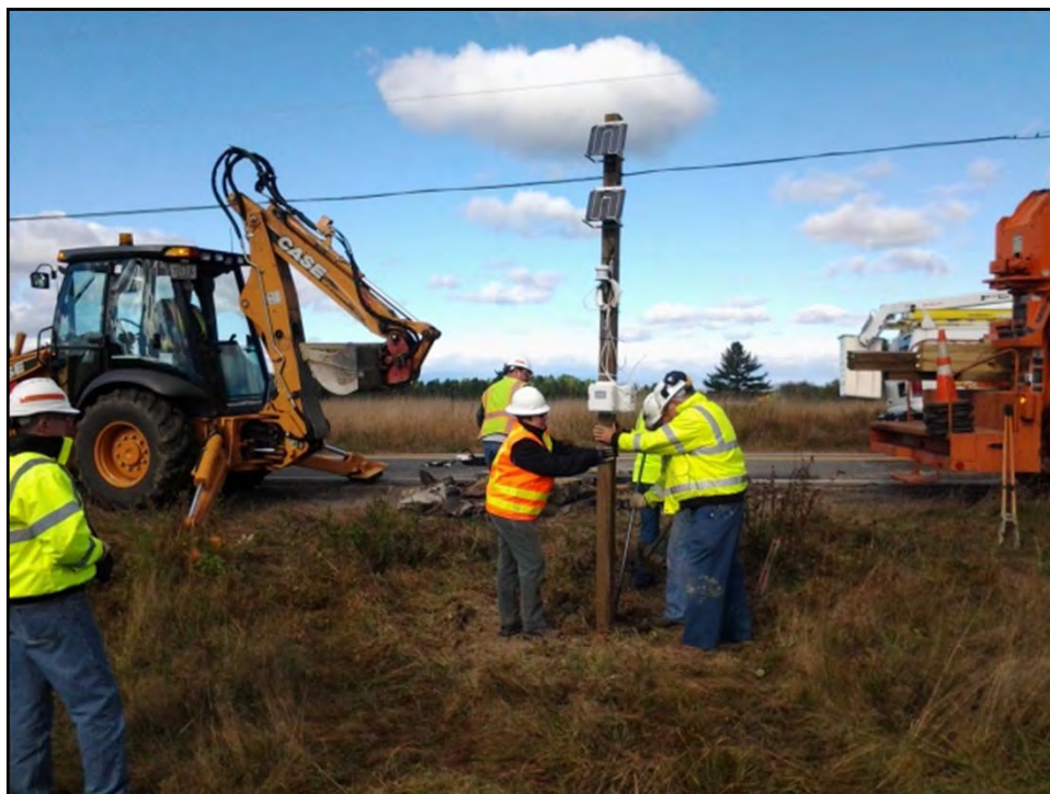
Fig F-10. Checking Vertical Alignment of Post
