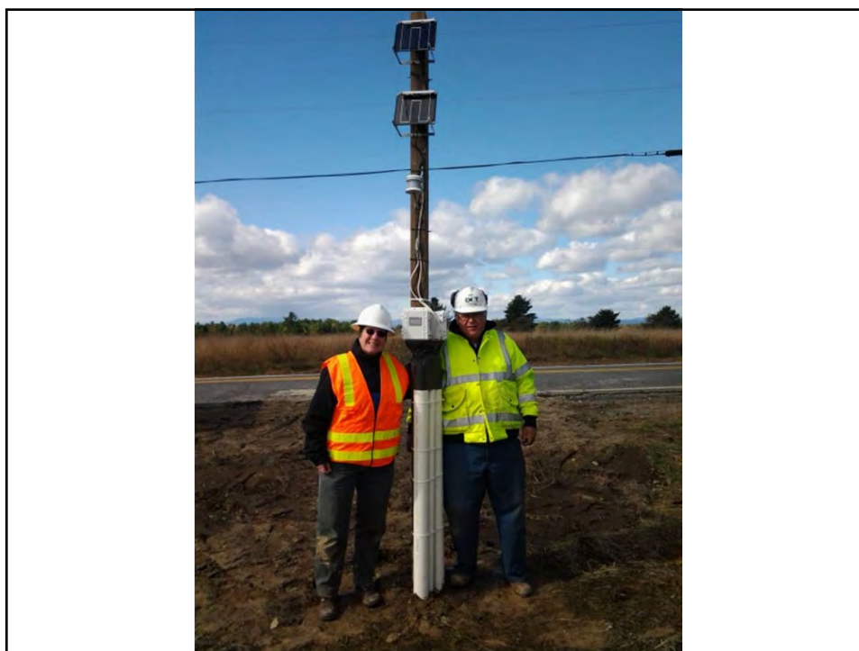
Fig F-16. Heather Miller and Bob Eaton at Completed Installation
