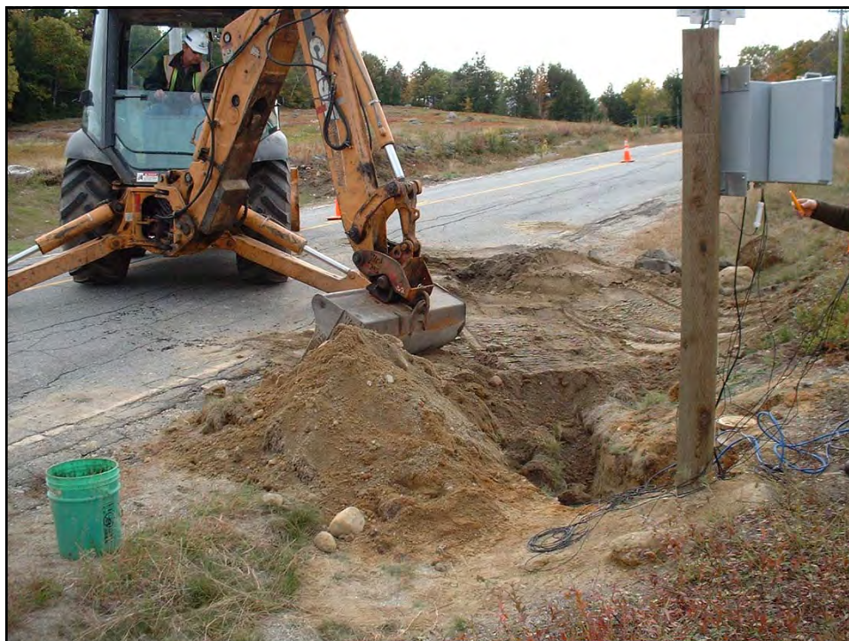
Fig E-27. Backfilling Trench
