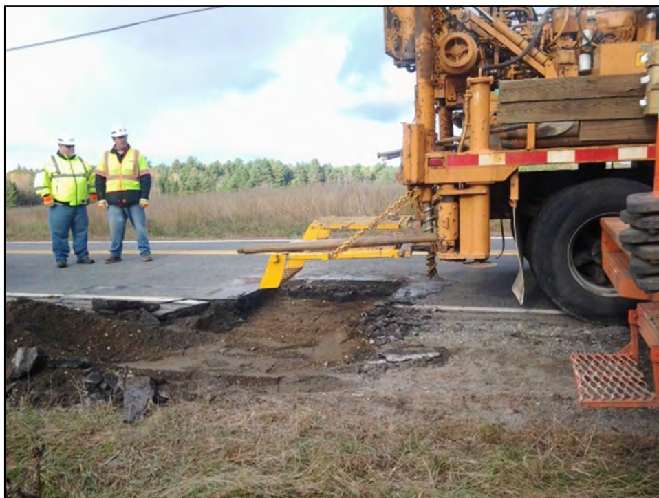
Fig F-3. Drilling Hole for Soil Samples
