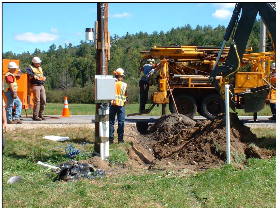
Fig D-9. Drilling Temperature Sensors Hole (Water Well Standpipe on Right)
