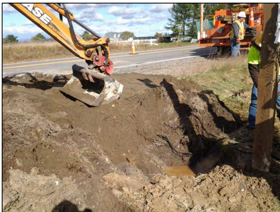
Fig F-13. Backfilling Trench
