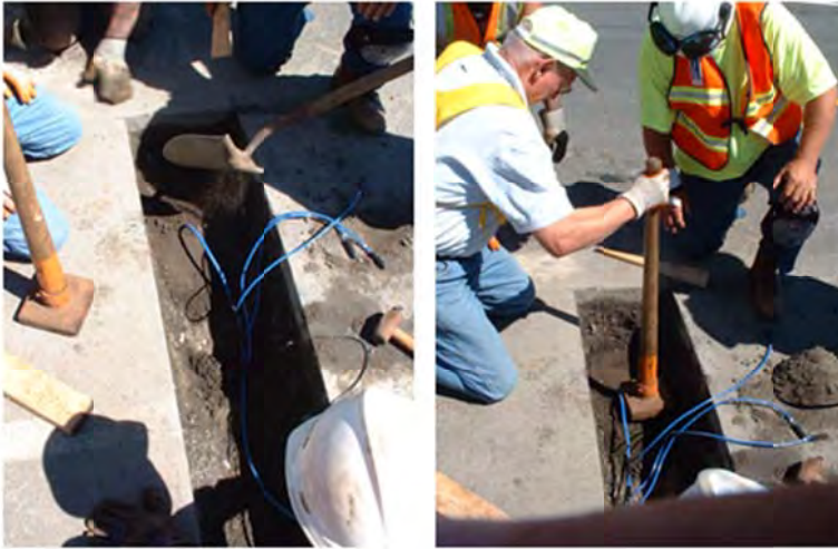
Figure 8. Backfilling trench in roadway at Warren Flats site
