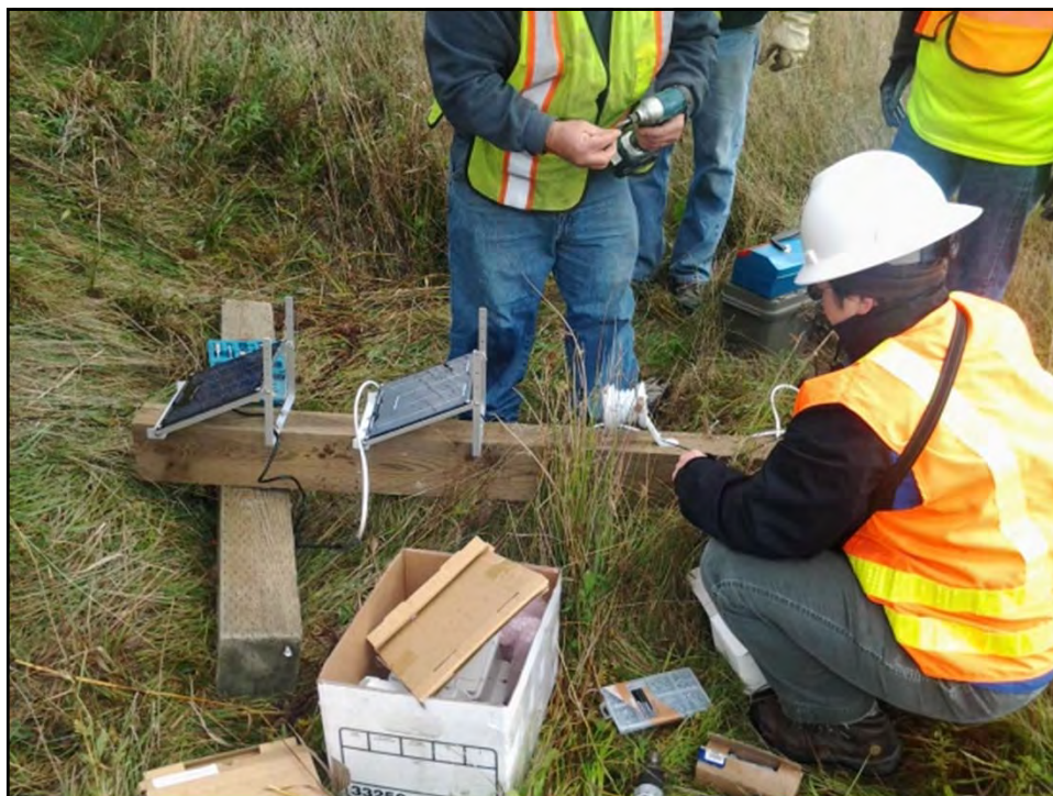
Fig F-8. Mounting Solar Panels to Wooden Post
