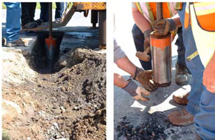
Figure 7. Coring old AC layer at Warren Flats site
