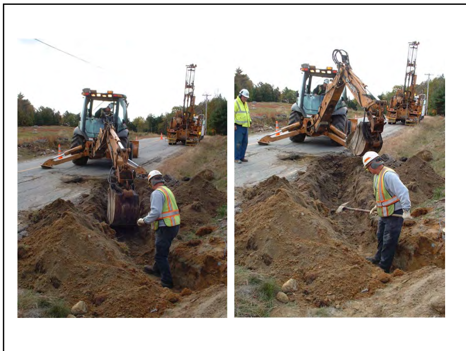
Fig E-18. Trenching for Subsurface Instrumentation Wires
