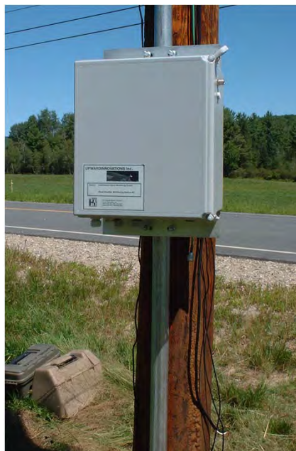
Fig D-7. Looking West
