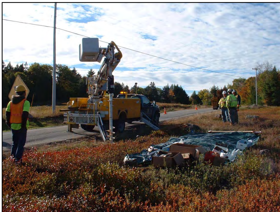
Fig E-7. Drilling Instrumentation Readout Post Borehole
