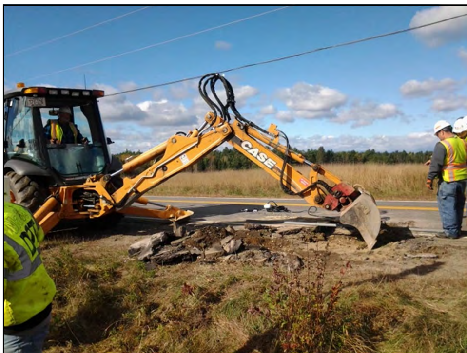
Fig F-11. Digging Trench from Road to Post
