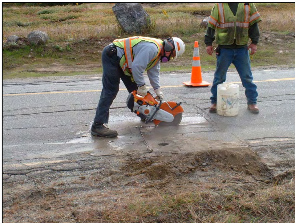
Fig E-16. Saw Cutting Pavement
