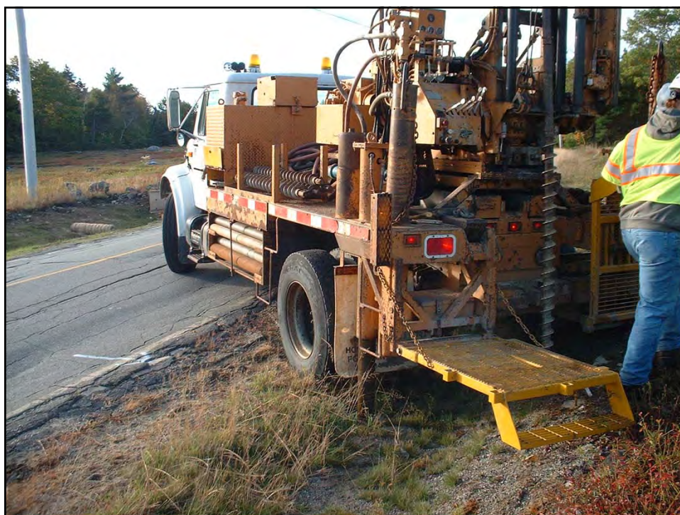
Fig E-2. Drilling Water Well
