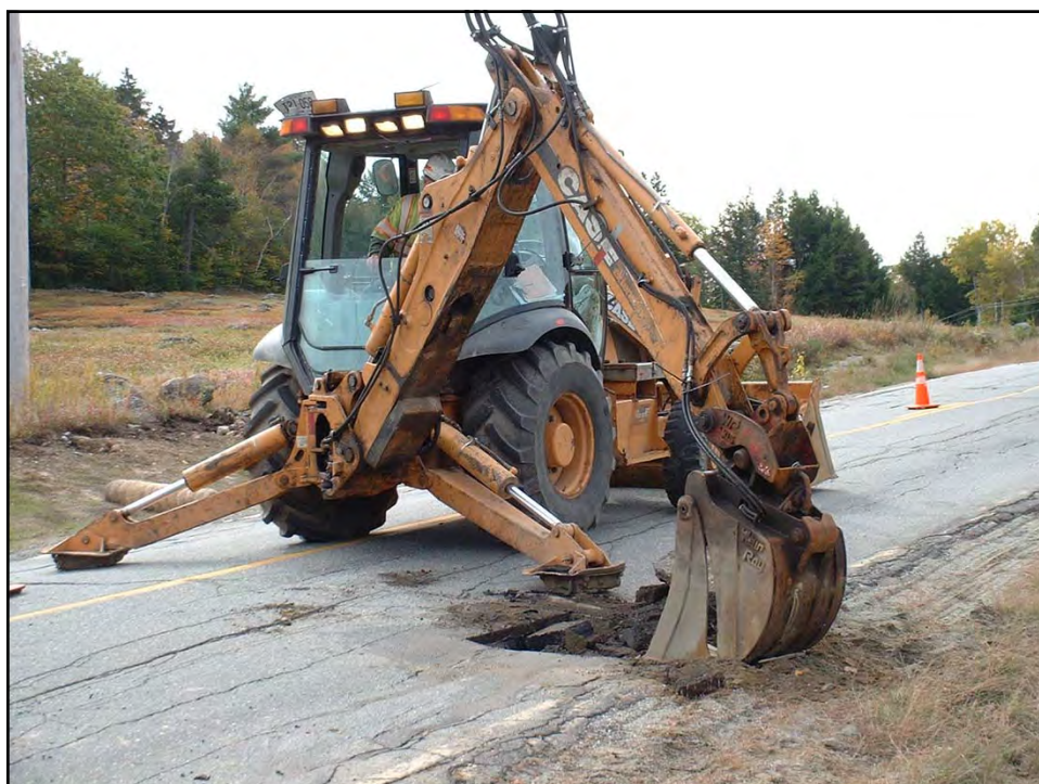
Fig E-17. Removing Pavement for Trench
