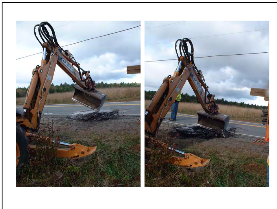
Fig F-2. Removing Pavement from Road Trench for Instrumentation Installation
