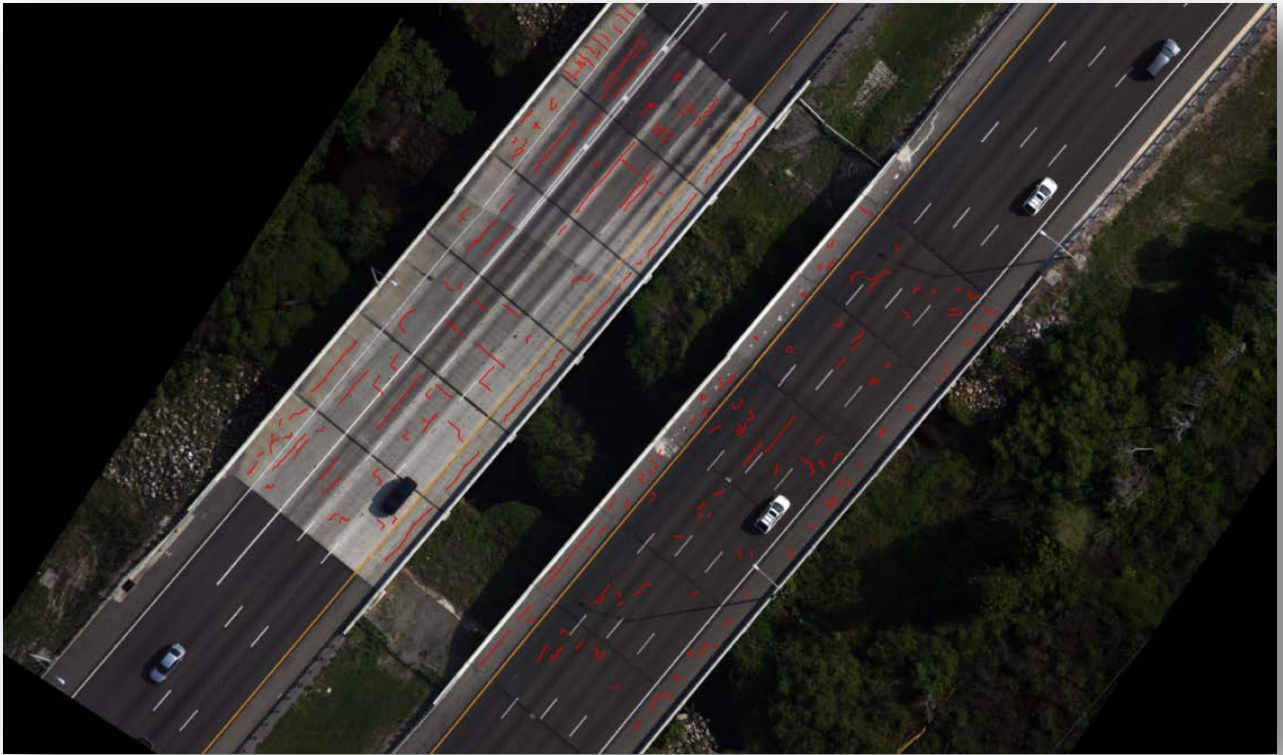
Figure C.3.9: Bridge NO. 920098 Crack Image
