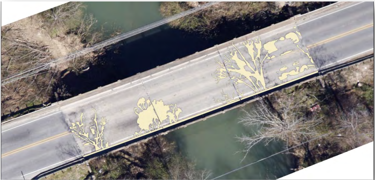
Figure C.1.2: Bridge NO. 003267 Obstruction Image
