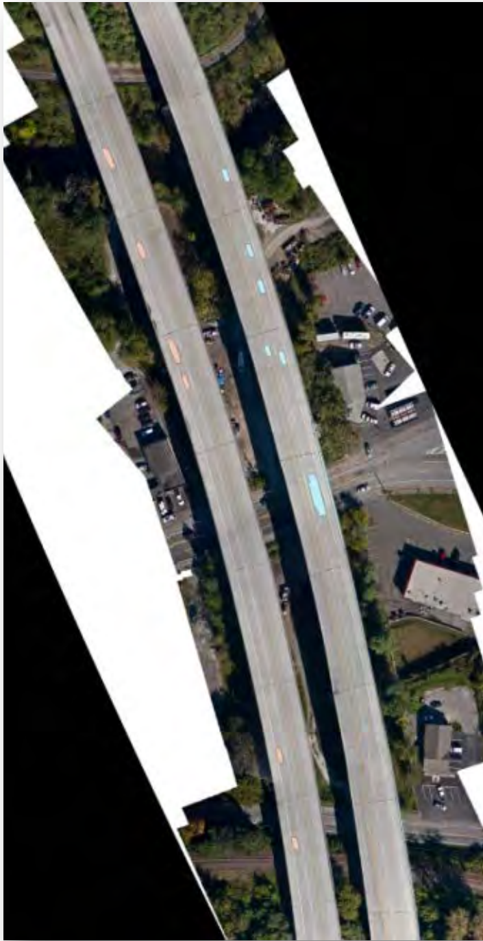
Figure C.8.38: Bridge NO. 1052842 Obstruction Image
