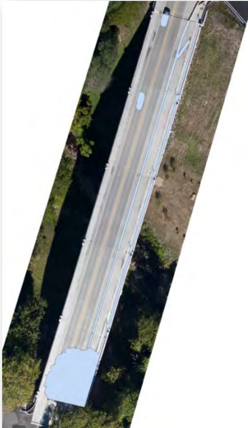
Figure C.8.8: Bridge NO. 1007140 Obstruction Image
