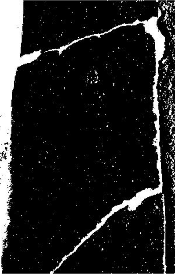
Filtered Image of total damages
