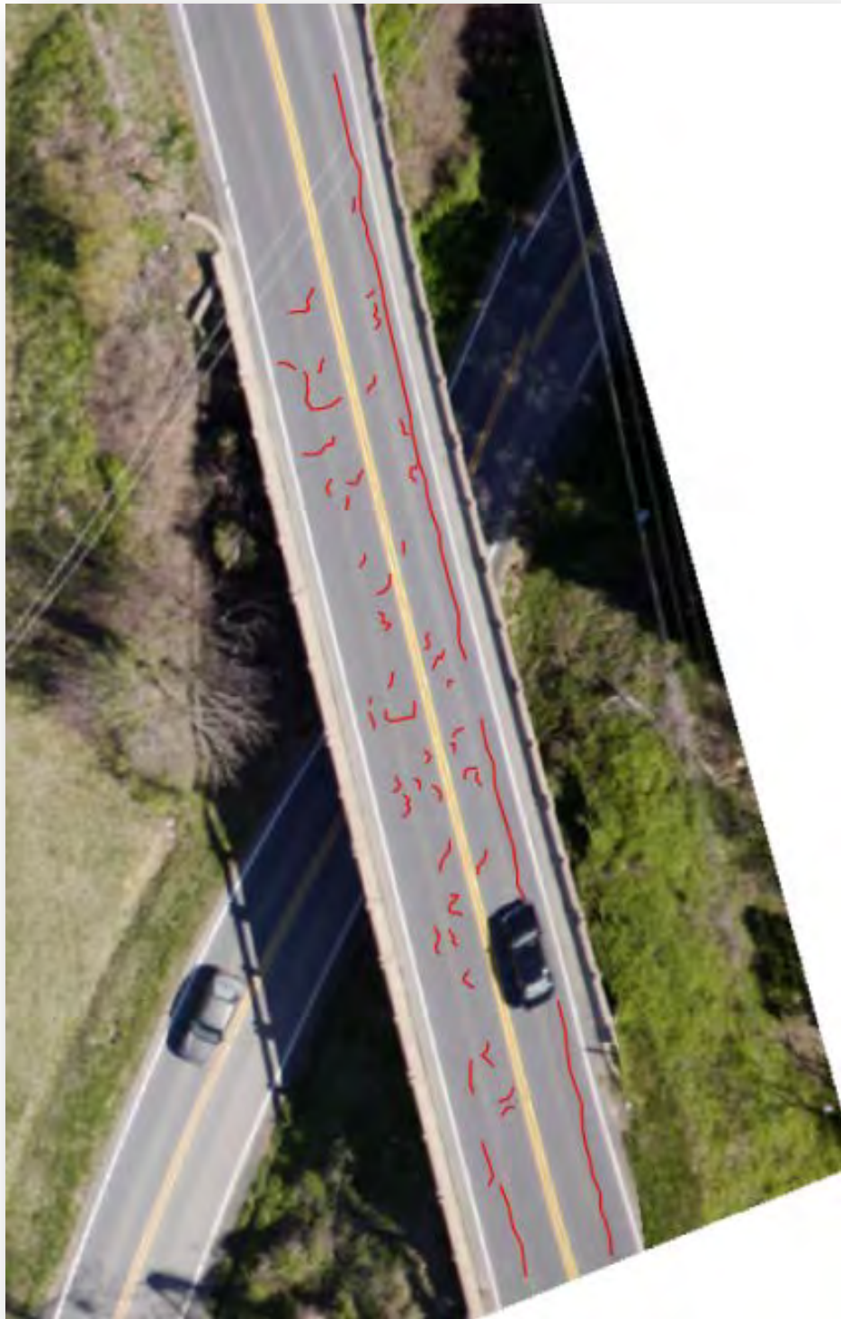
Figure C.5.27: Bridge NO. US21 St. 21 Crack Image
