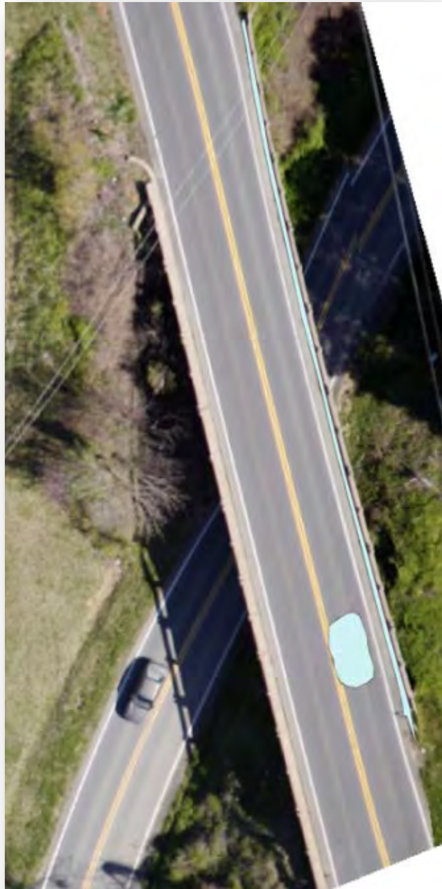
Figure C.5.26: Bridge NO. US21 St. 21 Obstruction Image
