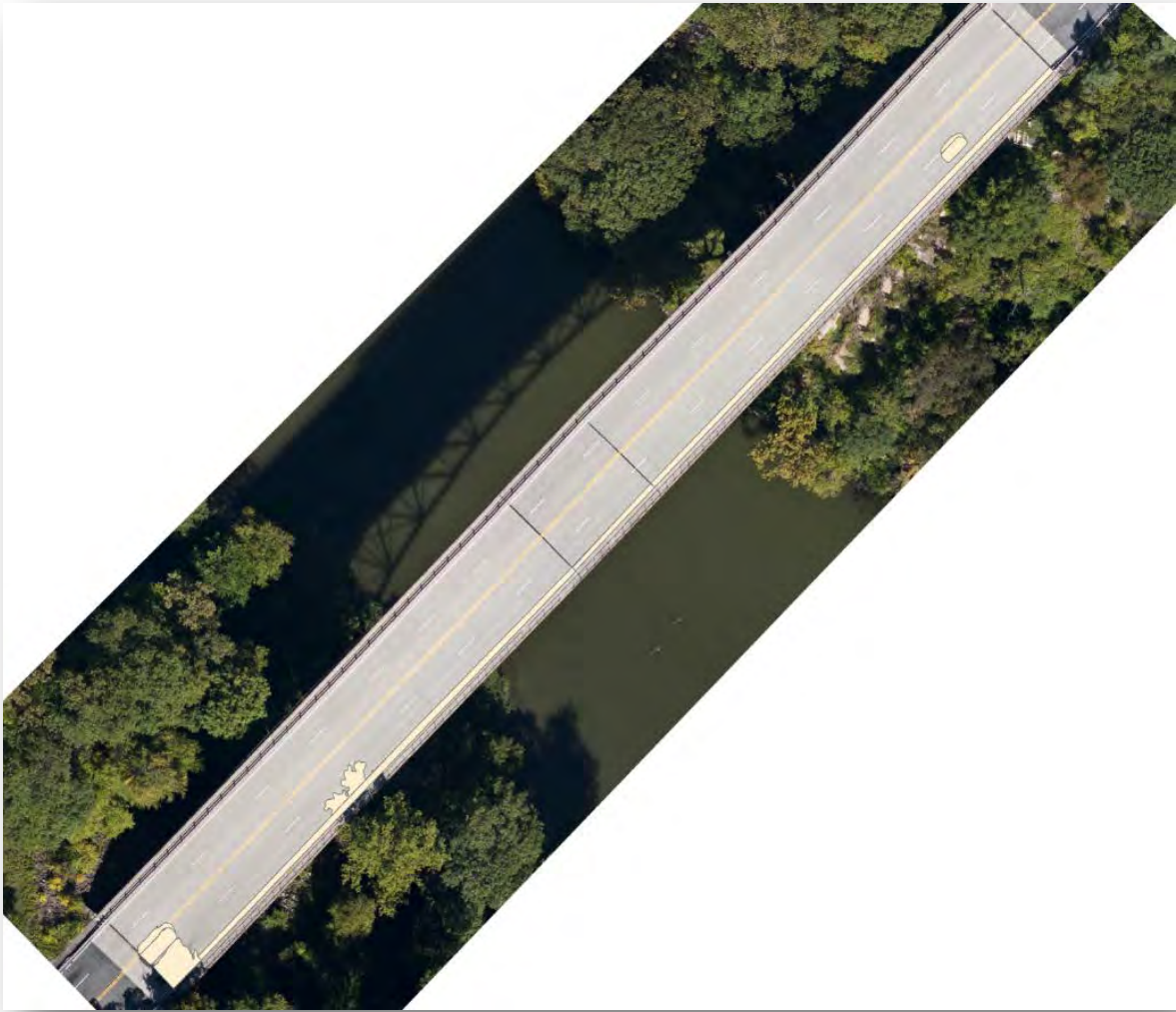
Figure C.8.11: Bridge NO. 1007150 Obstruction Image
