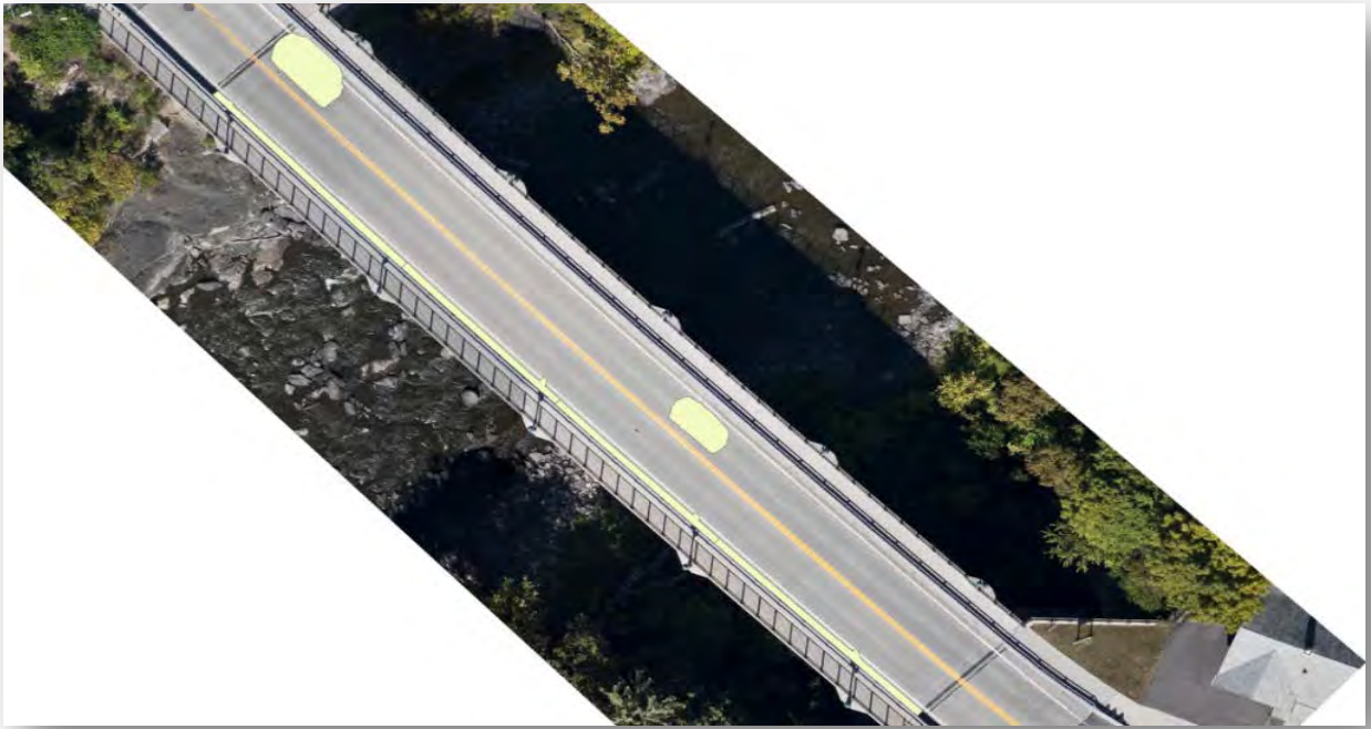
Figure C.8.26: Bridge NO. 1026680 Obstruction Image
