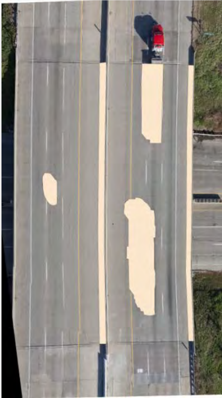
Figure C.4.8: Bridge NO. 41300-10 Obstruction Image
