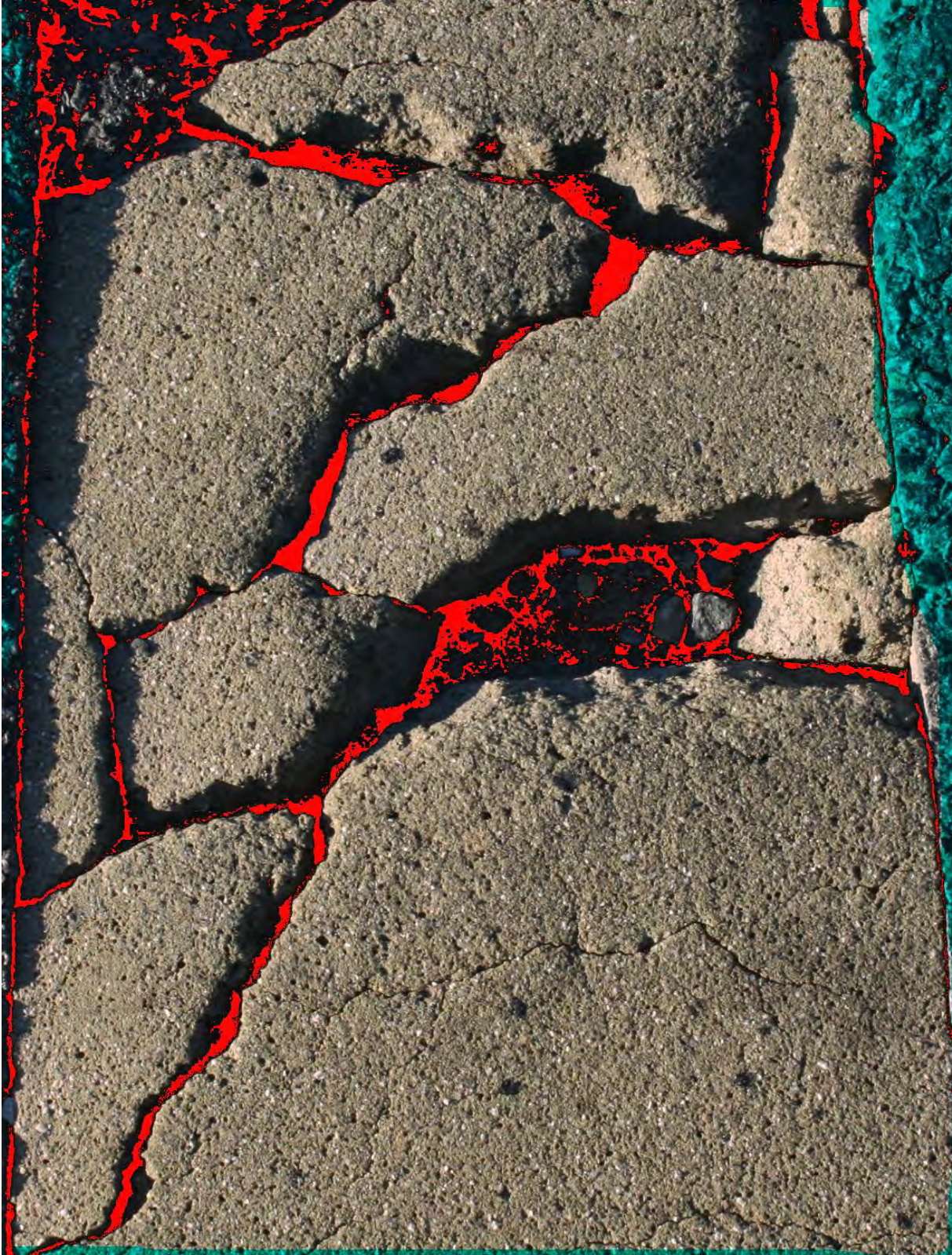
B.1.24: Original image of the area of study being marked with total damages in red pixels.
