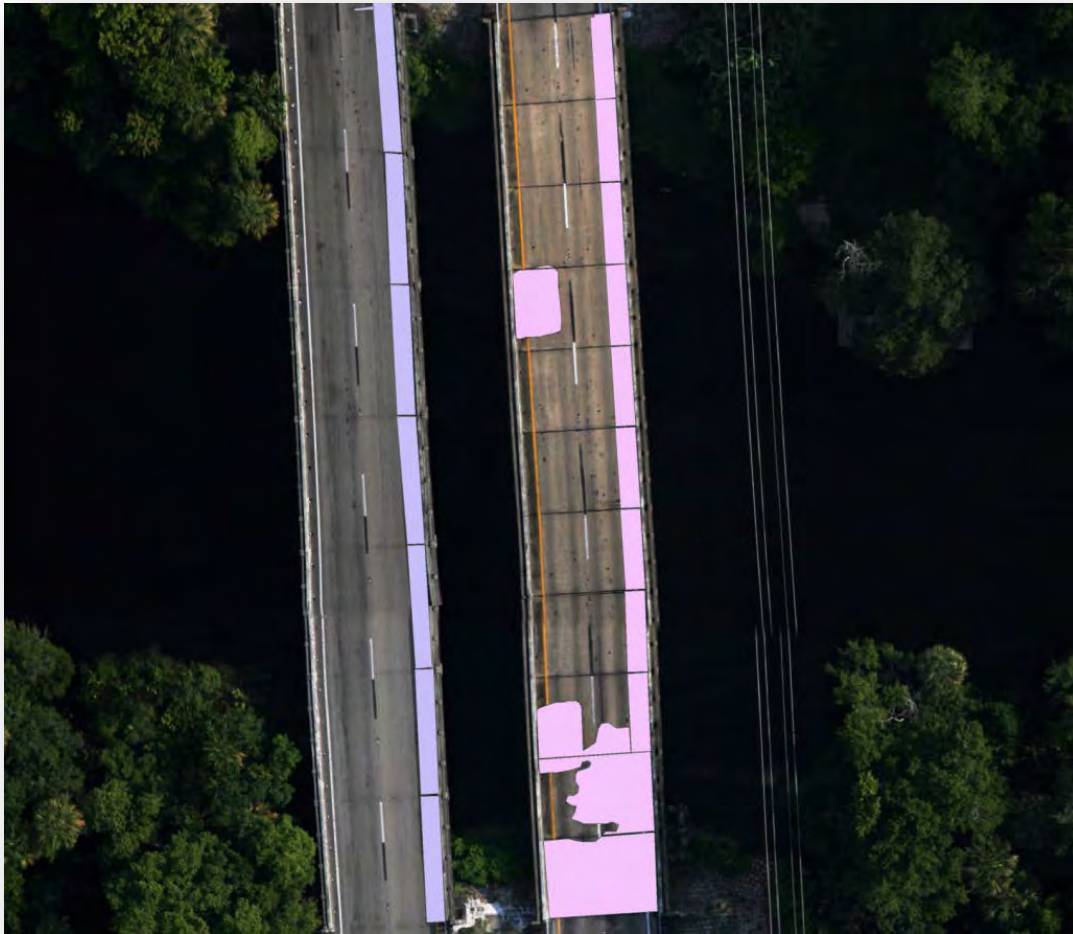
Figure C.3.214: Bridge NO. 730008 Obstruction Image
