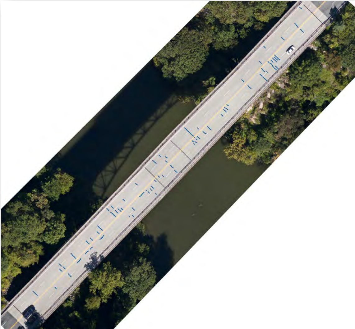
Figure C.8.12: Bridge NO. 1007150 Crack Image
