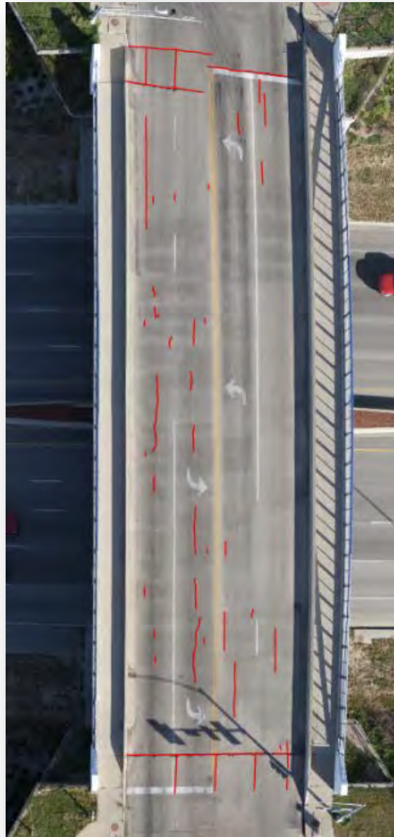
Figure C.4.18: Bridge NO. 42401 Crack Image
