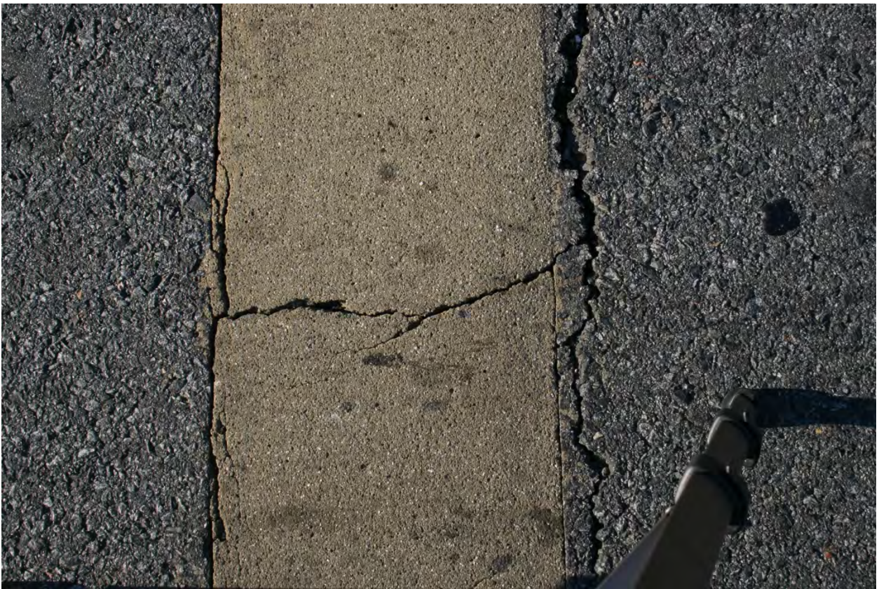
Figure 10: Ground image of Mallard creek church road bridge
