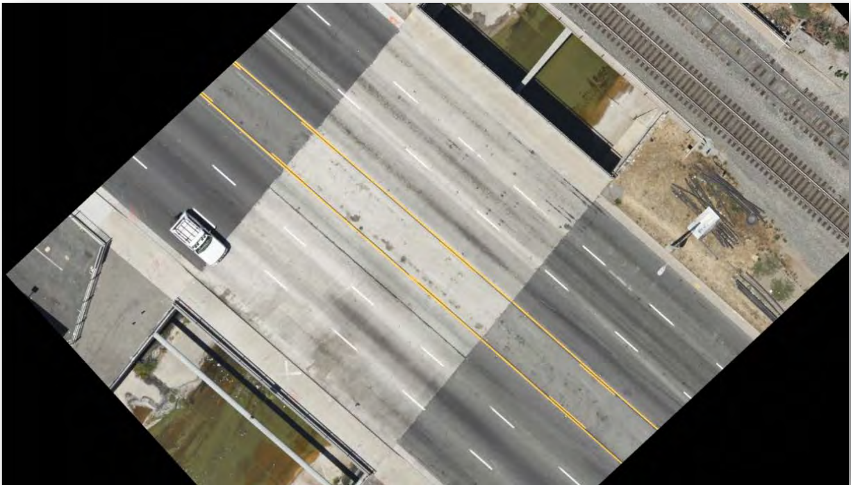
Figure C.2.2613: Bridge NO. 53C0431 Blank Image
