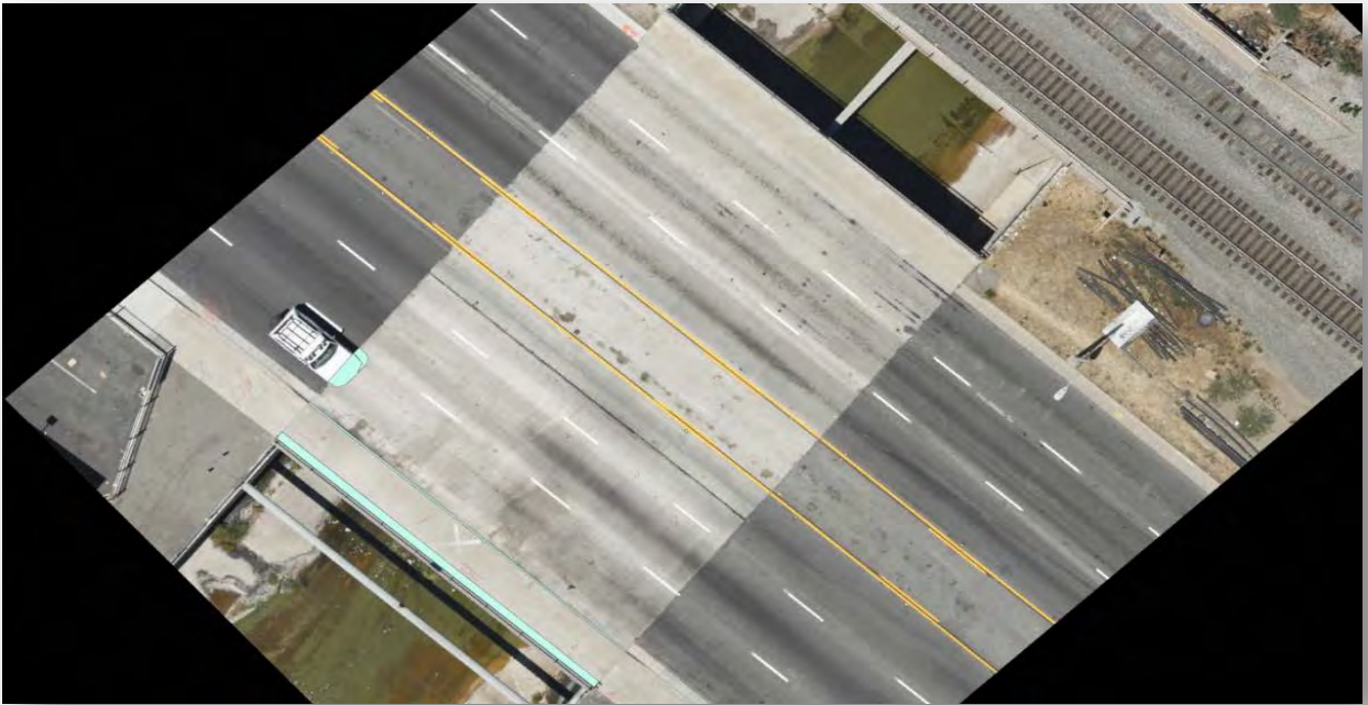
Figure C.2.27: Bridge NO. 53C0431 Obstruction Image
