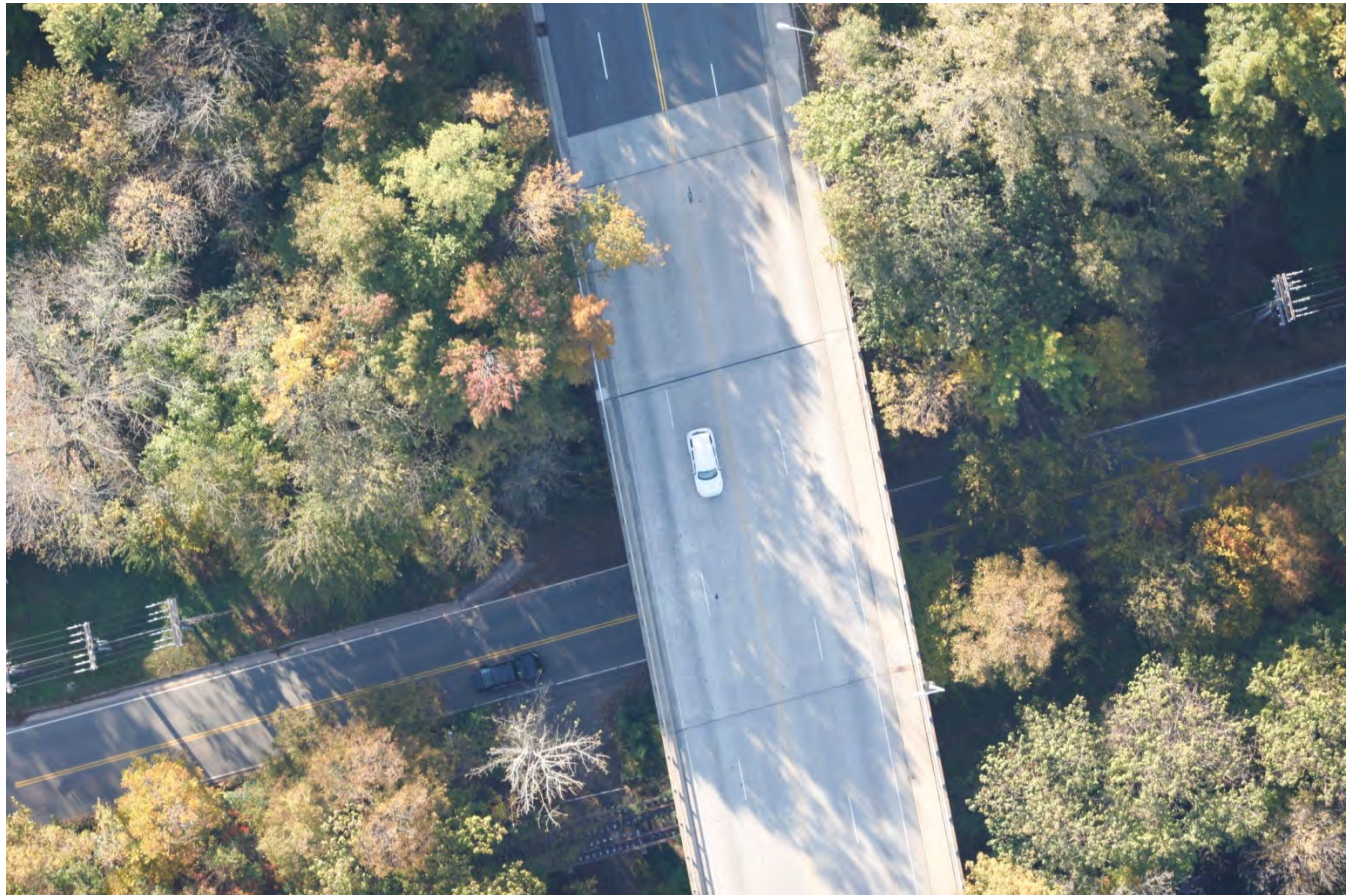
Figure 3: Heavily Shadowed Bridge Deck (SI-SFAP)
