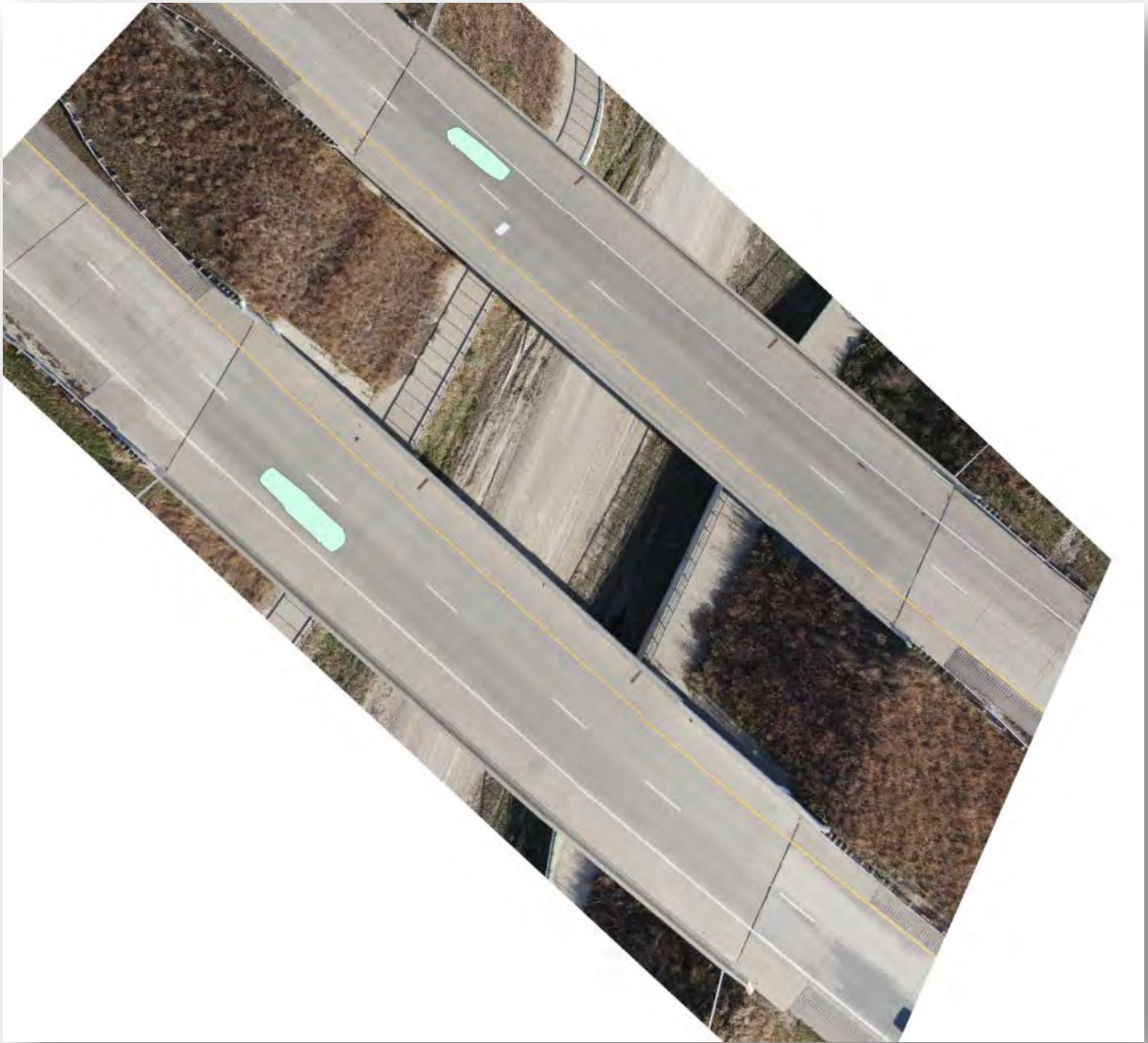
Figure C.4.35: Bridge NO. 608660 Obstruction Image
