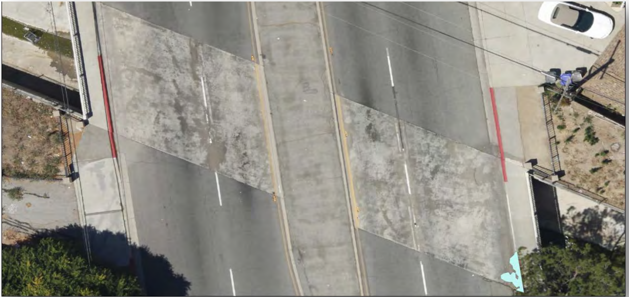
Figure C.2.13: Bridge NO. 53C0470 Obstruction Image
