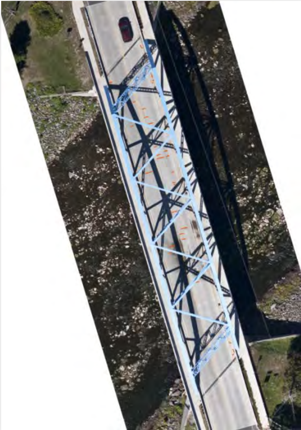
Figure C.8.24: Bridge NO. 1022310 Crack Image
