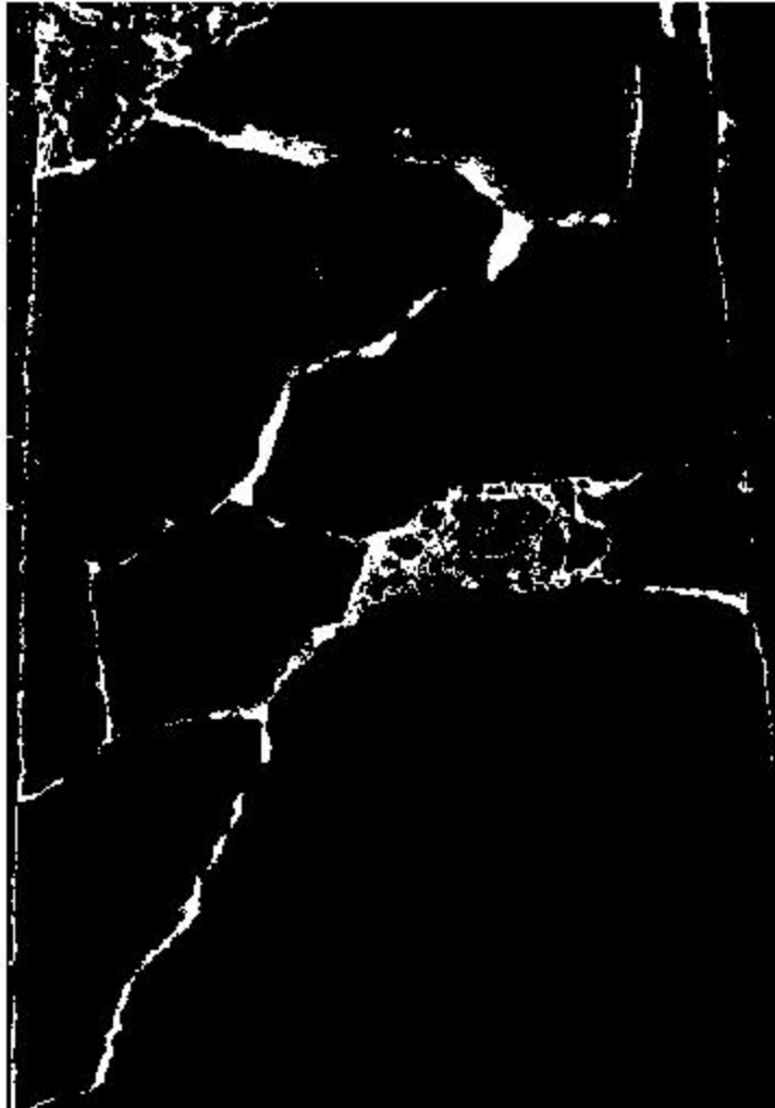
Filtered Image of Major cracks
