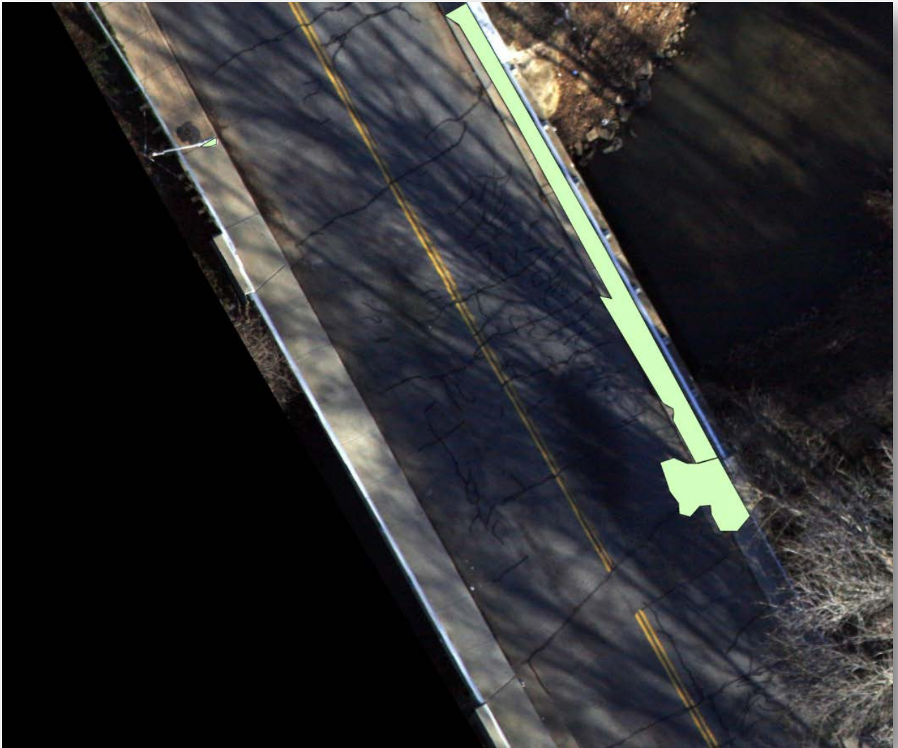
Figure C.5.2: Bridge NO. 590376 Obstruction Image
