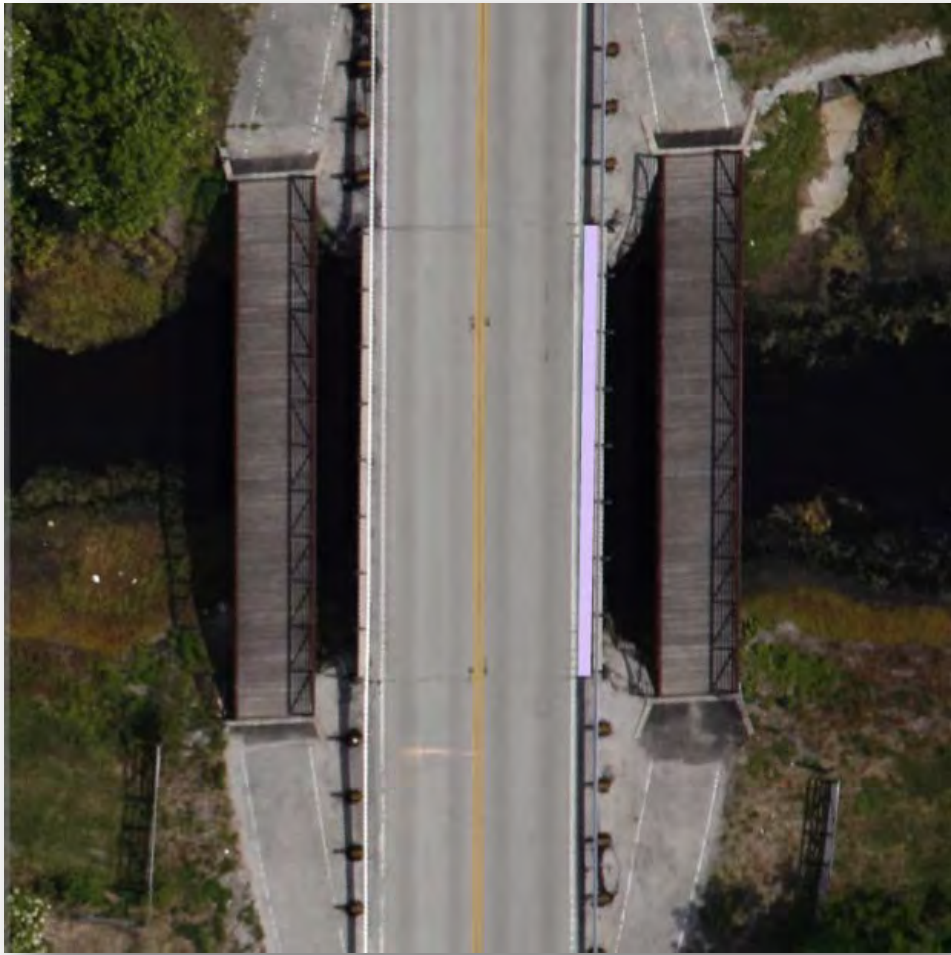
Figure C.3.14: Bridge NO. 924038 Obstruction Image
