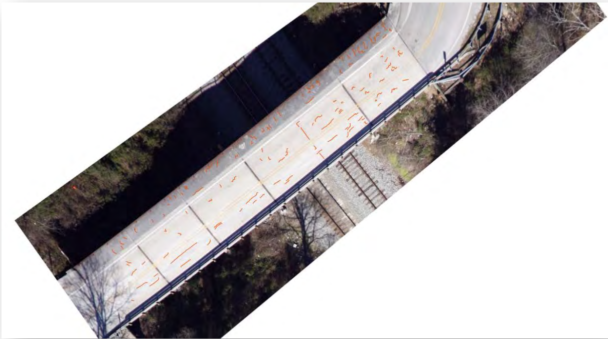
Figure C.1.5: Bridge NO. 10357 Crack Image
