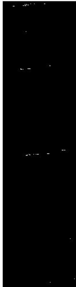
Filtered Image of Minor Cracks
