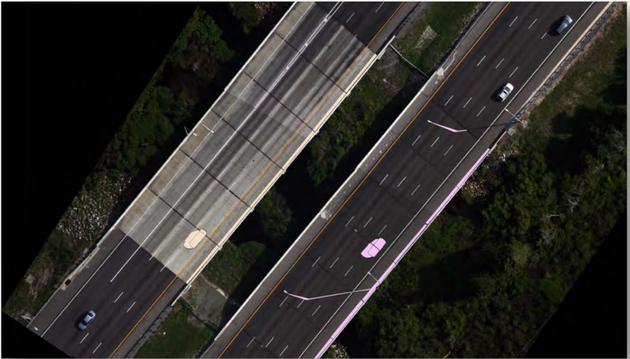
Figure C.3.11: Bridge NO. 920099 Obstruction Image
