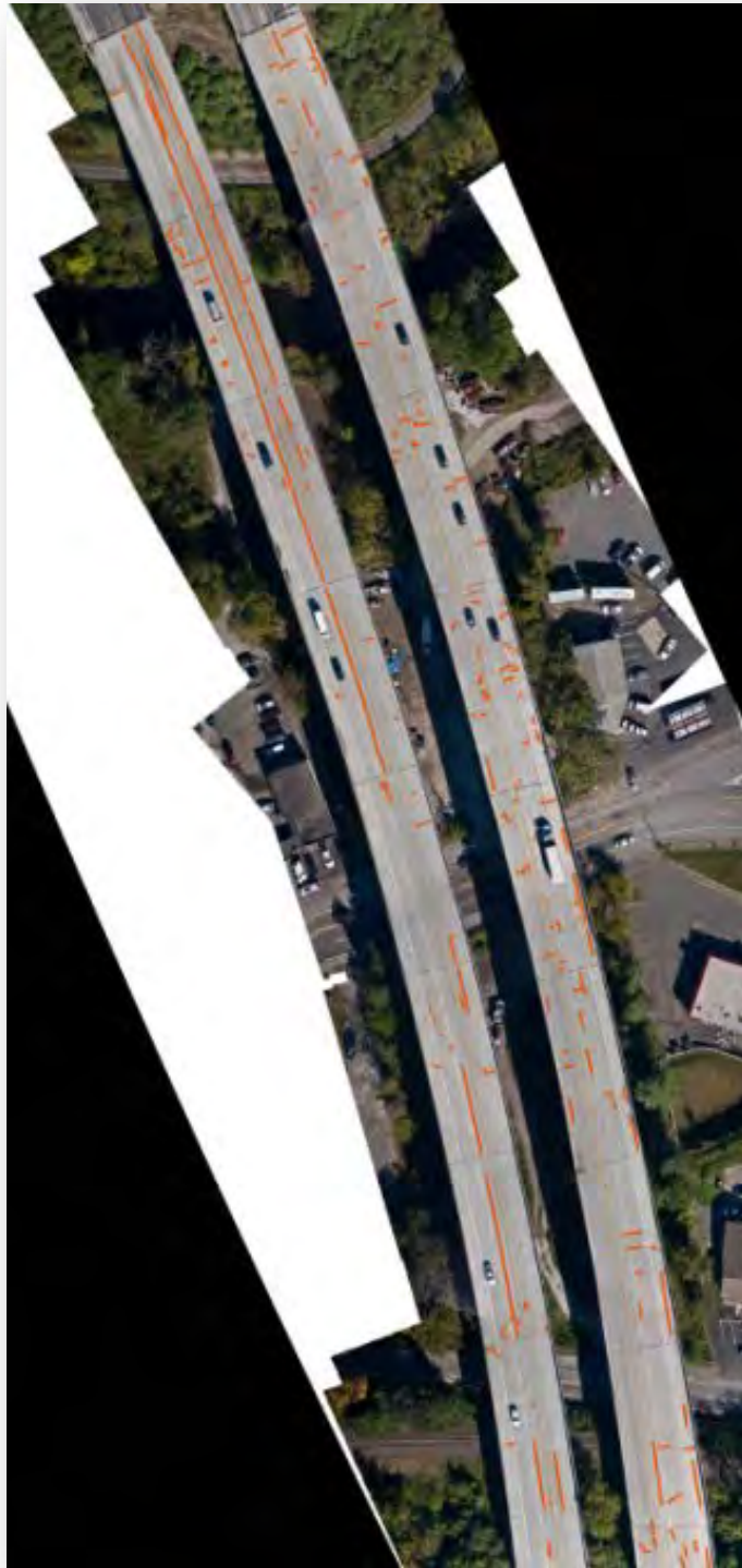
Figure C.8.36: Bridge NO. 1052841 Crack Image
