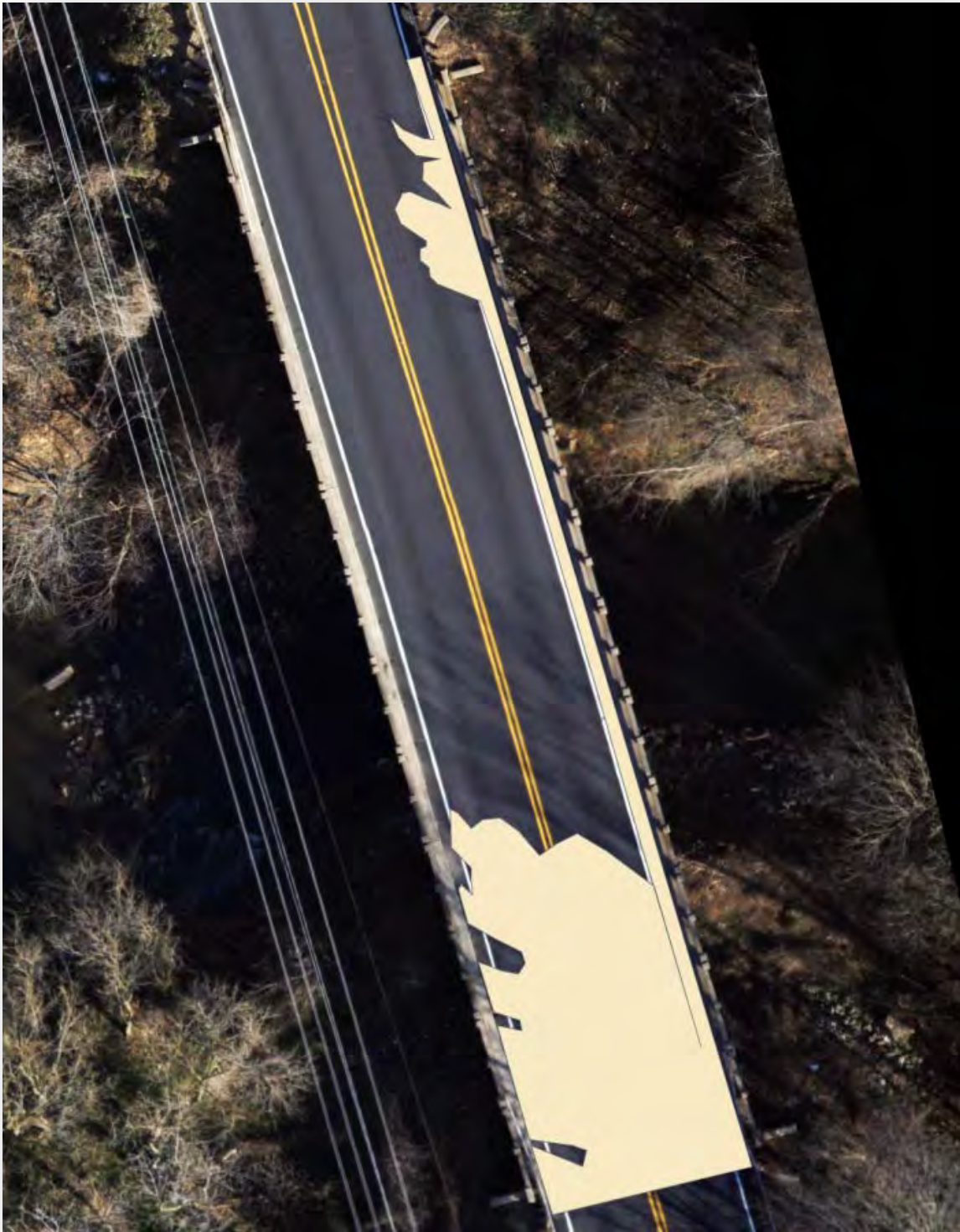
Figure C.5.8: Bridge NO. 590049 Obstruction Image
