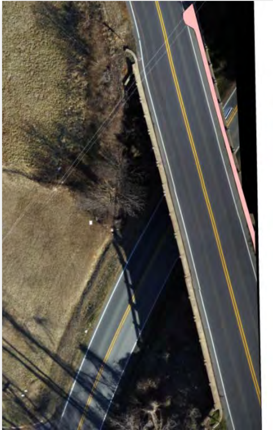
Figure C.5.23: Bridge NO. US21 St. 2004 Obstruction Image
