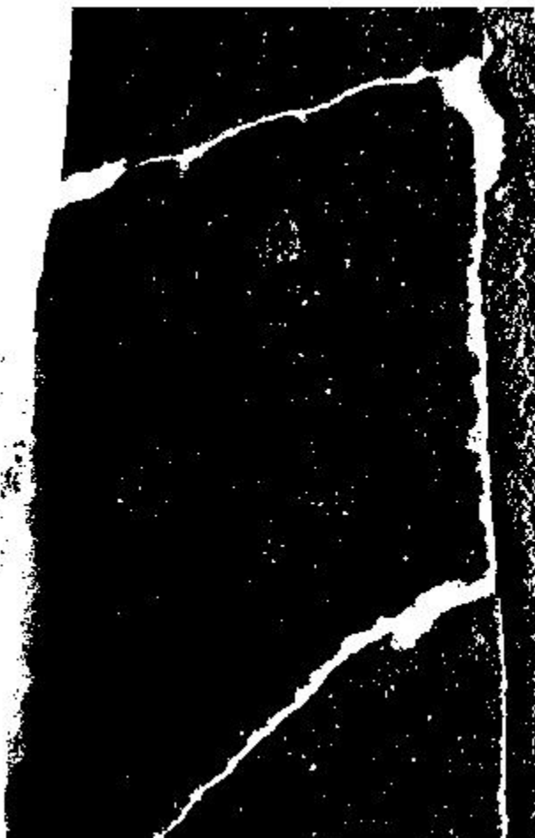
Filtered Image of Major cracks
