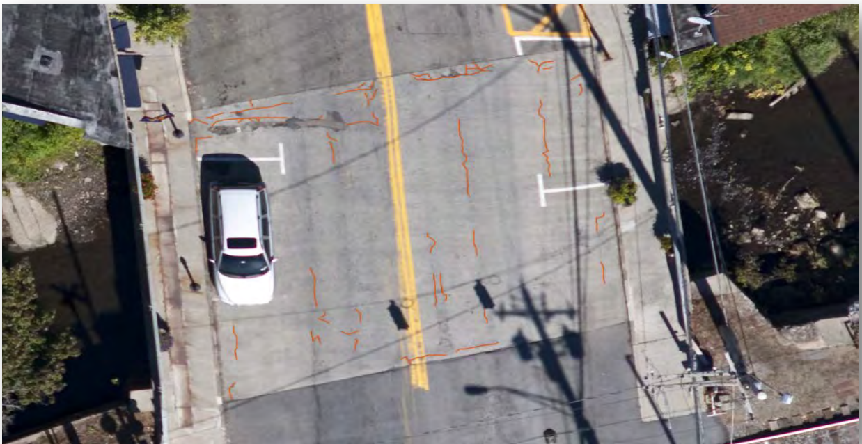
Figure C.8.21: Bridge NO. 1014090 Crack Image
