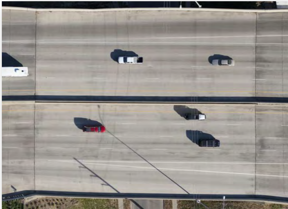
Figure C.4.13: Bridge NO. 42381-91 Blank Image
