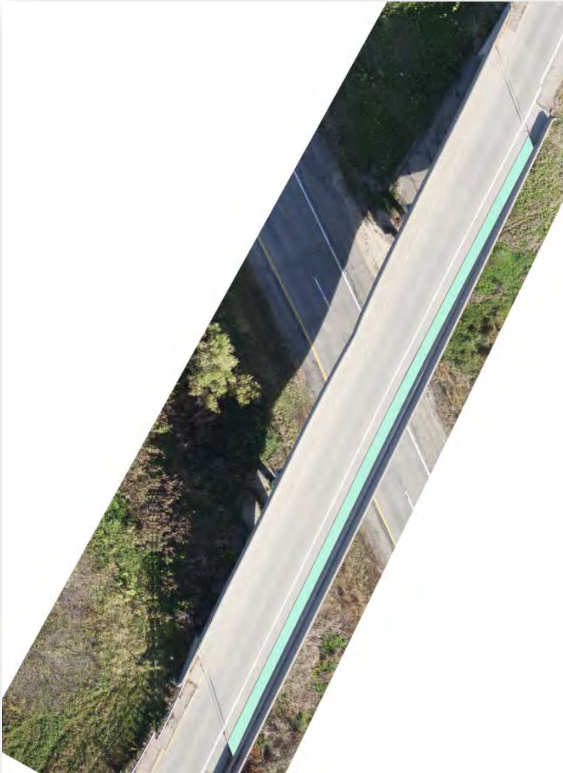
Figure C.4.23: Bridge NO. 605405 Obstruction Image
