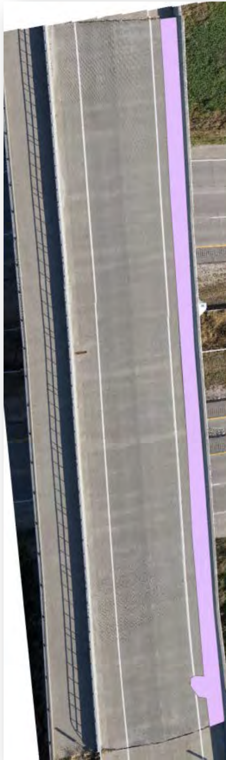
Figure C.4.29: Bridge NO. 608575 Obstruction Image
