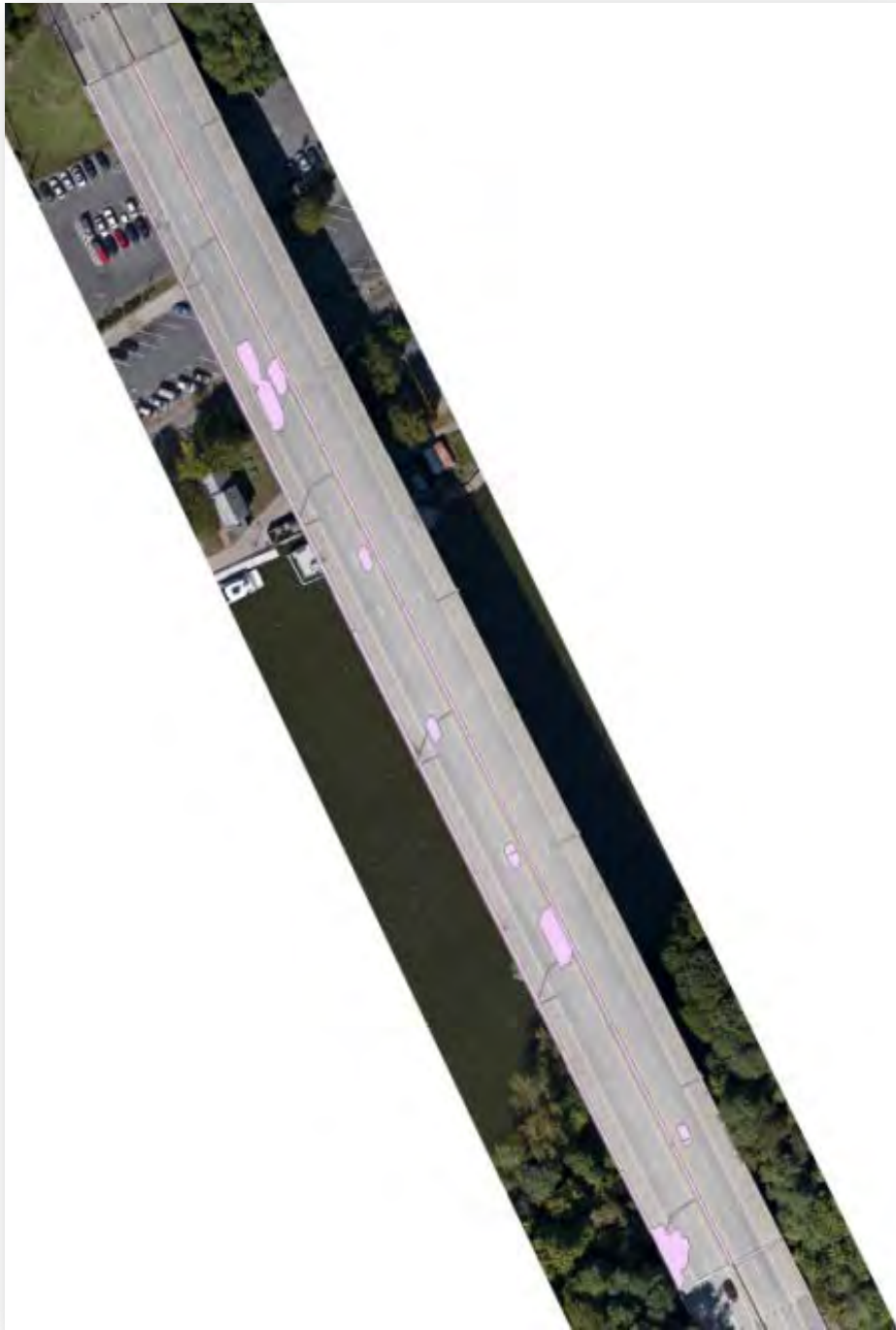
Figure C.8.41: Bridge NO. 1069749 Obstruction Image
