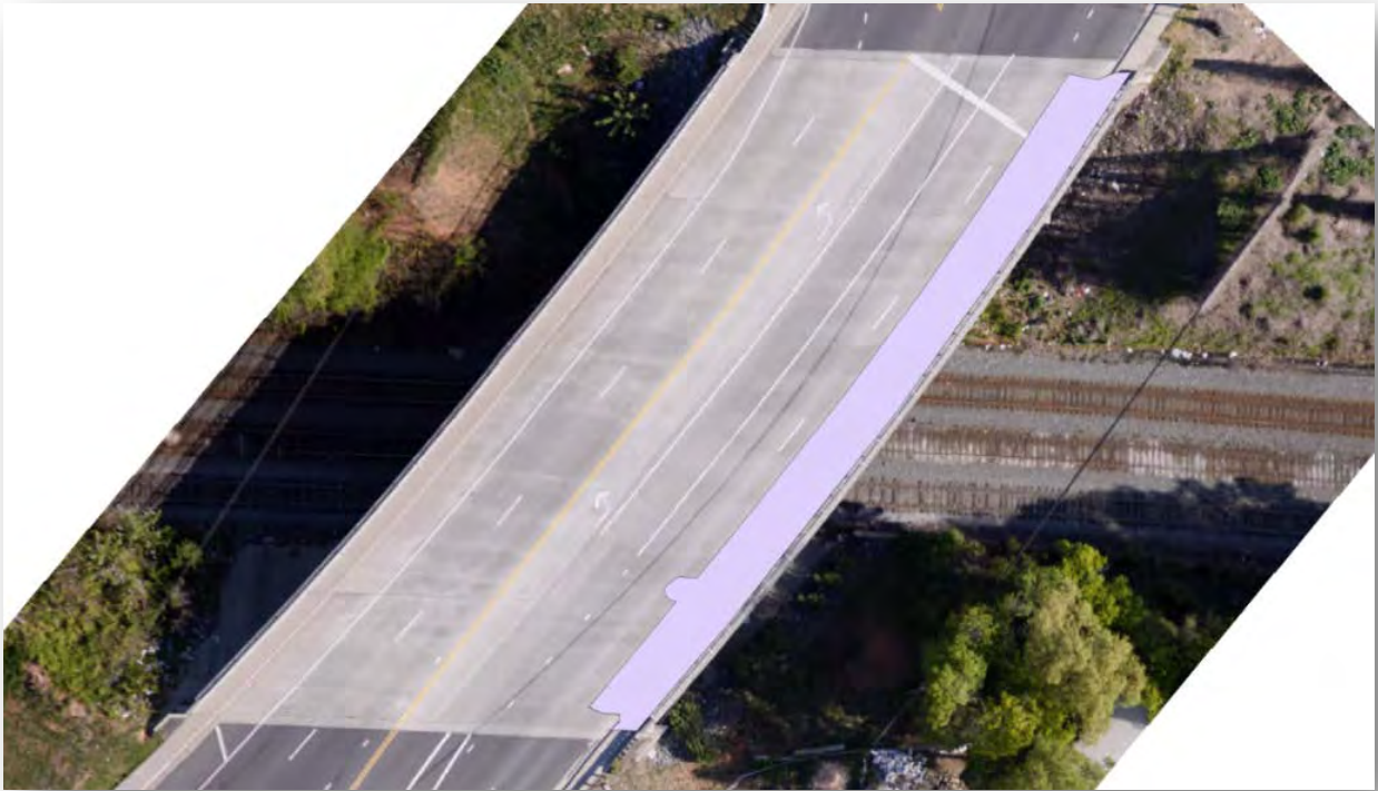
Figure C.5.5: Bridge NO. 590108 Obstruction Image
