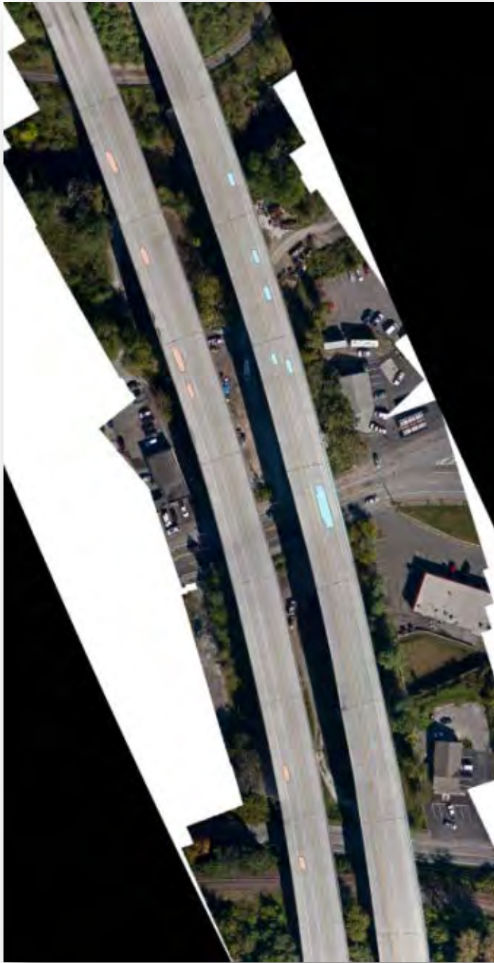
Figure C.8.35: Bridge NO. 1052841 Obstruction Image
