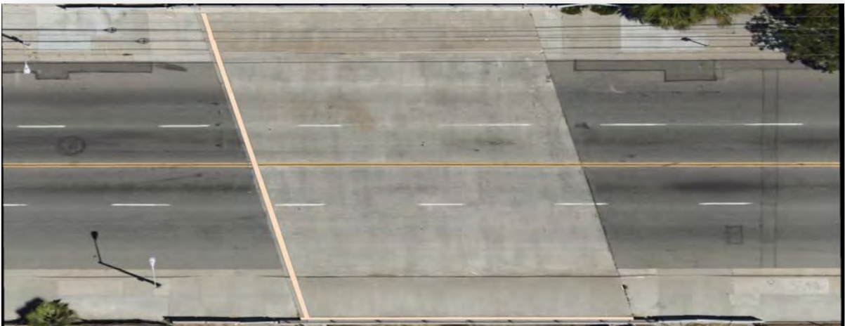
Figure C.2.29: Bridge NO. 53C0625 Obstruction Image
