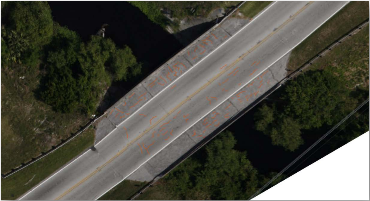
Figure C.3.25: Bridge NO. 924510 Crack Image
