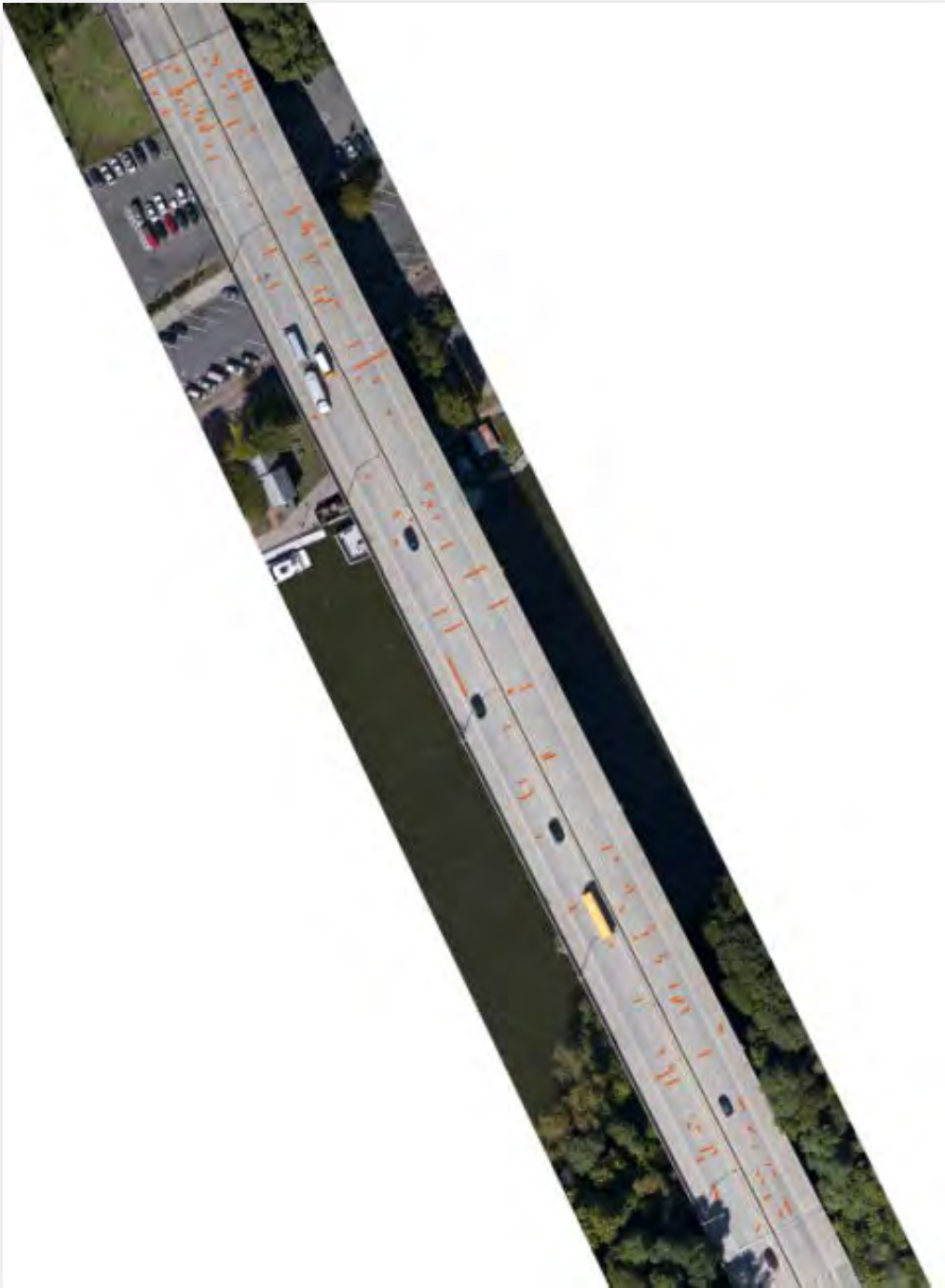
Figure C.8.42: Bridge NO. 1069749 Crack Image
