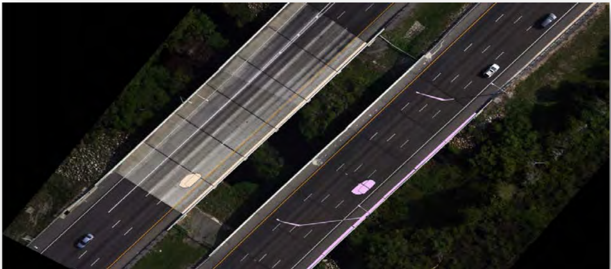
Figure C.3.8: Bridge NO. 920098 Obstruction Image
