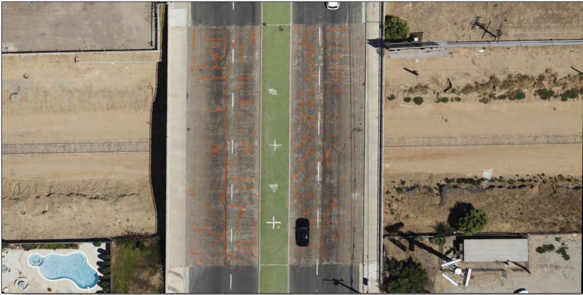
Figure C.2.31: Bridge NO. 53C0825 Crack Image
