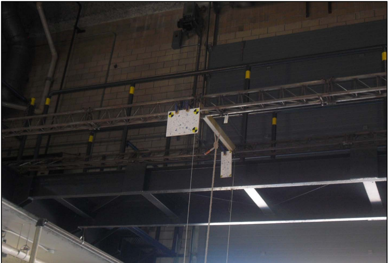
Figure 9-26: Steel bridge specimen used for continued investigations.
