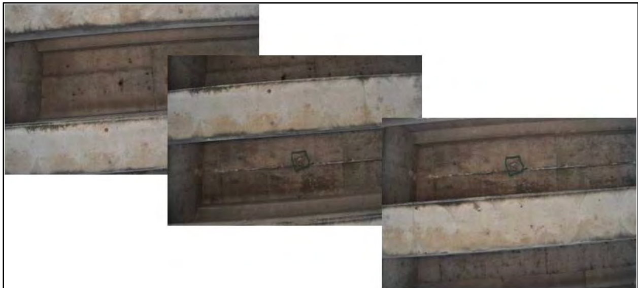
Figure 4-22: A series of photos taken during a bridge underside collect with the 3DOBS system.
