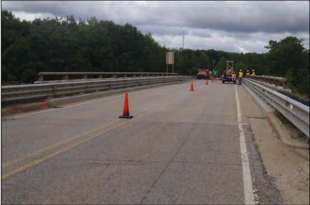
Figure 3-9: Mannsiding Road bridge SB.
