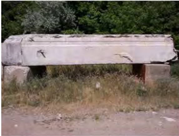
Front Face of Box Beam (closest to radar)
