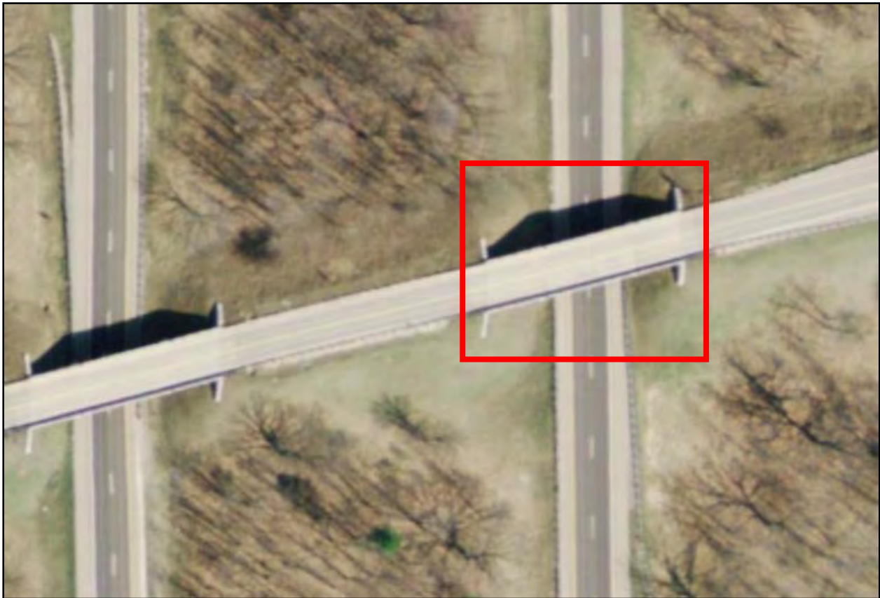
Figure 3-2: "Poor" bridge selection – Mannsiding Road NB.
