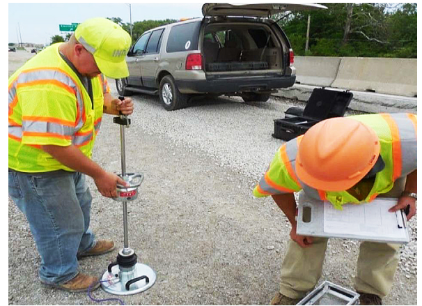
Road workers demonstrate the use of a lightweight deflectometer (LWD).
