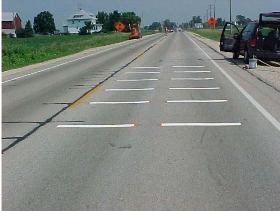
Figure 6. Temporary rumble strips
