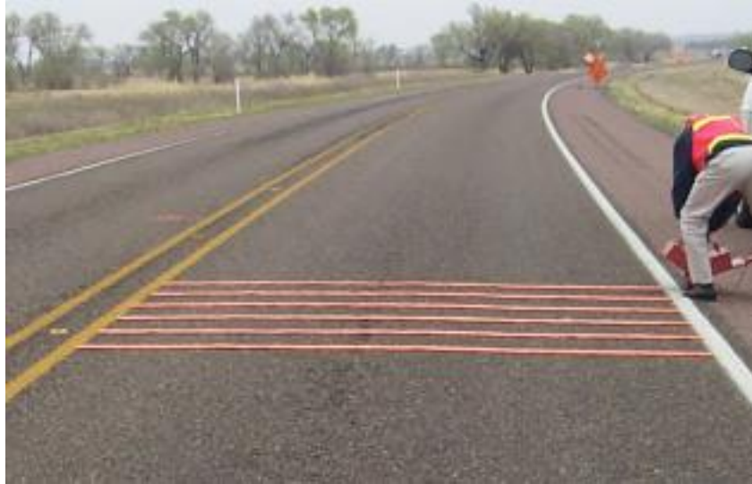
Figure 3. Rumble strip tape
