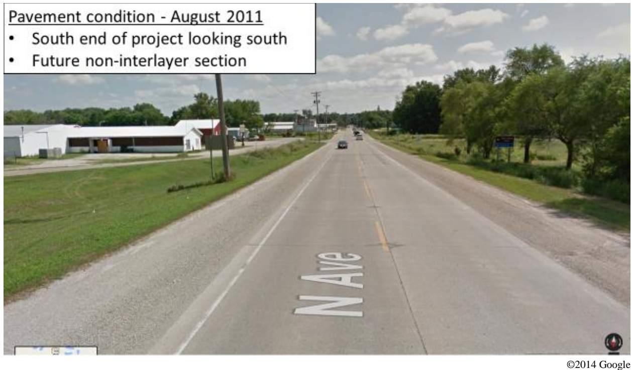
Figure 8. Pre-construction view of non-interlayer section on US 169
