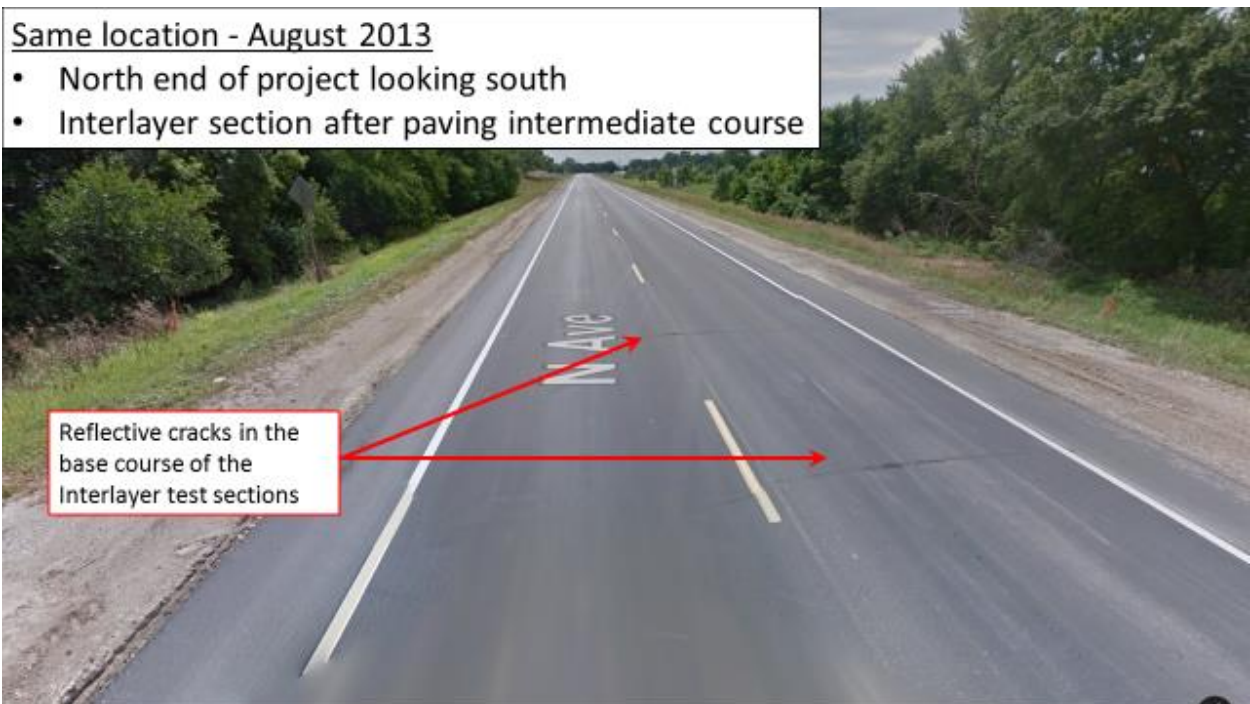
Figure 11. Post-construction view of intermediate course in interlayer section on US 169
