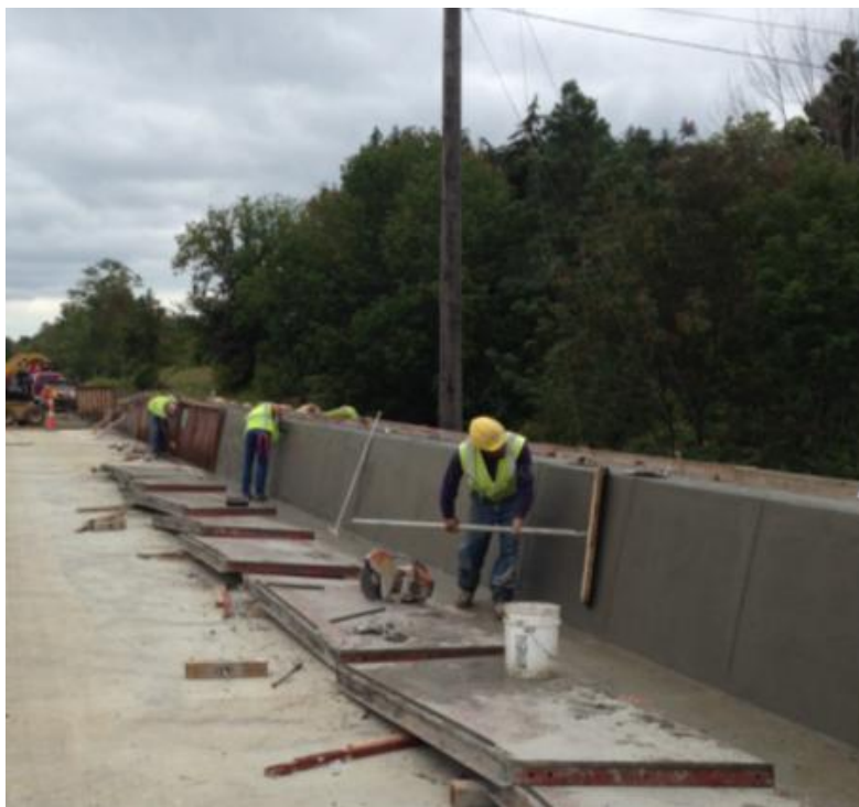
Figure 39: Rubbing the WB Paine Road north parapet (Photograph by Amy Kalabon)
