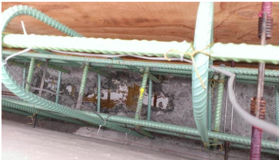
Figure 52: Placement of maturity sensors (Photograph by Amy Kalabon)
