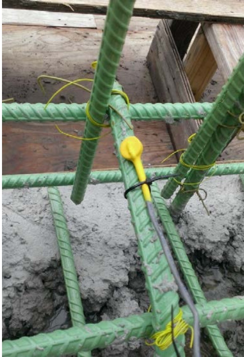
Figure 2: Maturity Sensor Attached to Reinforcement (Photograph by Amy Kalabon)
