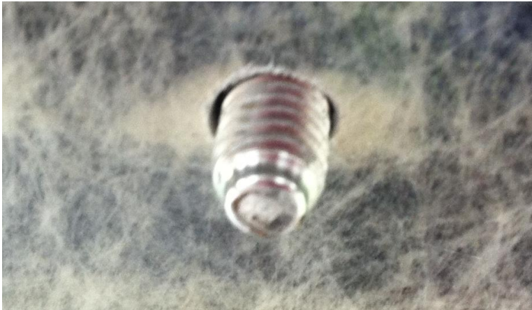
Figure 17 Swedge Bolt Anchored (VTrans 2014)
