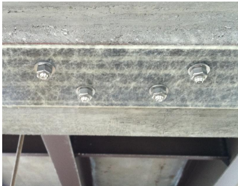
Figure 11 Completed Pattern of Bolts (VTrans 2014)
