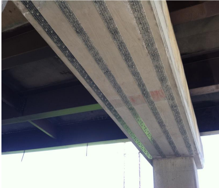
Figure 12 Completed FRP Installation (VTrans 2014)
