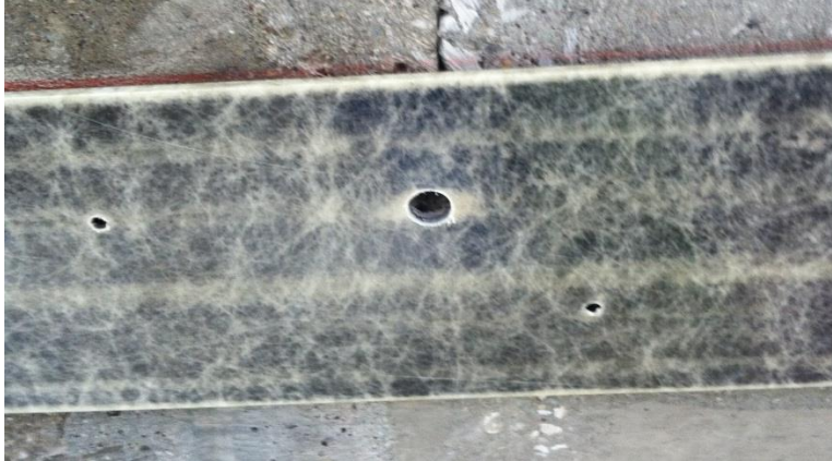
Figure 16 Drilled holes in FRP strip and concrete were \frac{3}{8} -inch (VTrans 2014)
