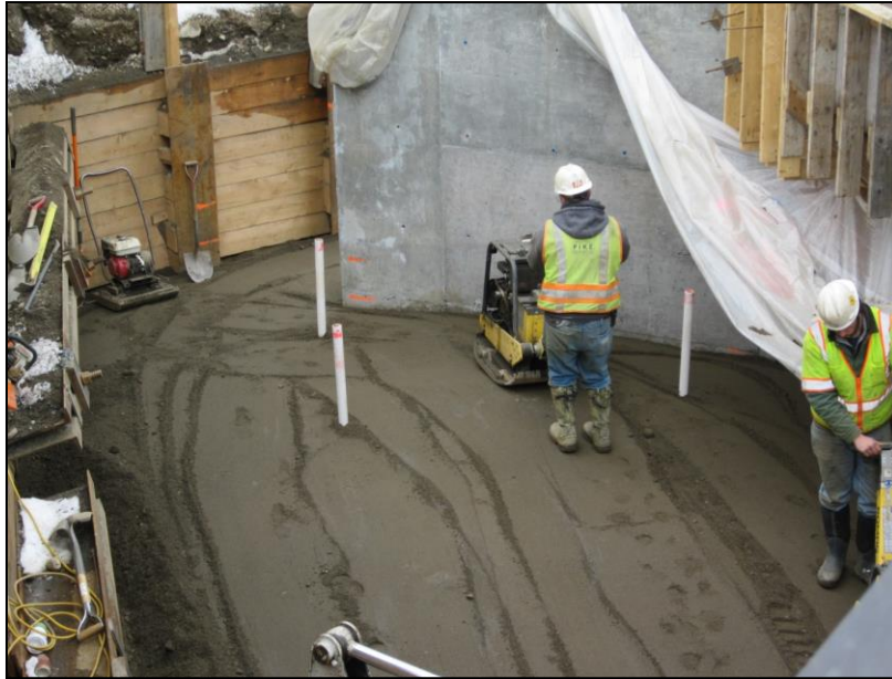
Figure 5.2: Bridgewater piezometer installation
