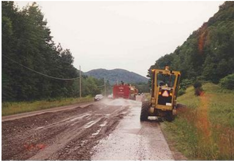
Figure 4 Water application during RSB construction
