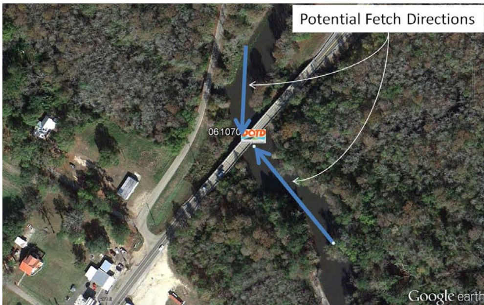
Figure 18 Aerial photograph of bridge removed from consideration because of limited fetch
