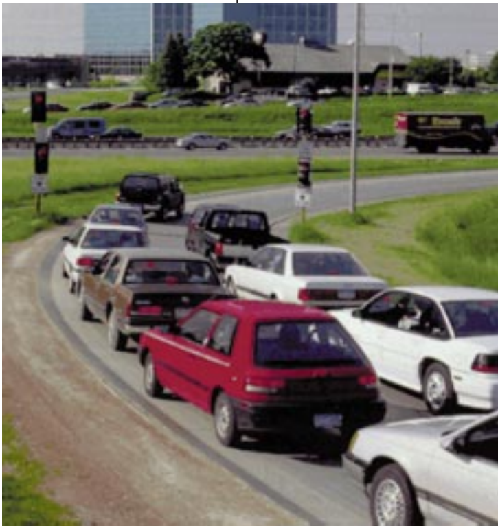
A ramp meter releases traffic to the freeway to avoid a breakdown in mainline traffic flow. Photo courtesy of Federal Highway Administration.
