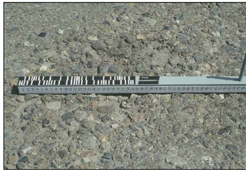
FIGURE 42 Distress Type ACP 13—Loss of Coarse Aggregate.
