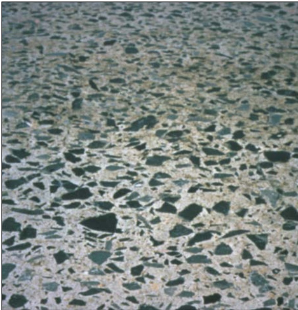
FIGURE 72 Distress Type JCP 9—Polished Aggregate.
