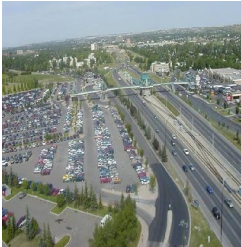
Large park-and-ride facilities and LRT station in expressway median
