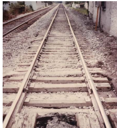
October, 1984 – Before Renewal
