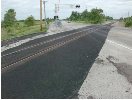
2013 After Replacing Concrete Surface with a Timber/Asphalt Surface
