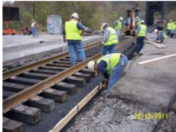
November 2011 During the Installation
