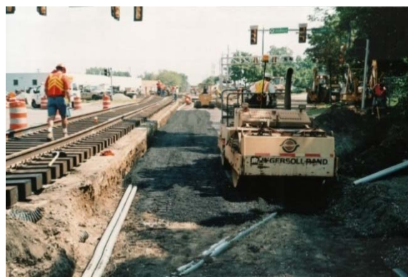
2005, Compacting the Asphalt Underlayment
