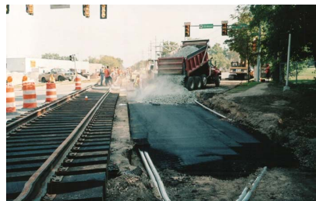
2005, Dumping the Ballast on the Underlayment
