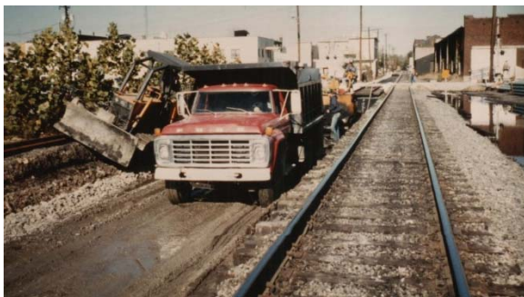
October, 1984 – During Paving
