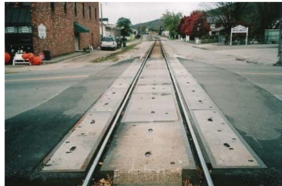
October 2006 After Surfacing/ Replacing Panels
