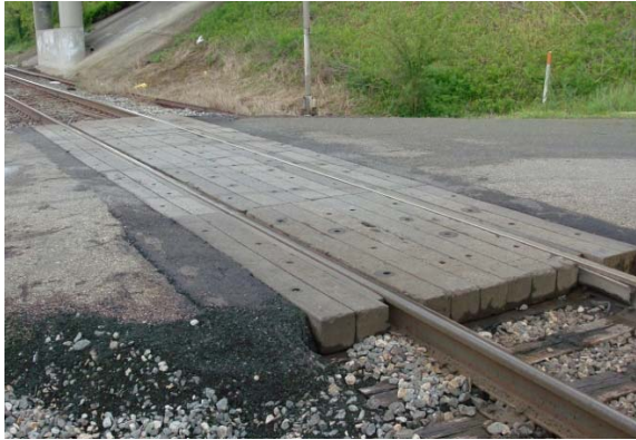
2011 After Changing out Rail and Replacing Composite Surface. Still in Perfect Condition
