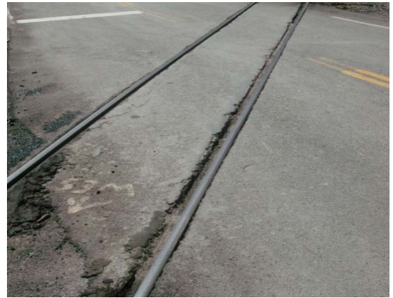
2011, Still Smooth, Slight Amount of Raveling of the Asphalt Next to the Flangeway
