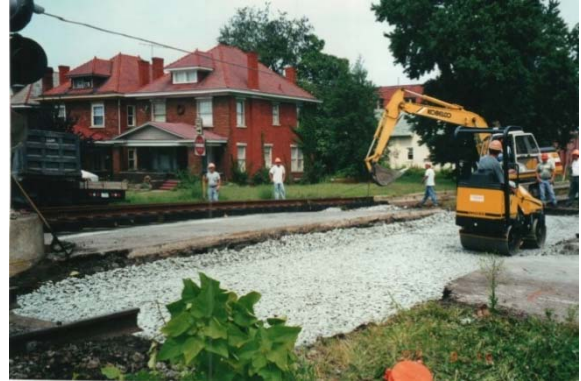
2000, Compacting the Ballast
