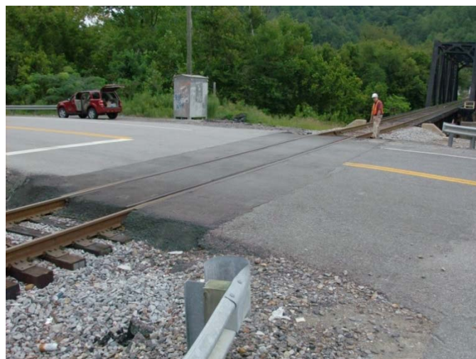
2012, Excellent Performance of the "Ballastless" Crossing
