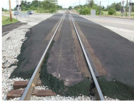
2013 After Replacing Concrete Surface with a Timber/Asphalt Surface
