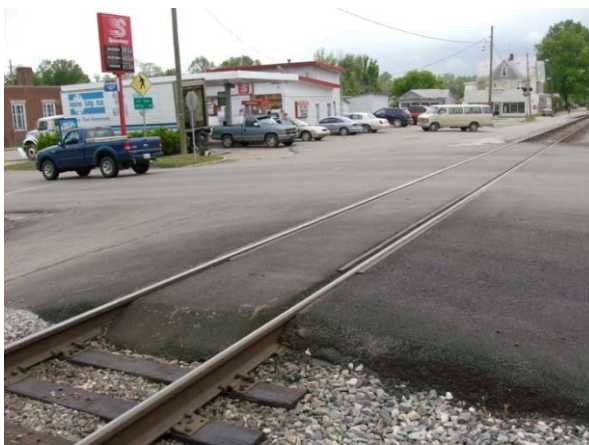
2011 – Converted to Rubber Seal/Asphalt in 2010
