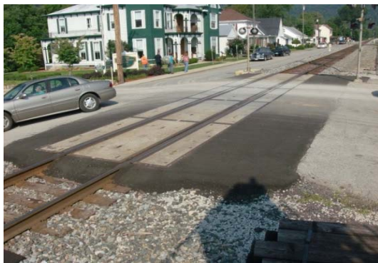
2013, After Removing Panels, Surfacing Through, and Repaving Approaches
