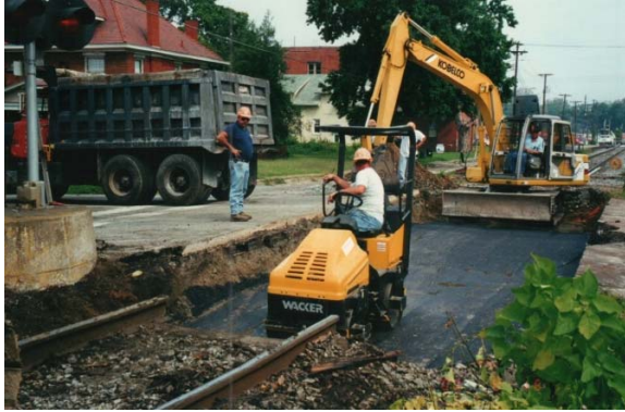
2000, Compacting the Asphalt Underlayment
