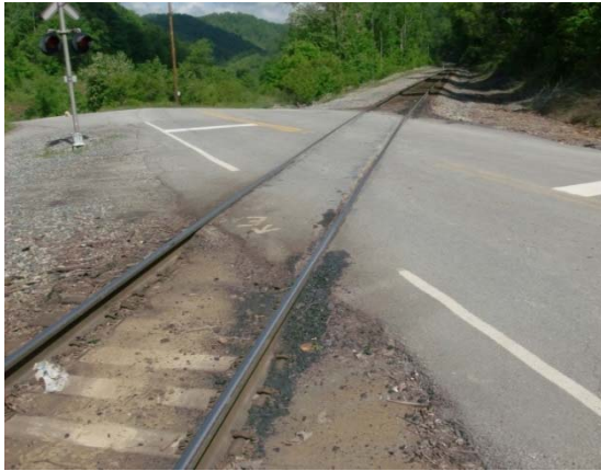
2011, Still Smooth, Slight Amount of Raveling of the Asphalt Next to the Flangeway
