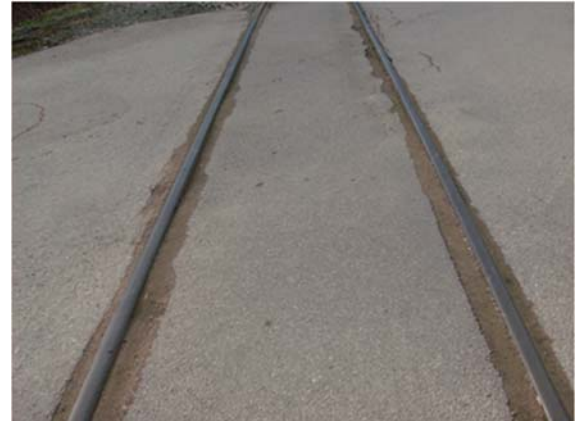
2013, Similar Condition, Slight Raveling of Flangeways
