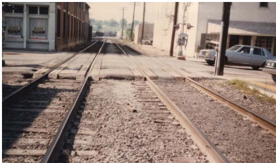
October, 19984 – Before Renewal
