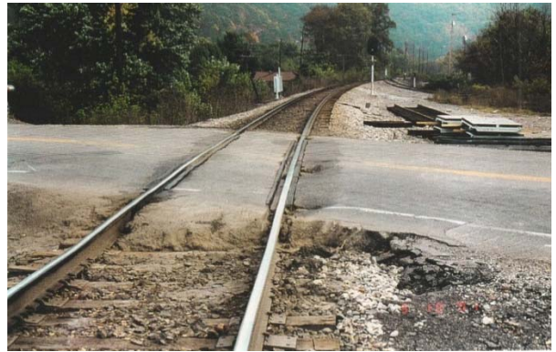
October, 2001 – Before Renewal
