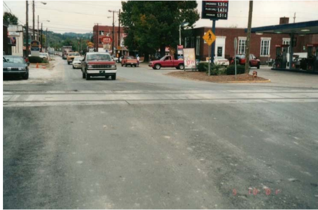
November 2001-After Renewal with Concrete
