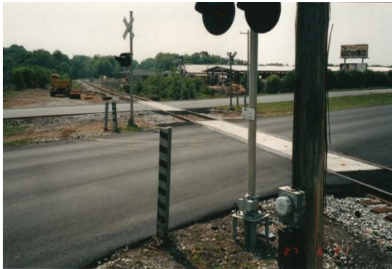
Finished Project, Two Weeks Later
