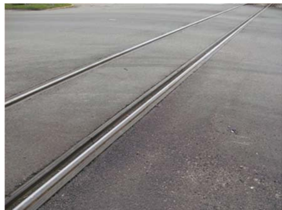
2011 – Converted to Rubber Seal/Asphalt in 2010
