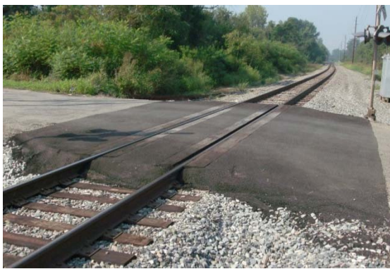
2013 After Renewing with Timber/Asphalt Surface Earlier in the Year
