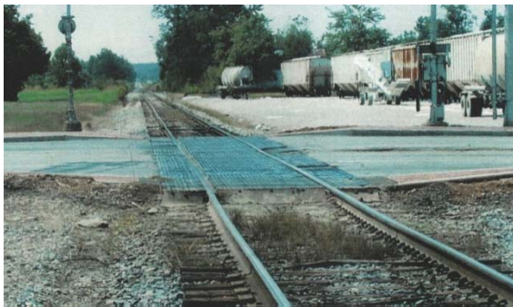
2009- Mainline Before Renewal
