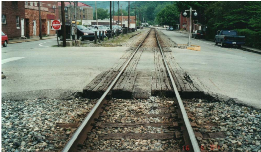
2002- Before Renewal with Concrete Surface
