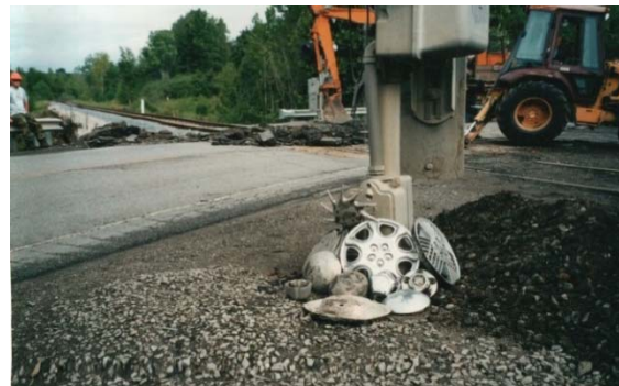
2002 Removing the Old Surface
