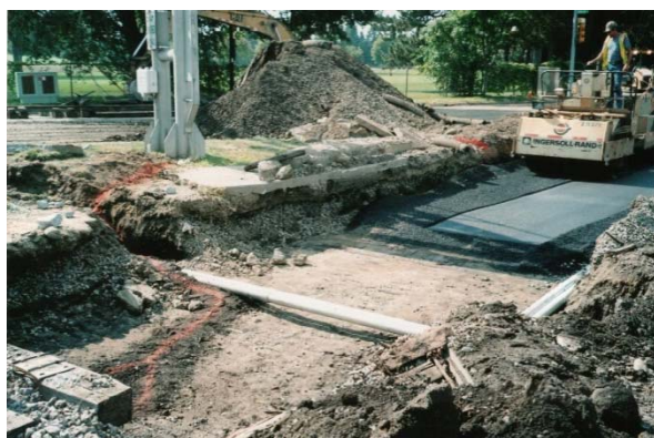
2005, Compacting the Second Lift
