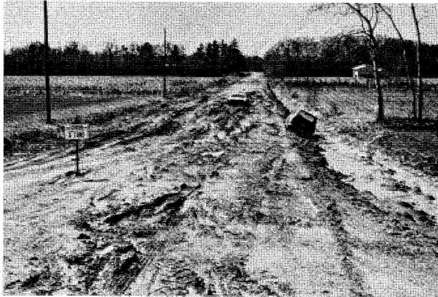
Figure 20. Severe frost boil within an alluvial area several miles southwest of Alburnett sections, April 1978.
