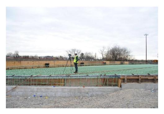
Figure 14 Scanning the rebar surface
