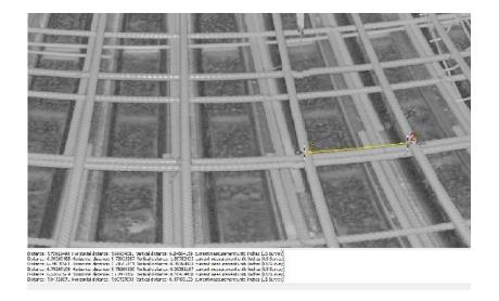
Figure 23 Spacing of top transverse rebar
