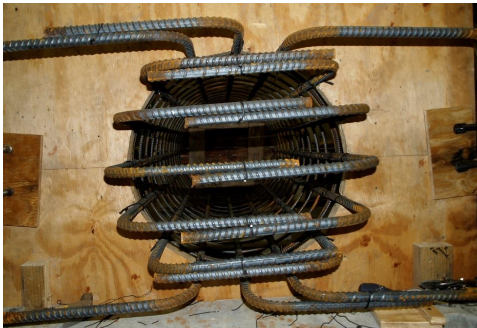
Figure 2.22 Longitudinal Column Rebar Bends in the Footing
