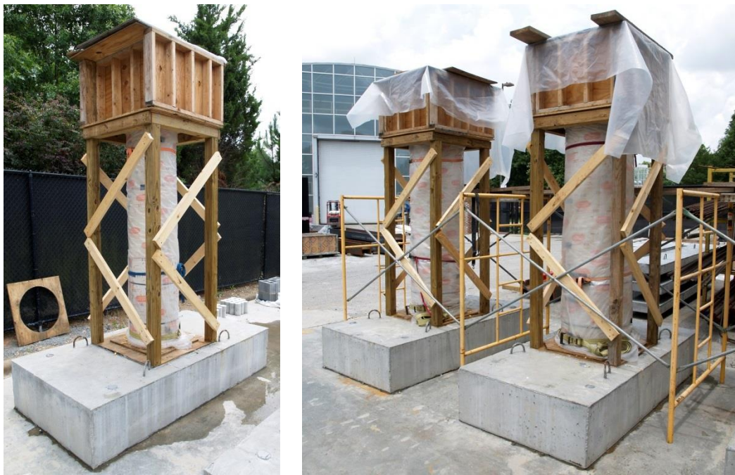
Figure 2.32 Column Stabilization and Cap Formwork
