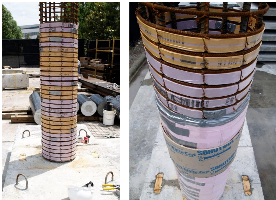
Figure 2.30 Installation of 2-Layer Full Cover Concrete Blockout
