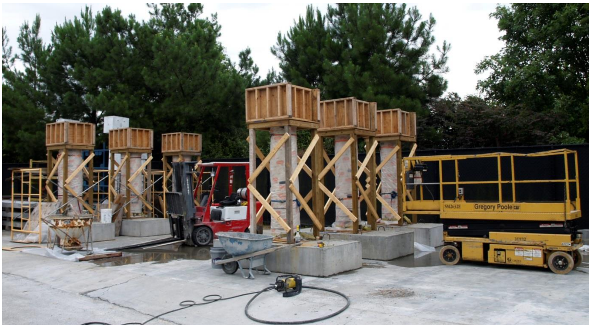
Figure 2.34 Casting with Fork Lift, 1/3 Cubic Yard Hopper, and 13' Concrete Vibrator
