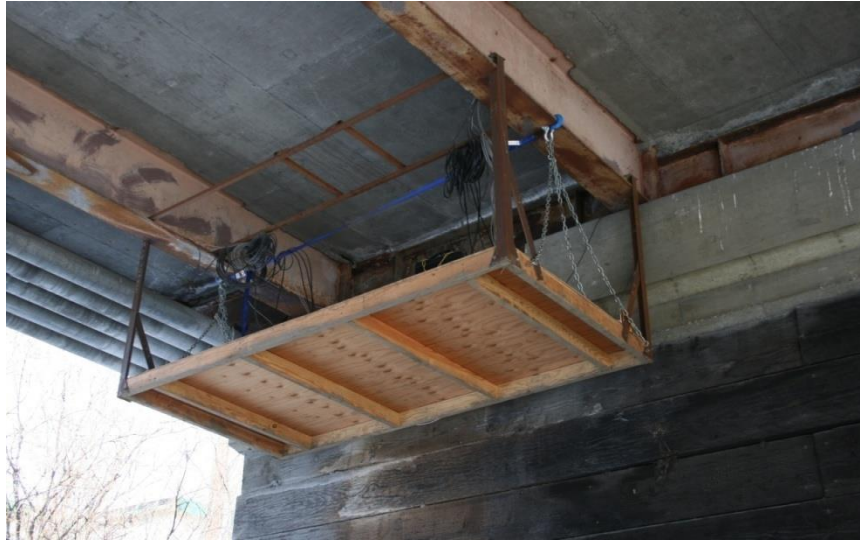
Figure 3.4 Hanging rolling platform
