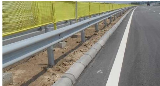
Fig. 1.1: A W-beam guardrail behind a curb.
