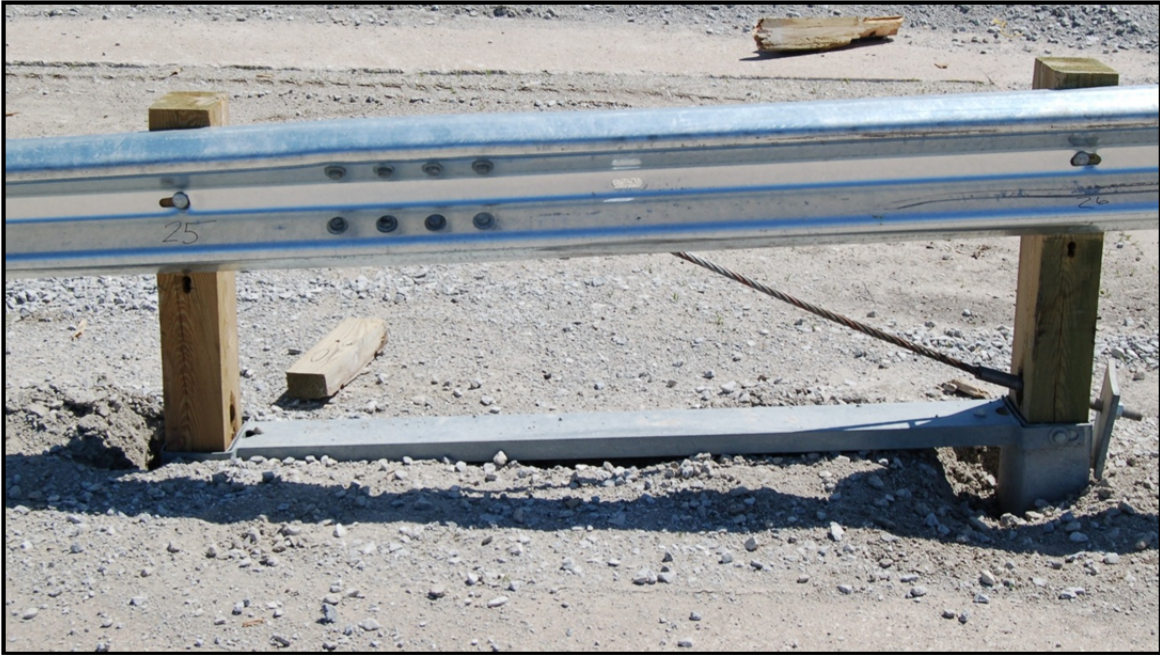
(a) Downstream Anchor, Test No. LSC-1
