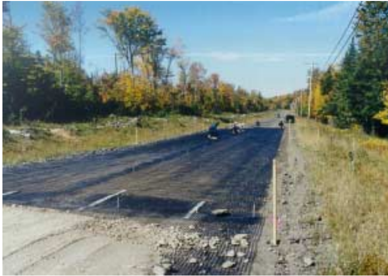
Geogrid Placement 50-meter length - full roadway width
