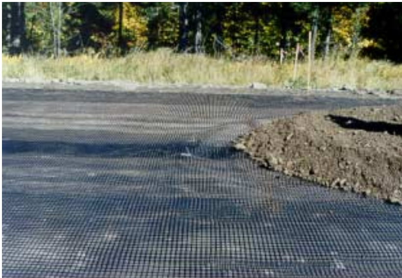
Variable Depth Gravel Placement
