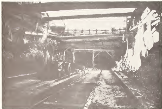
Red Line, outbound of the Dupont Circle Station, during construction through the Rock Creek Park west of Connecticut Avenue. A cut-and-cover section will connect with the twin earth tunnels in background, leading to the Woodley Park-Zoo Station (WMATA photo by Phil Portlock)
