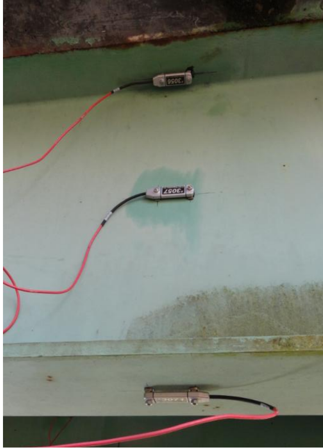
Figure 2 - Cross-section view of interior girder.
