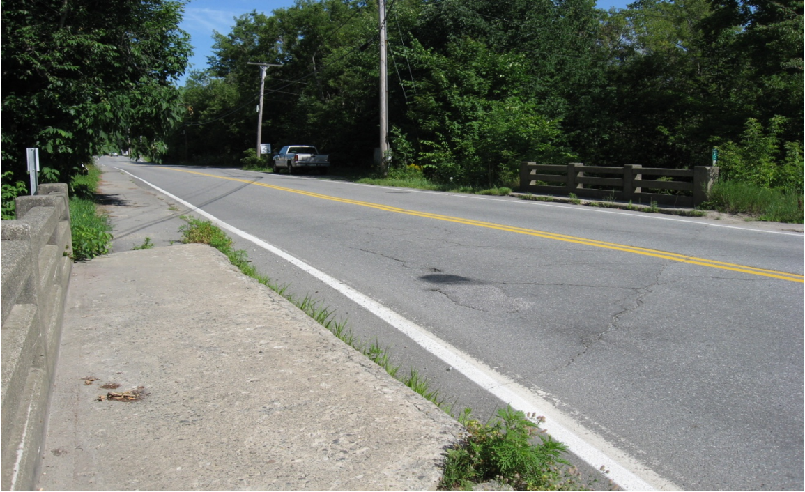
Figure 31 - Photo of Brewer Bridge #5638 from Bridge Visit Conducted in July 2010
