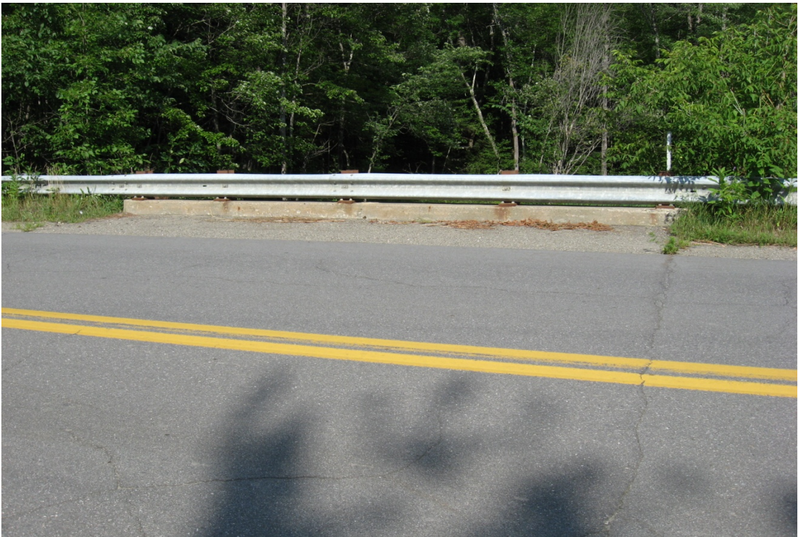
Figure 48 - Photo of Palmyra Bridge #5699 Rail from Bridge Visit Conducted in August 2010
