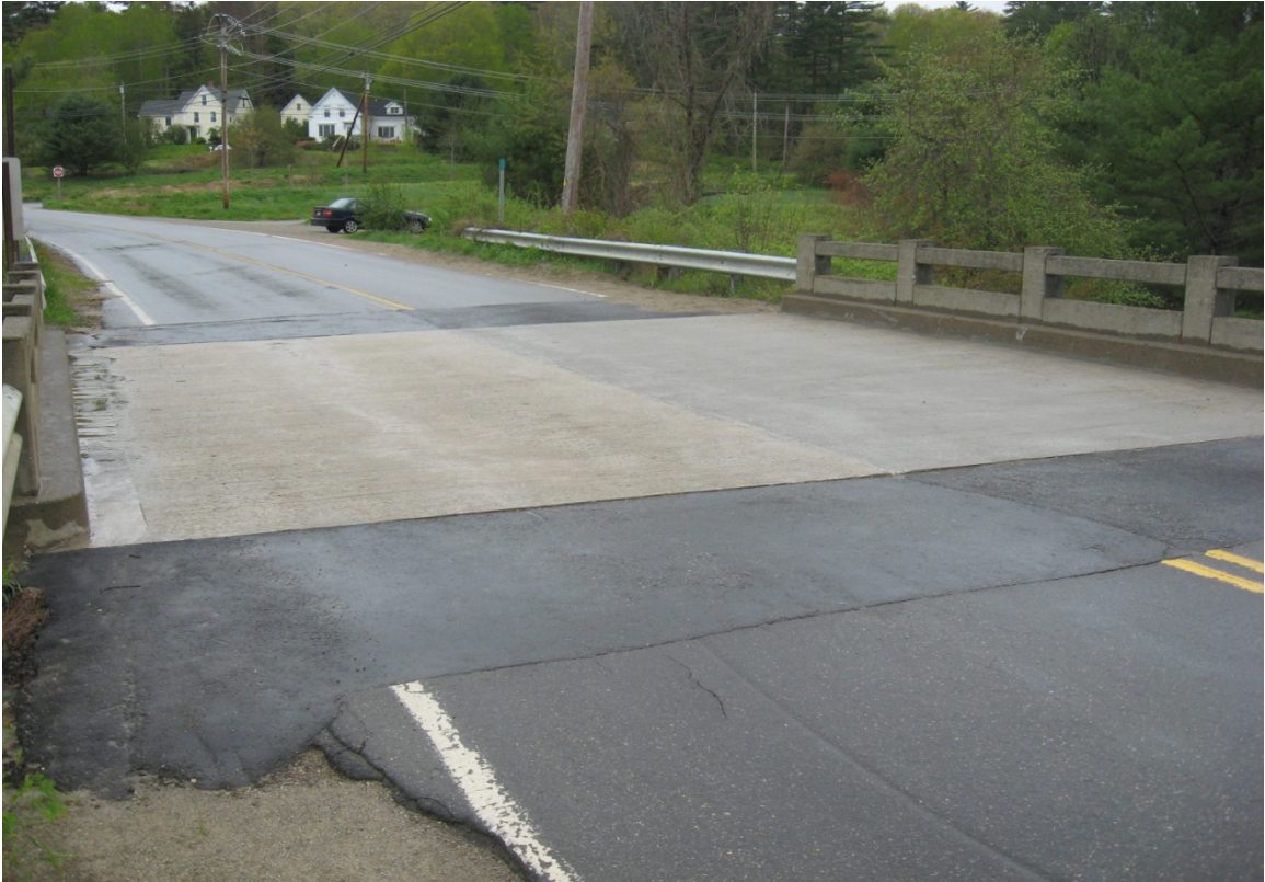
Figure 47 – Photo of Newcastle Bridge #5608 from Bridge Visit Conducted in May 2011
