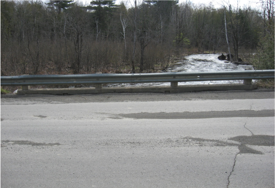
Figure 42 – Photo of Linneus Bridge #5733 from Bridge Visit Conducted in May 2011
