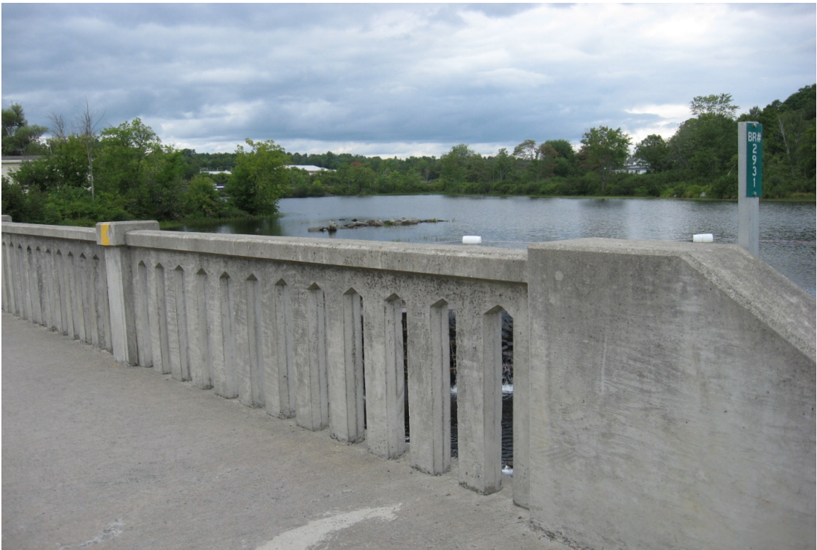
Figure 44 - Photo of Milo Bridge #2931 Top Rail from Bridge Visit Conducted August 2010
