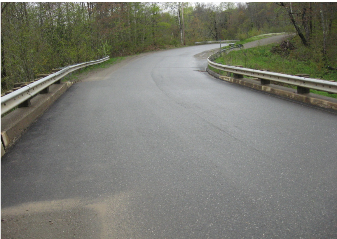
Figure 46 – Photo of Monroe Bridge #5538 from Bridge Visit Conducted in May 2011
