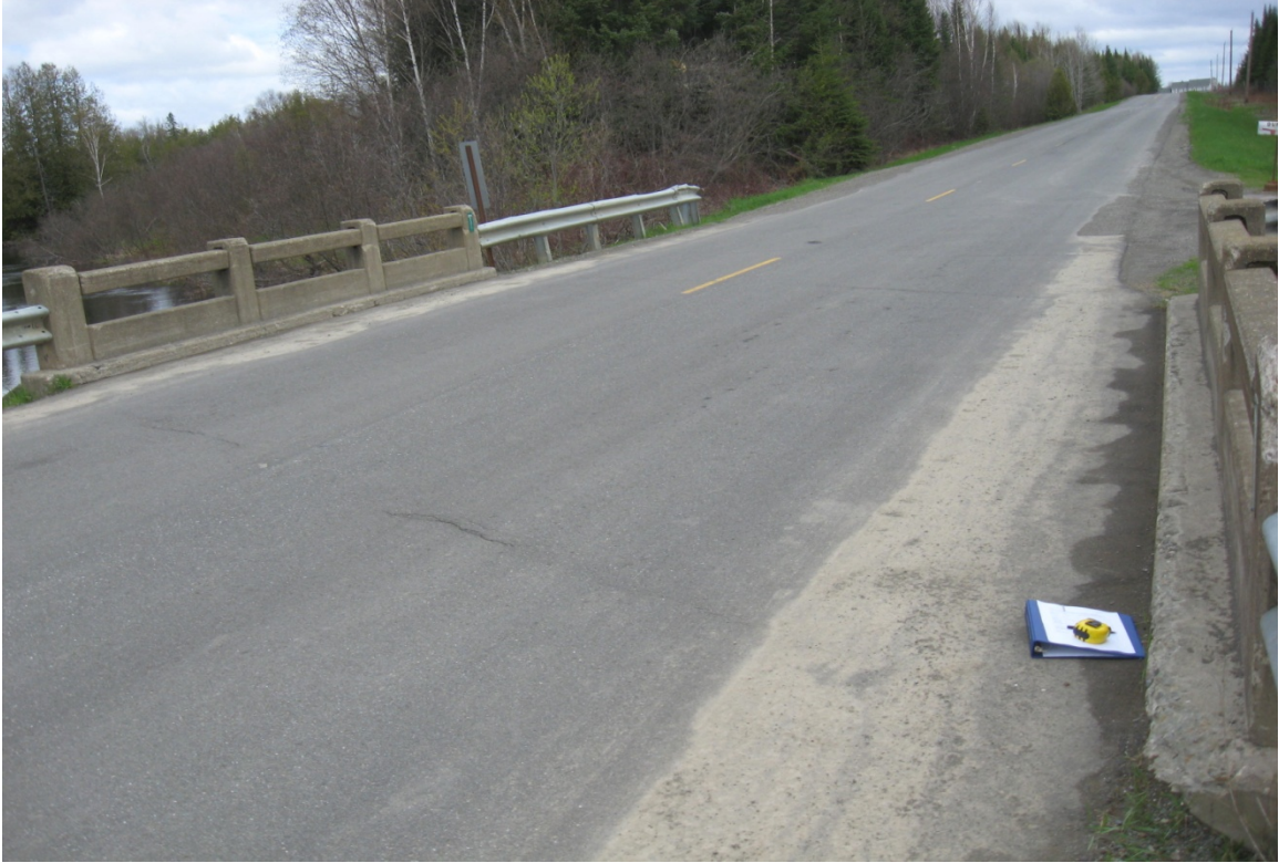
Figure 41 – Photo of Linneus Bridge #5311 from Bridge Visit Conducted in May 2011
