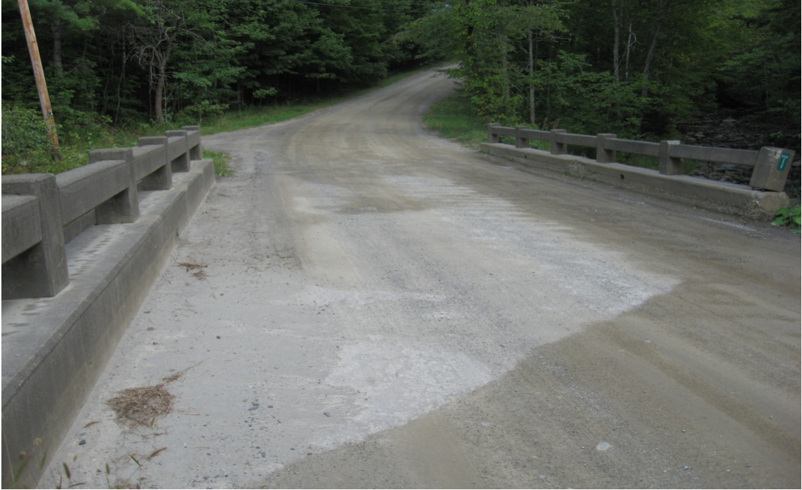
Figure 27 – Photo of Albion Bridge #2529 from Bridge Visit in August 2010.
