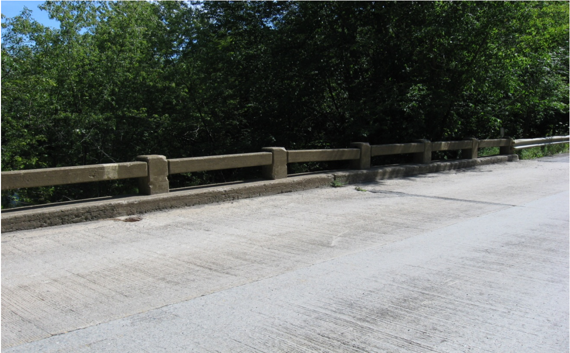
Figure 39 - Photo of Levant Bridge #5253 Rail from Bridge Visit Conducted in July 2010
