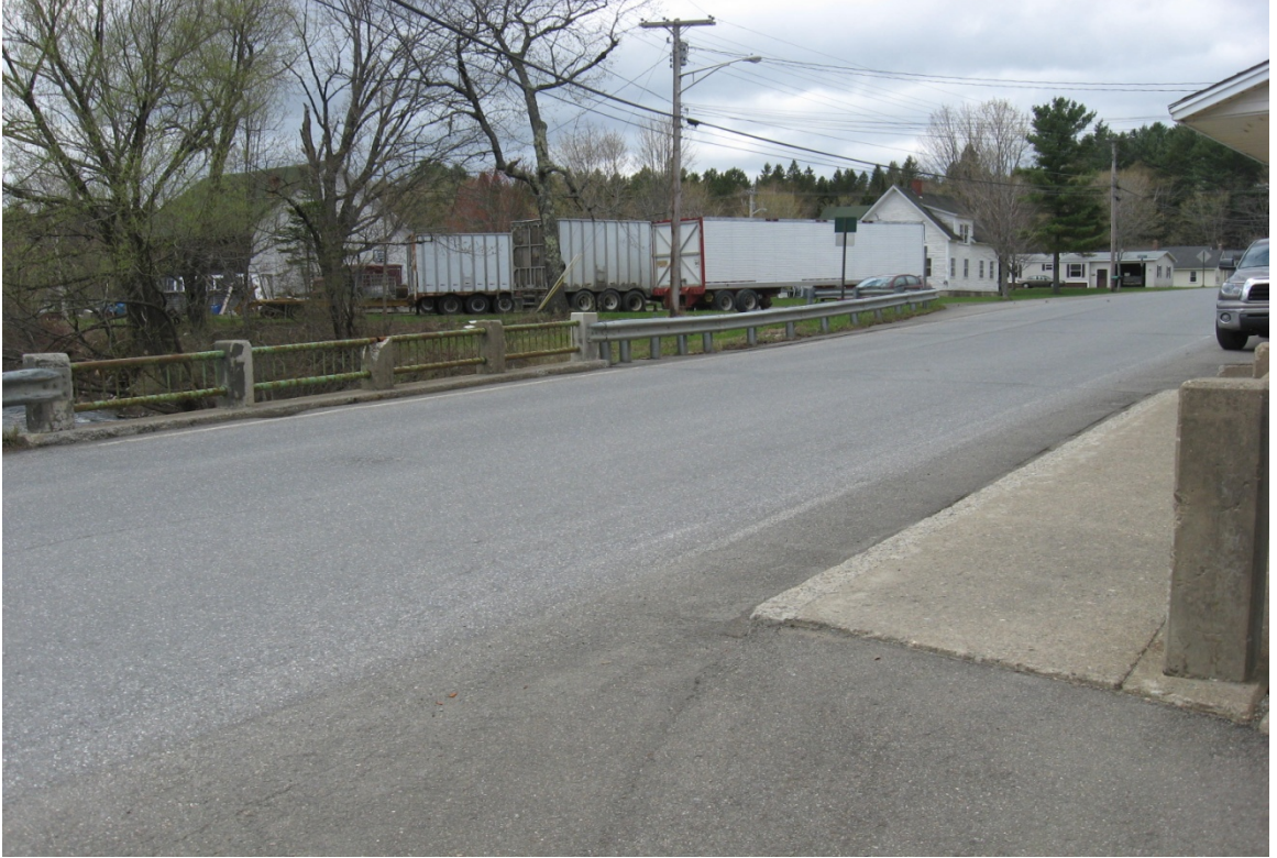
Figure 49 – Photo of Sherman Bridge #5311 from Bridge Visit Conducted in May 2011
