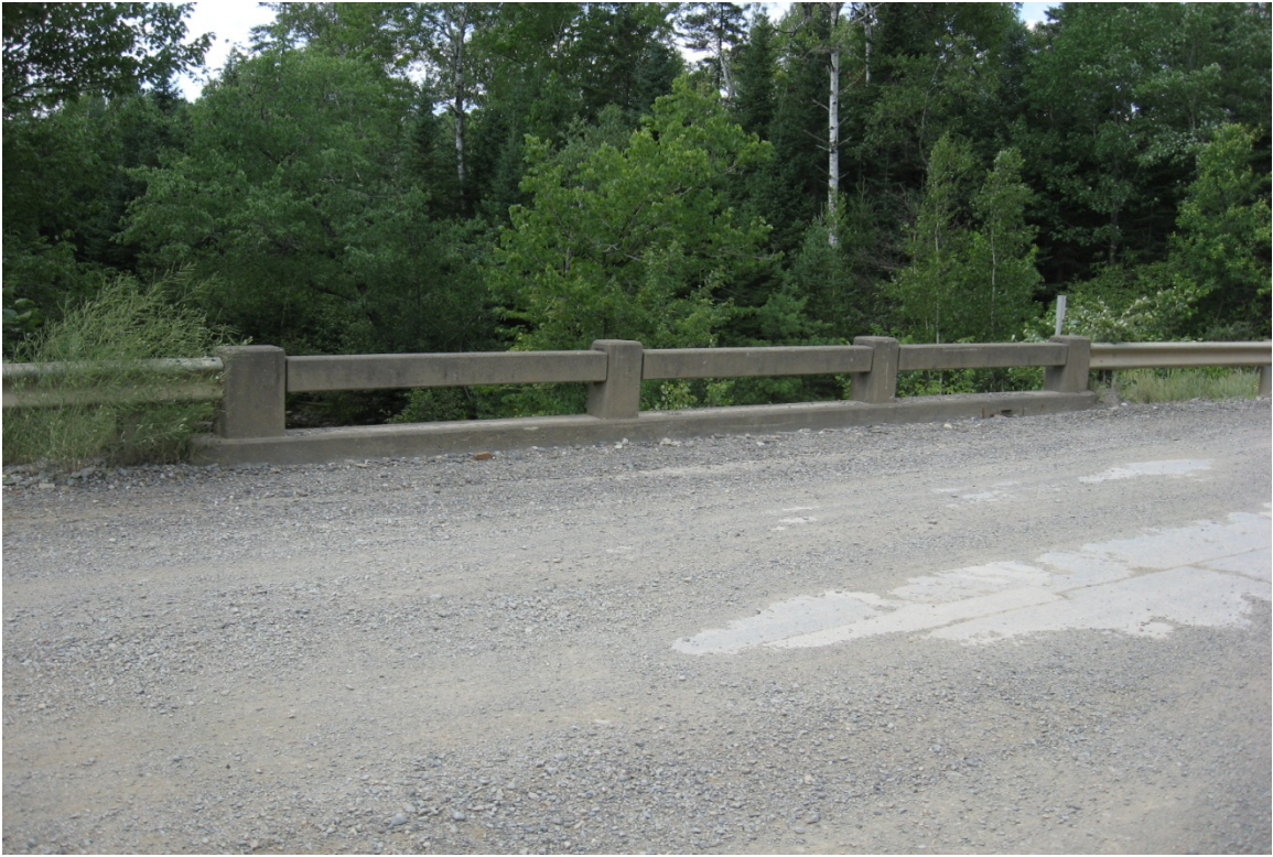
Figure 43 - Photo of Milford Bridge #2070 Rail from Bridge Visit Conducted July 2010
