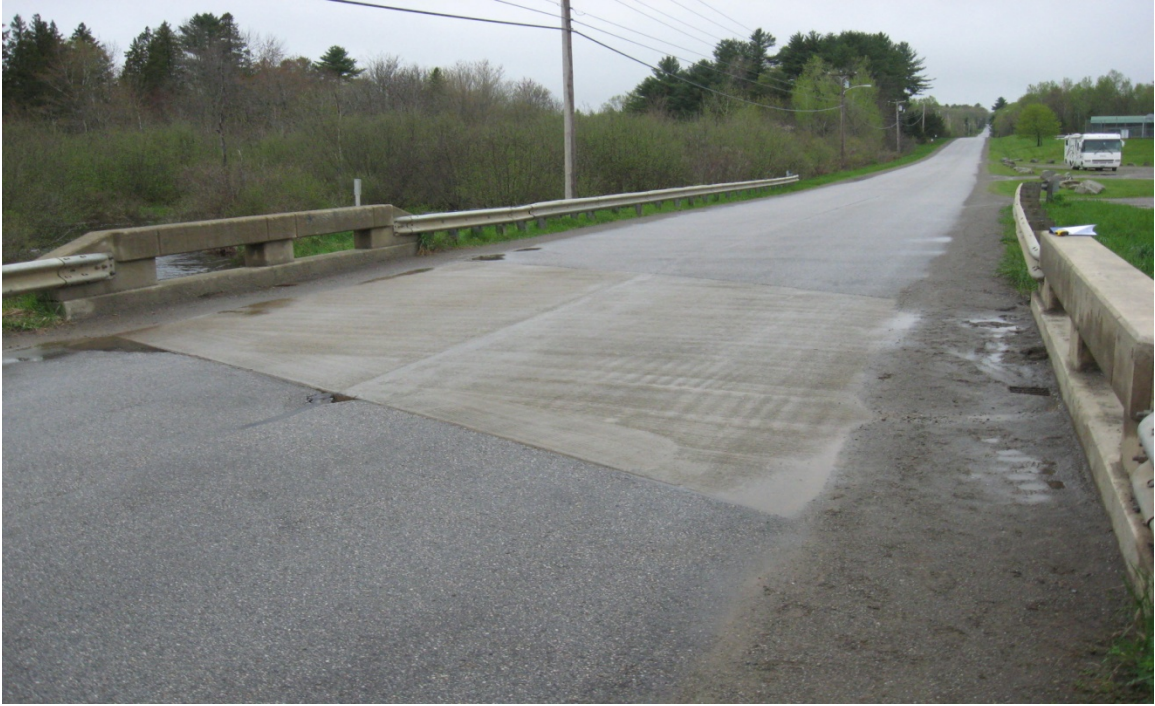
Figure 33 – Photo of Carmel Bridge #5632 from Bridge Visit Conducted in May 2011
