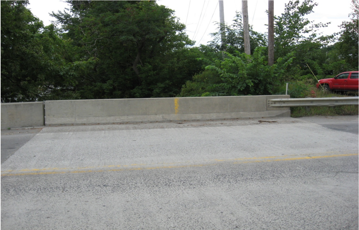
Figure 45 - Photo of Milo Bridge #2931 Bottom Rail from Bridge Visit Conducted August 2010
