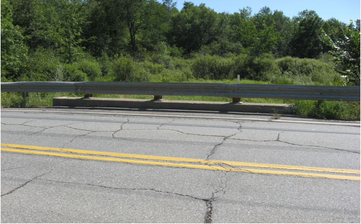
Figure 37 - Photo of Hermon Bridge Rail from bridge Visit Conducted August 2010.
