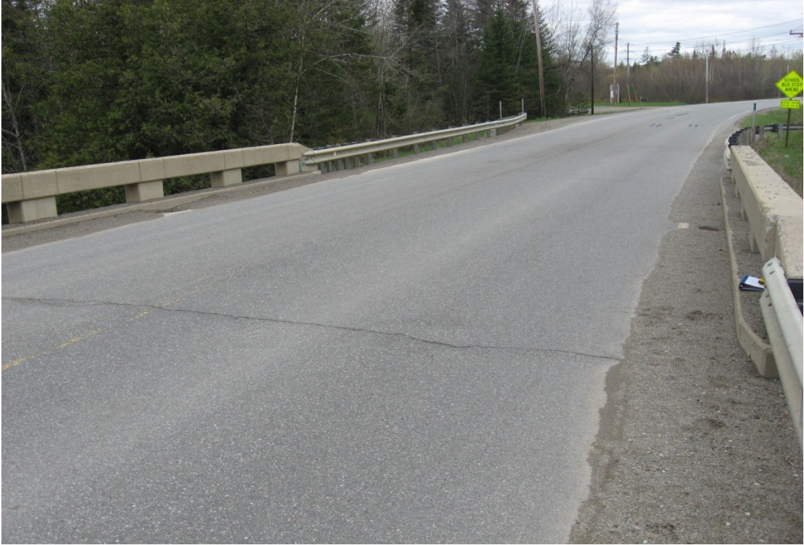
Figure 34 – Photo of Chester Bridge #5907 from Bridge Visit Conducted May 2011
