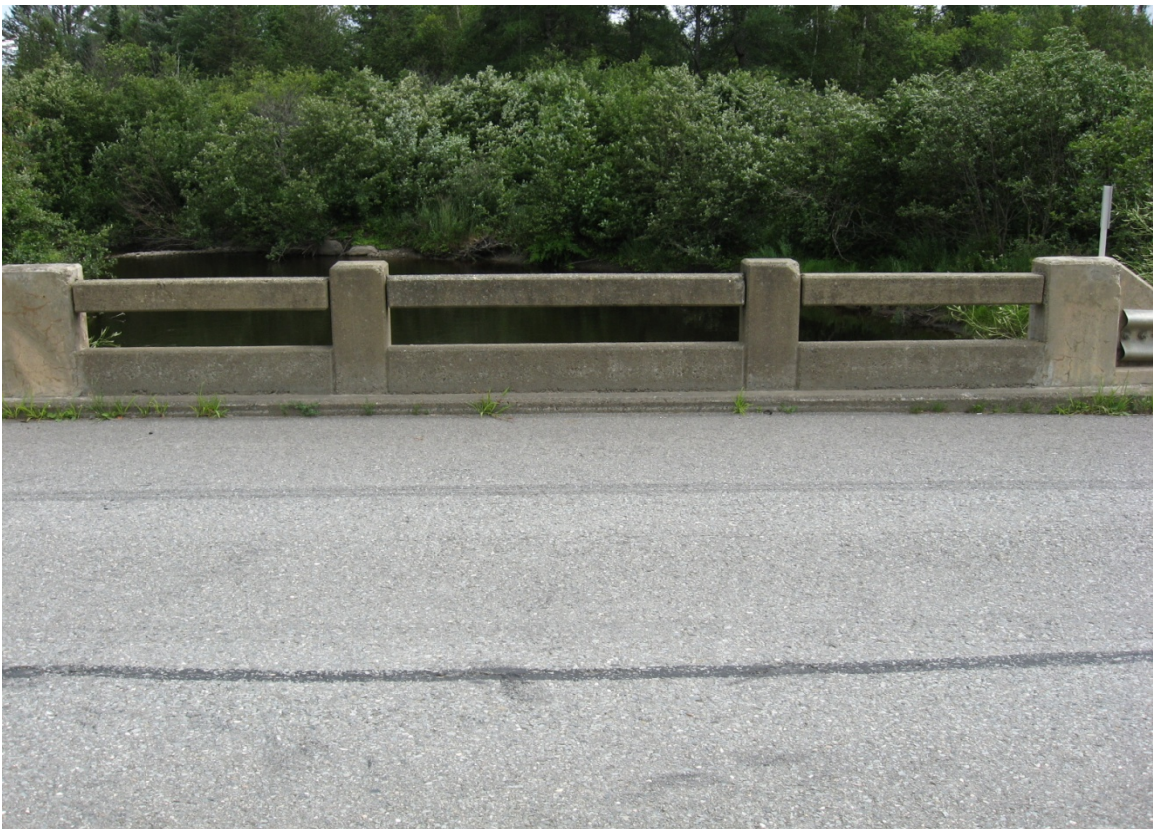
Figure 30 - Photo of Bradford Bridge #3430 Rail from Bridge Visit Conducted July 2010
