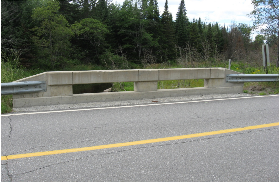
Figure 29 - Photo of Argyle Bridge #3827 Rails from Bridge Visit Conducted July 2010
