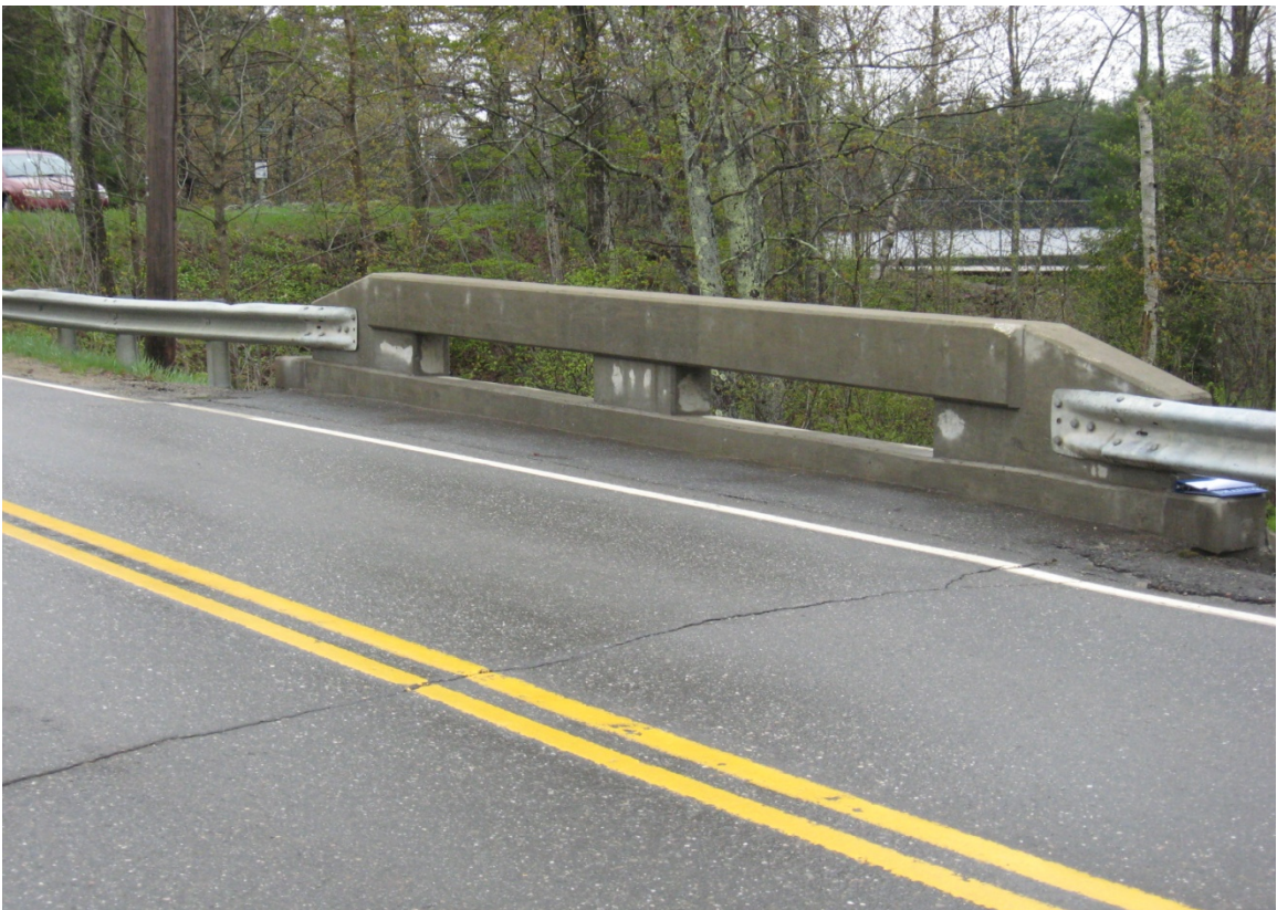
Figure 40- Photo of Liberty Bridge #3493 from Bridge Visit Conducted in May 2011
