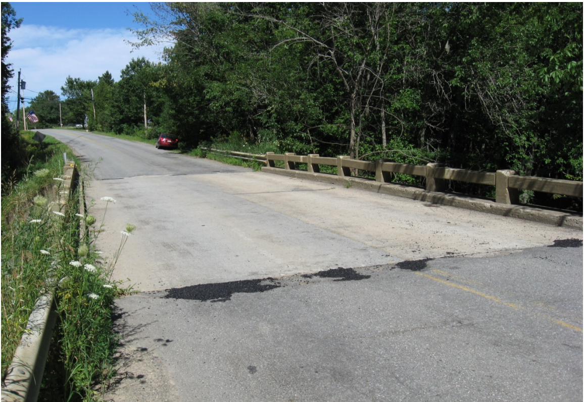
Figure 38 - Photo of Levant Bridge #5253 from Bridge Visit Conducted in July 2010
