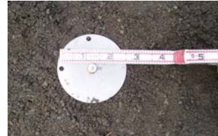
Soil Strain Gage Top Plate In Place Over Compacted Soil
