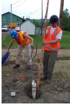
Installing Soil Thermocouple
