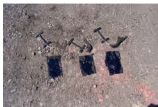
Geotextile fabric with layer of melted asphalt:
