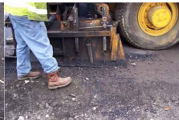
Paving over gages
