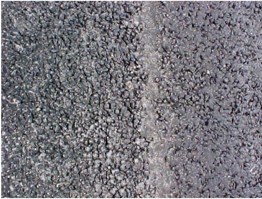
Photo 2: SMA Close-up (rolled)
