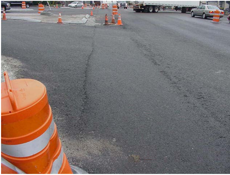
Photo 8: SMA 12.5mm Shim
