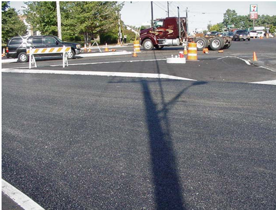
Photo 9: Finished SMA (same intersection and Fig 6 & 7)
