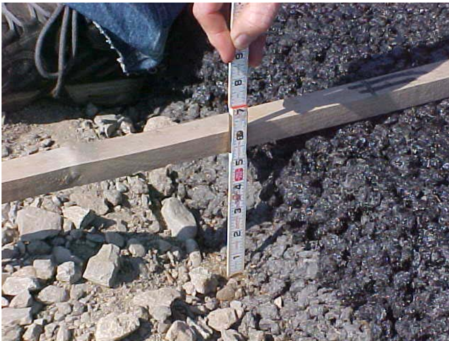
Photo 3: Depth of SMA base
