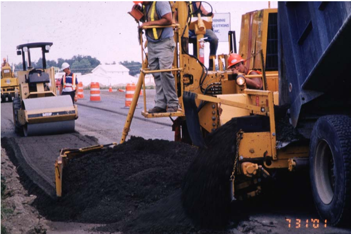
Figure 10. Final Lift of RAP Mixture
