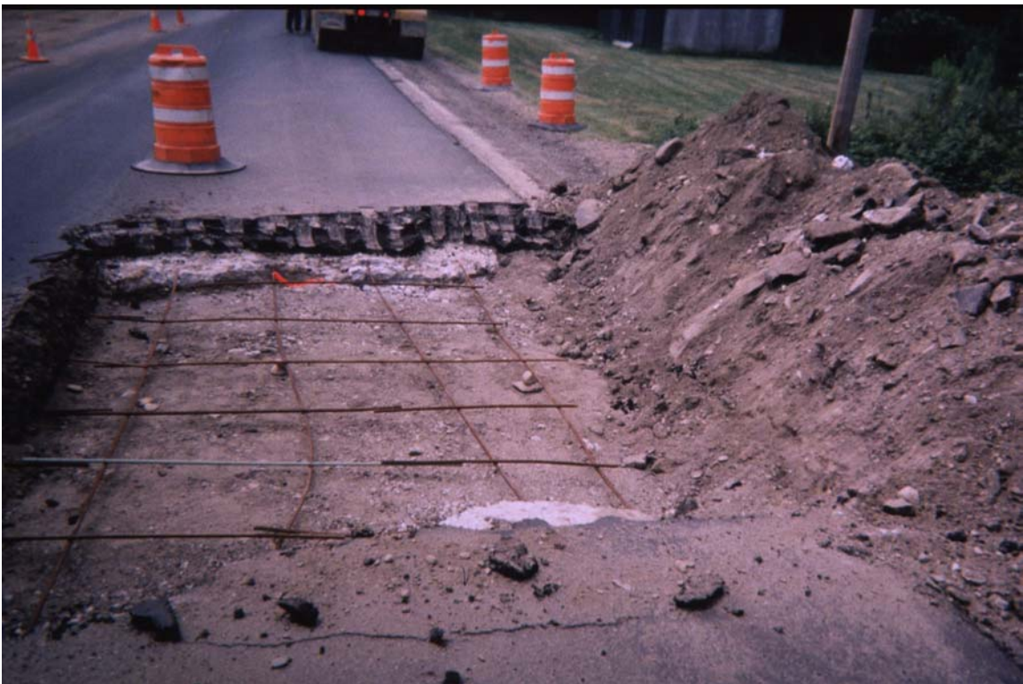
Figure 4. One of the Old Damaged Concrete Slabs Being Repaired
