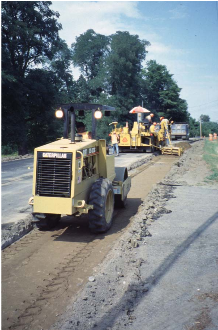
Figure 8. Preparation of Gravel Base
