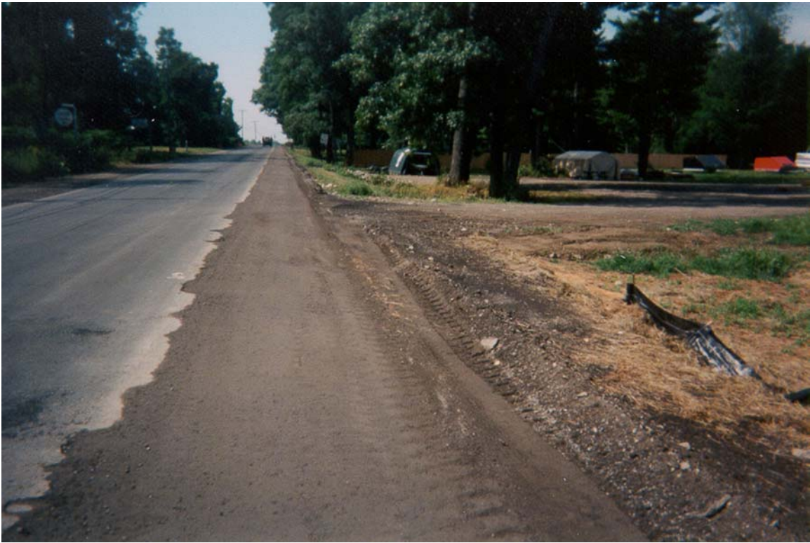
Figure 13. Shoulder Ready for Paving
