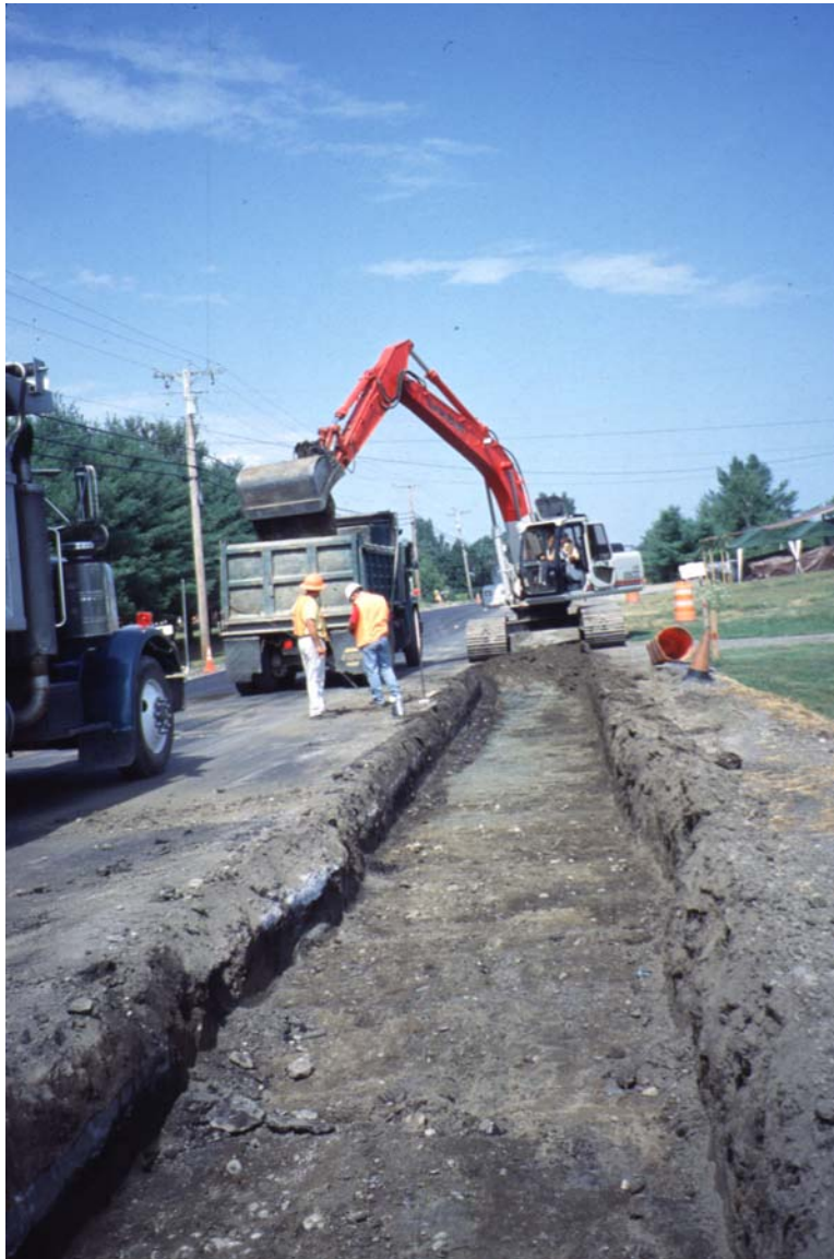
Figure 5. Excavation of Trench Adjacent to PCC Slabs
