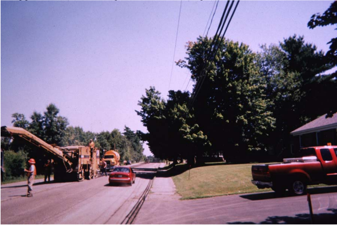
Figure 3. Initial Asphalt Grinding Operation
