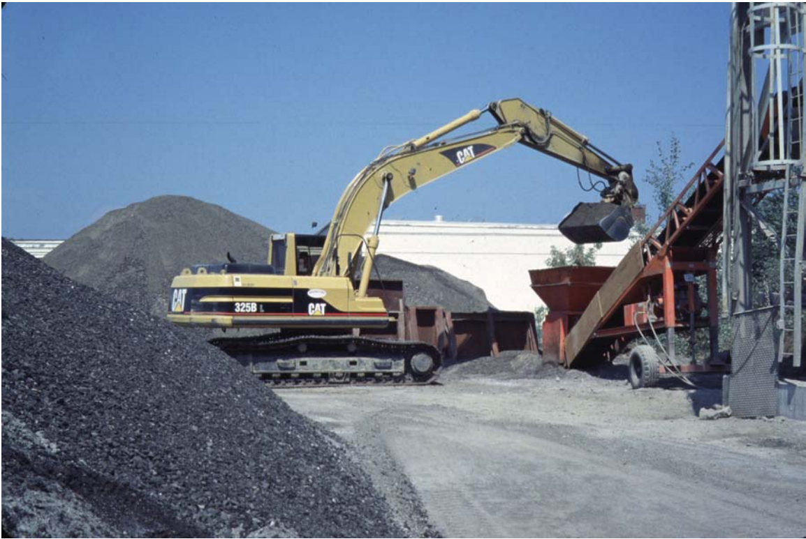
Figure 17. Preparing the Mix
