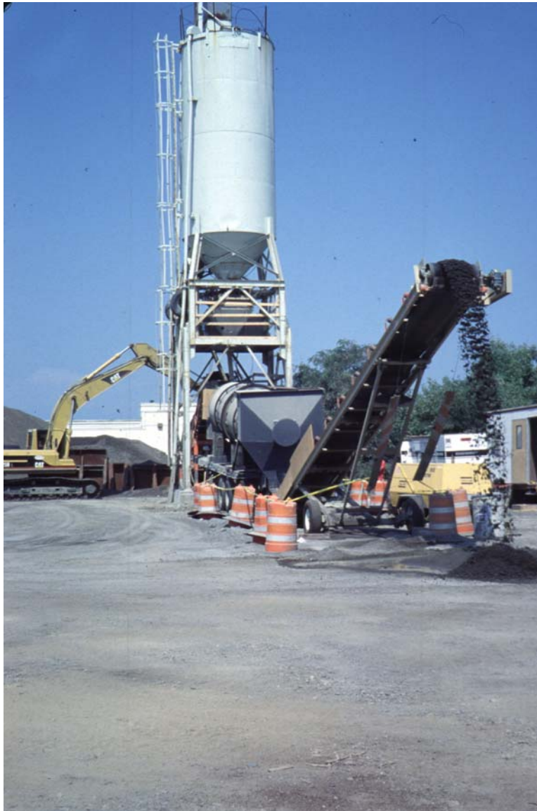
Figure 16. Customized Mixing Equipment for Preparing the RAP & PC
