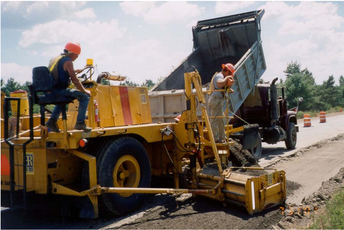
Figure 9. Placing the RAP Mixture
