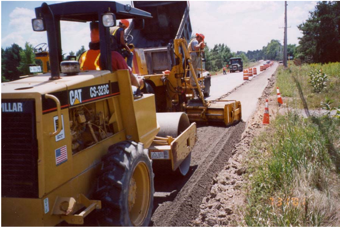
Figure 11. Rolling the Final Lift of RAP
