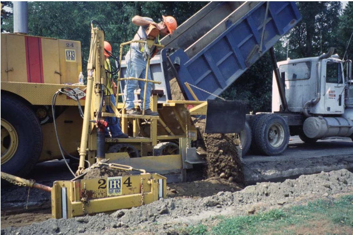
Figure 7. Shoulder Spreader Equipment Placing Gravel Base
