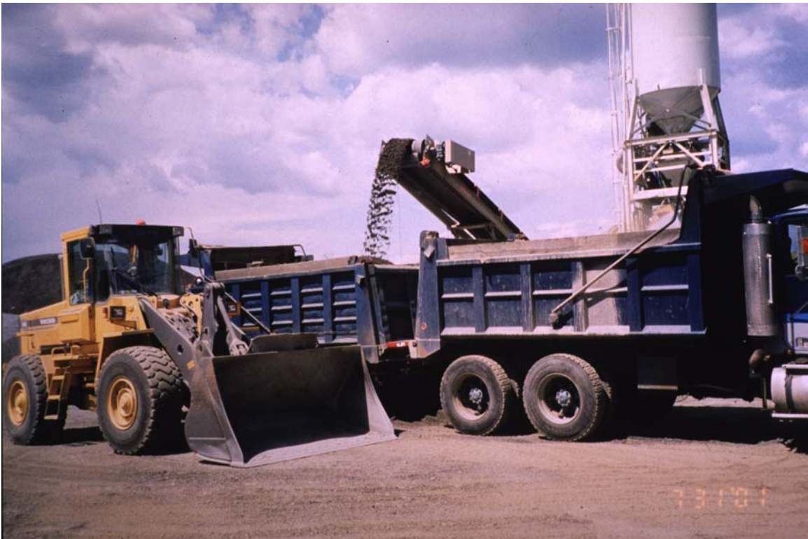
Figure 18. Mixture being Loaded into Trucks
