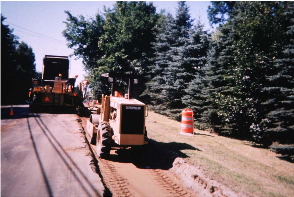
Figure 6. Placement of Gravel Base
