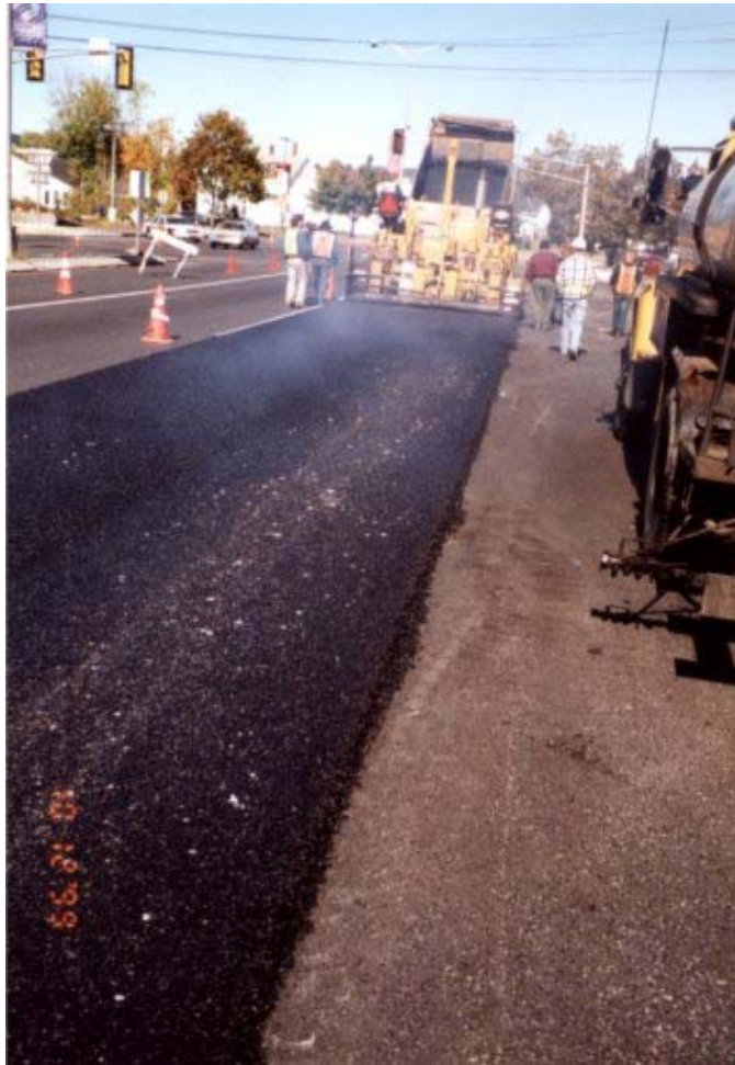
Figure 3. White Blotches Appear (Mineral Filler) in the 1 st Lift.
