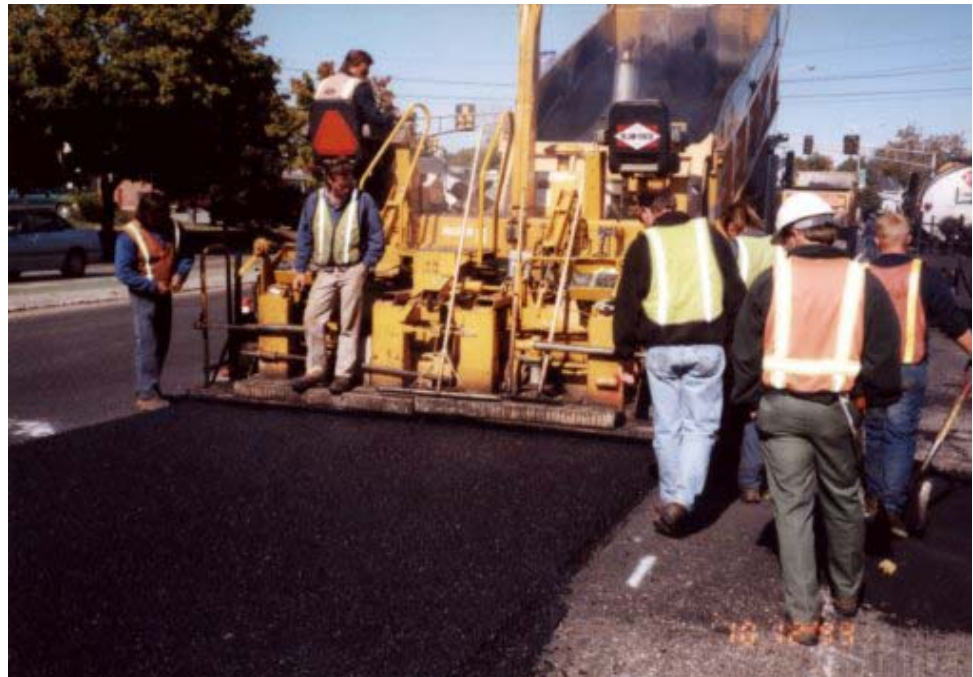
Figure 2. Paving Begins
