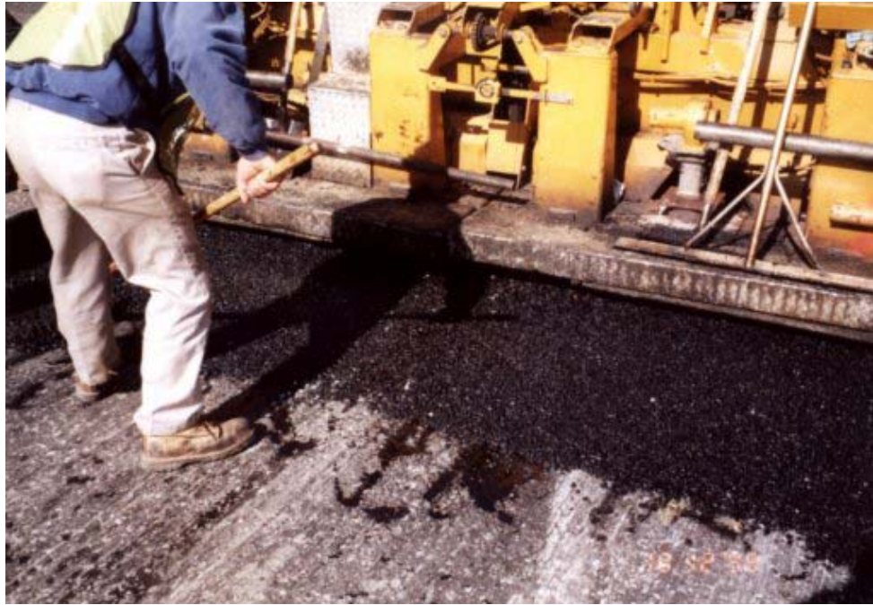
Figure 1. Constructing a Pad at beginning of SMA Section.
