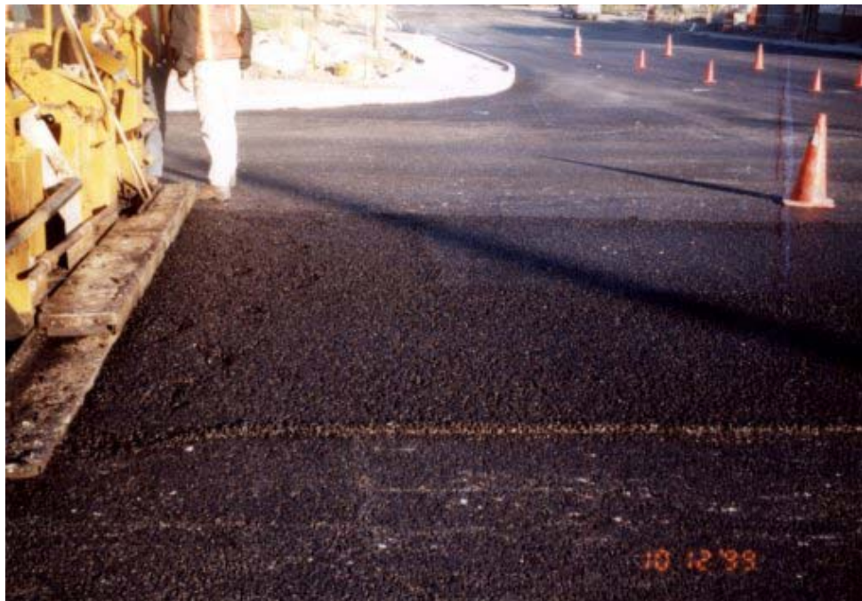
Figure 6 Second Lift of SMA.
