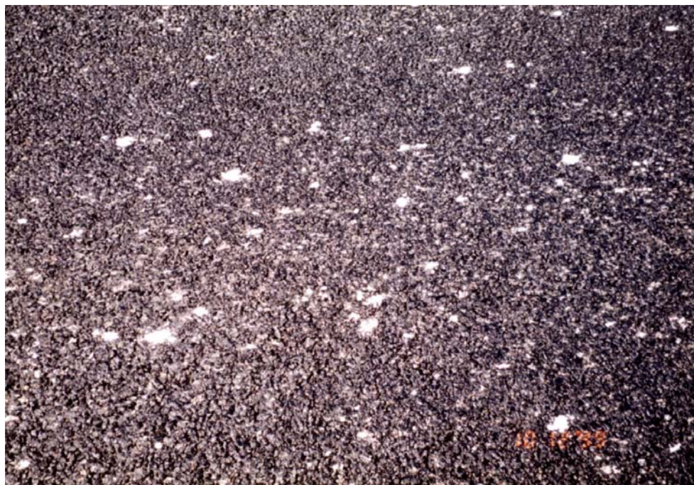
Figure 4. Close up of Blotches caused by Mineral Filler.
