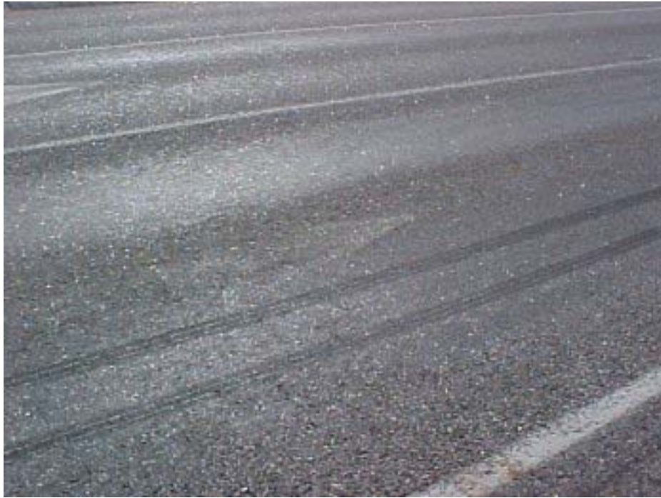
Figure 7. Wheel paths are apparent.
