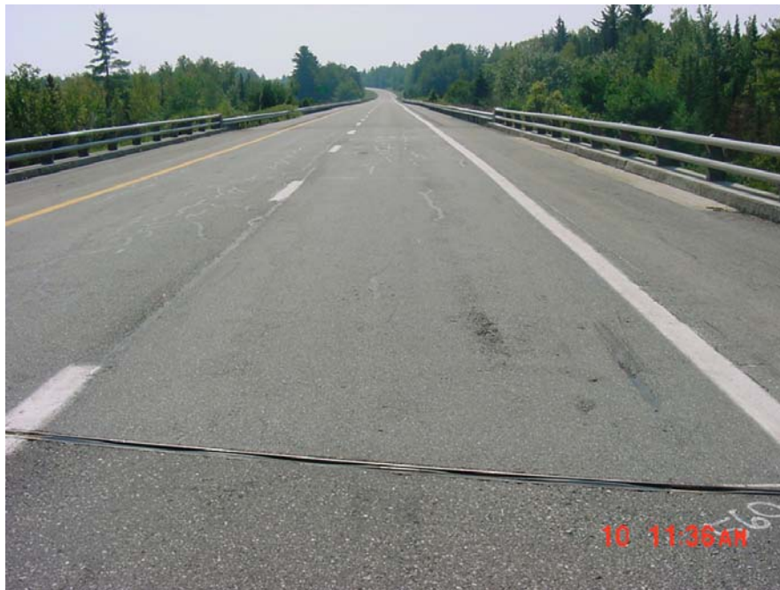
Photo 1. Bridge #6070 wearing surface
