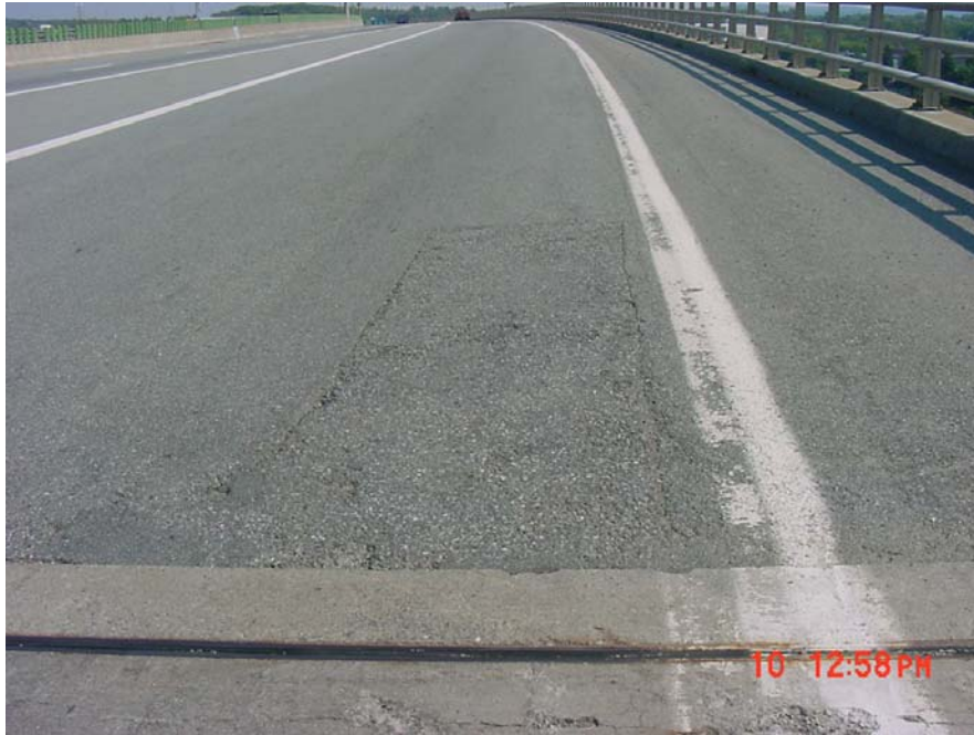
Photo 3. Bridge # 1558 patch area on entrance ramp
