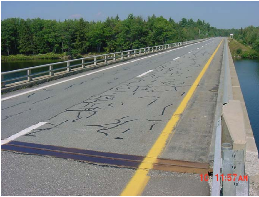
Photo 2. Bridge #6069 wearing surface
