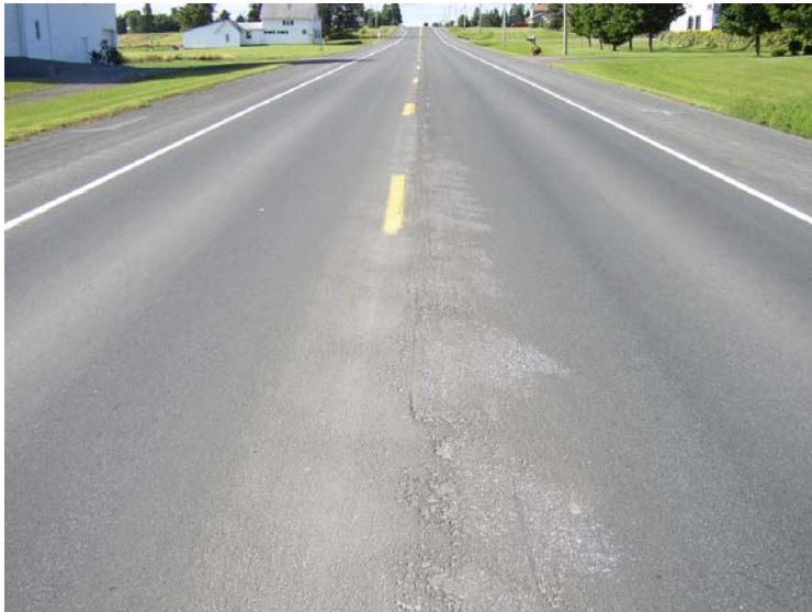
Photo 2: Section 1 Micro-Surface Centerline Plow Abrasion; August, 2004.
