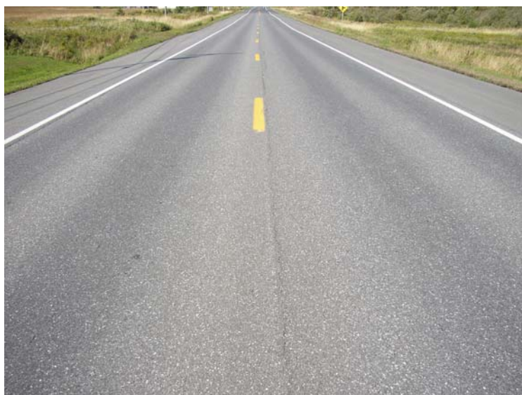
Photo 6: Section 3 Control Pavement Condition; September, 2005.
