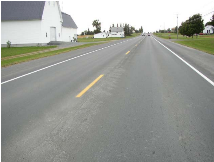
Photo 1: Section 1 Micro-Surface Centerline Plow Abrasion; September, 2003.
