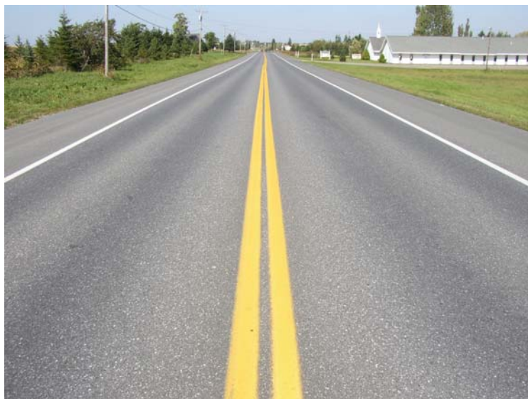
Photo 5: Section 2 Control Pavement Condition; September, 2005.
