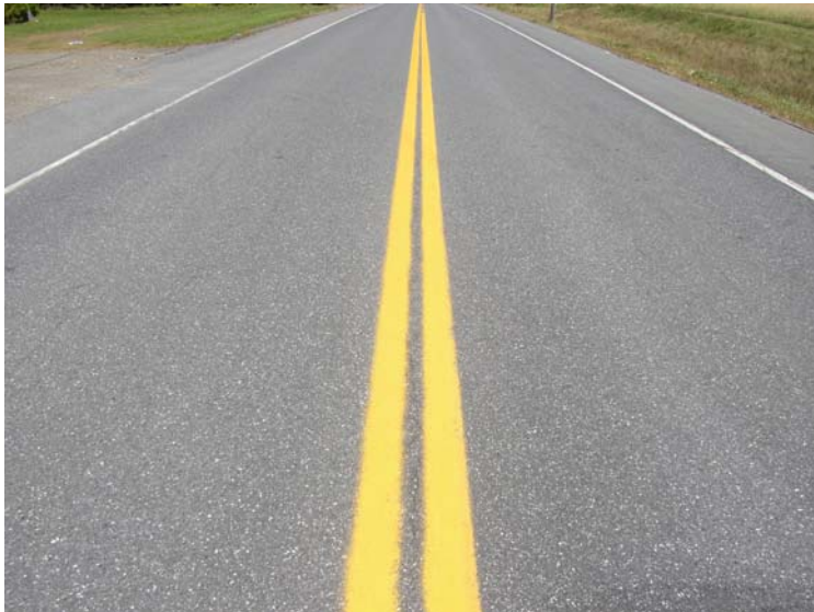
Photo 9: Section 6 Control Pavement Condition; September, 2005.
