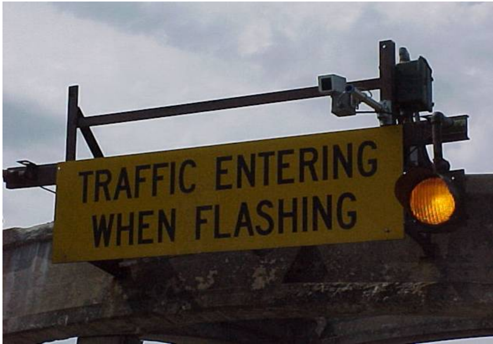
Figure 2. View of mainline warning sign.
