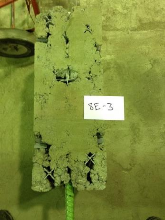
(c) Specimen with poor concrete consolidation
