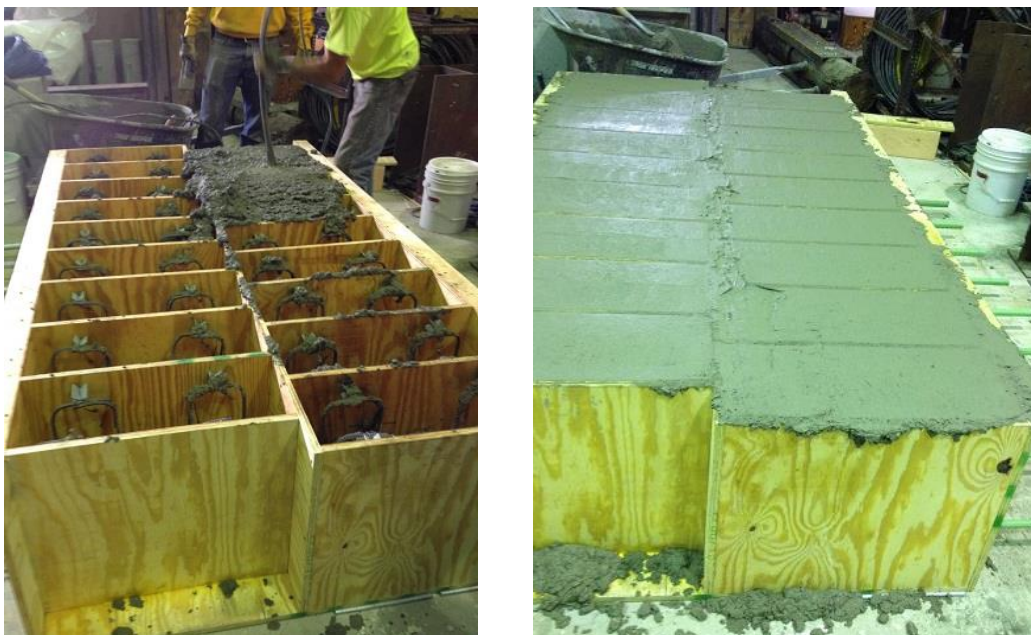
Figure 3-3. Concrete cast into the wooden forms
