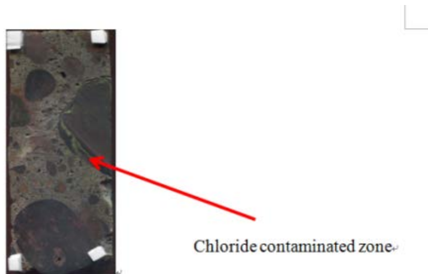
Figure 3.2: Example of chloride penetration in an ODOT concrete sample
