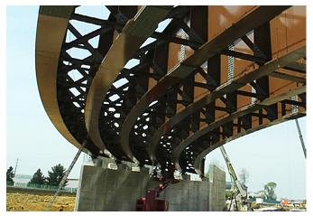
Weathering steel has a distinctive look, and with proper design considerations, makes an excellent low maintenance choice for bridge construction.
