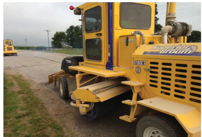
Figure 4.5 Brooms used to clear the road of debris prior to chip seal.
