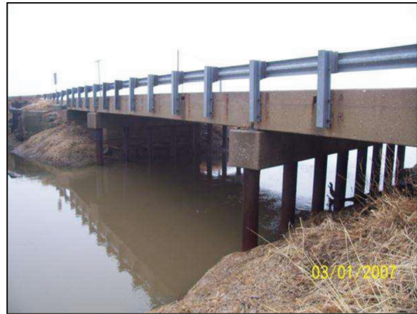
Figure 3.9 View of bridge 55-45-06258B.
