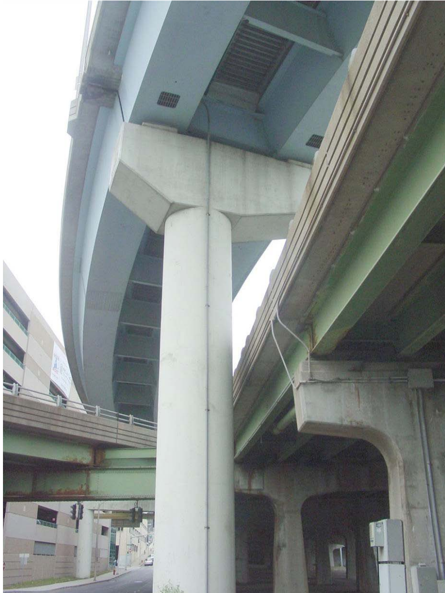
Figure 2. Column Support at Start of Segment Monitored
